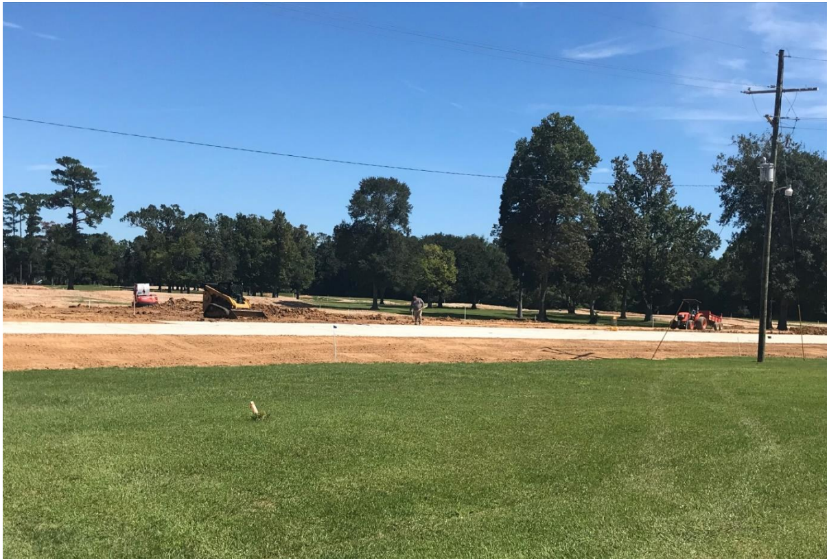
New parking path for driving range
