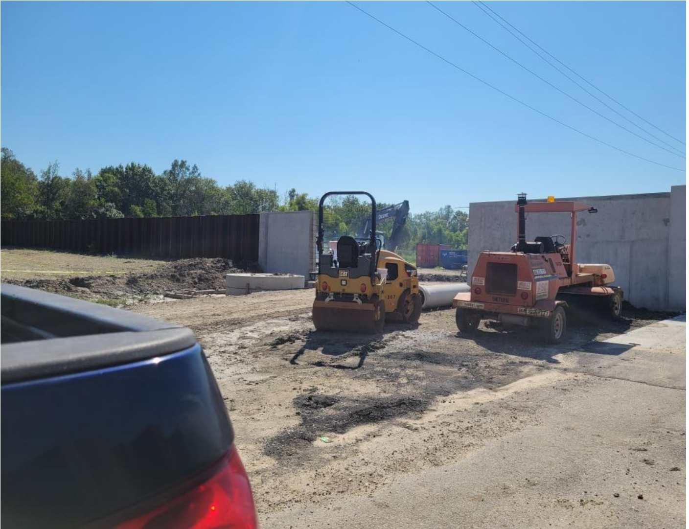
SHEET PILING ALONG THE FRONT OF THE WW TREATMENT PLANT. FLOOD INSTALLED
