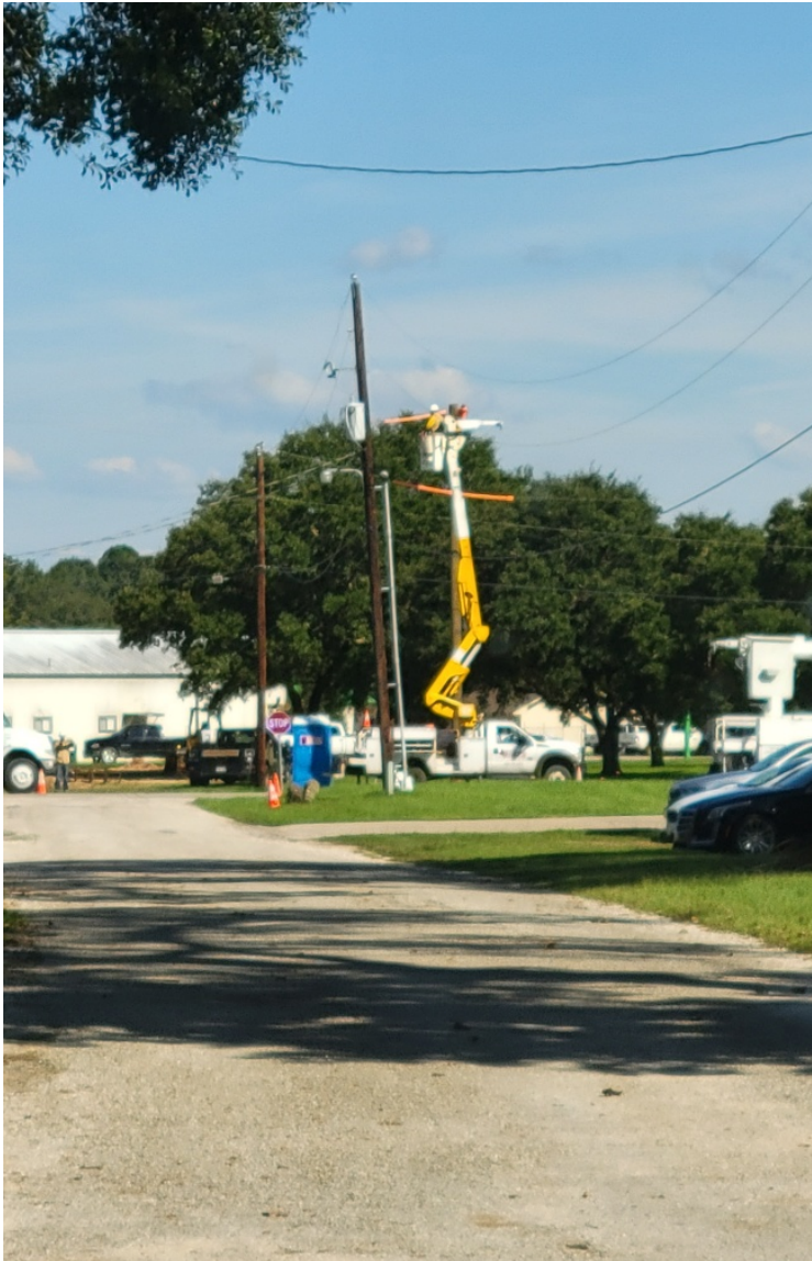
Texas Elite upgrading service on Chrysler St.
