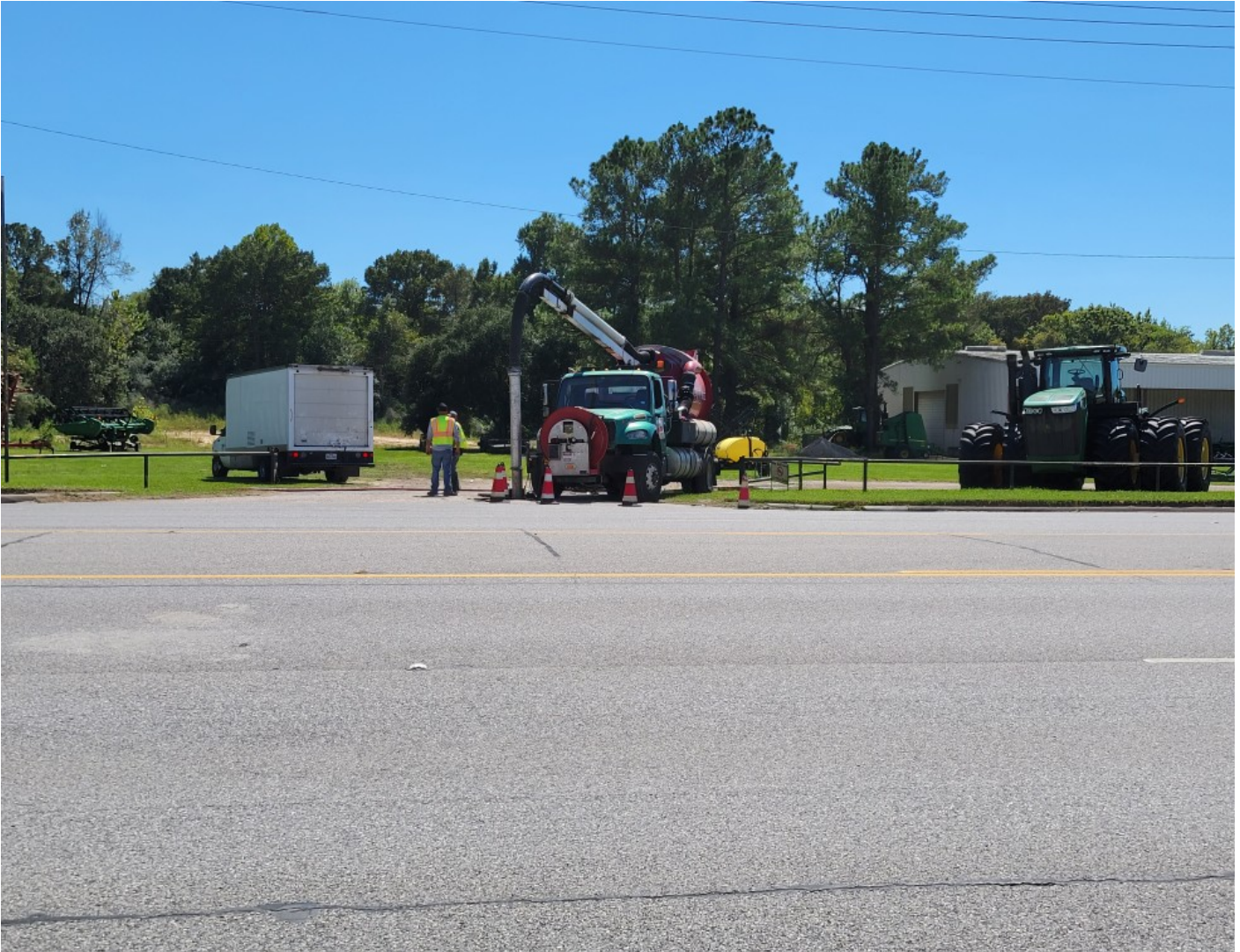
INSTALLATION OF CIPP (CURED IN-PLACE PIPE) FOR MLK TO US 90
