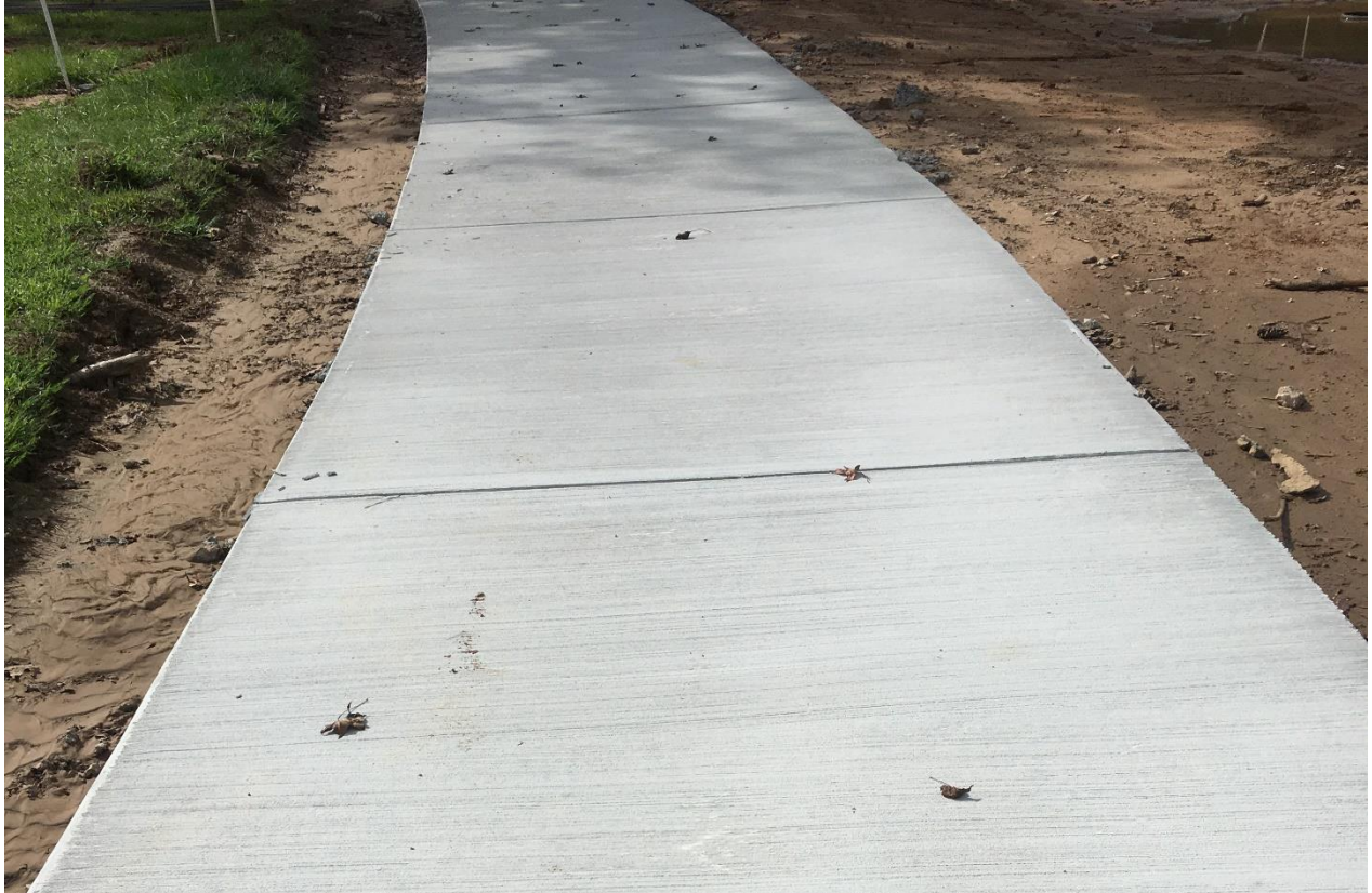
Concrete Cart Path - #1 Green
