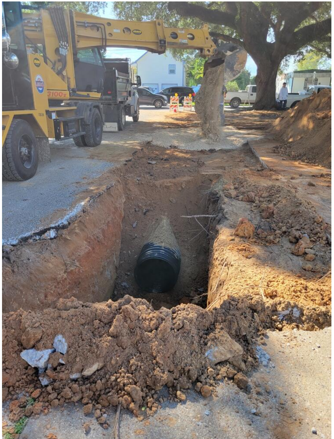
Heights St. storm drainage installation
