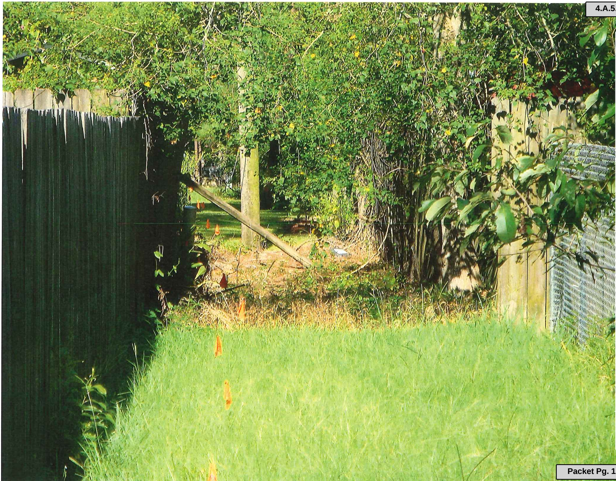
Attachment: 4th & Jessica Pics (3904 : Sewer Line Repairs)
