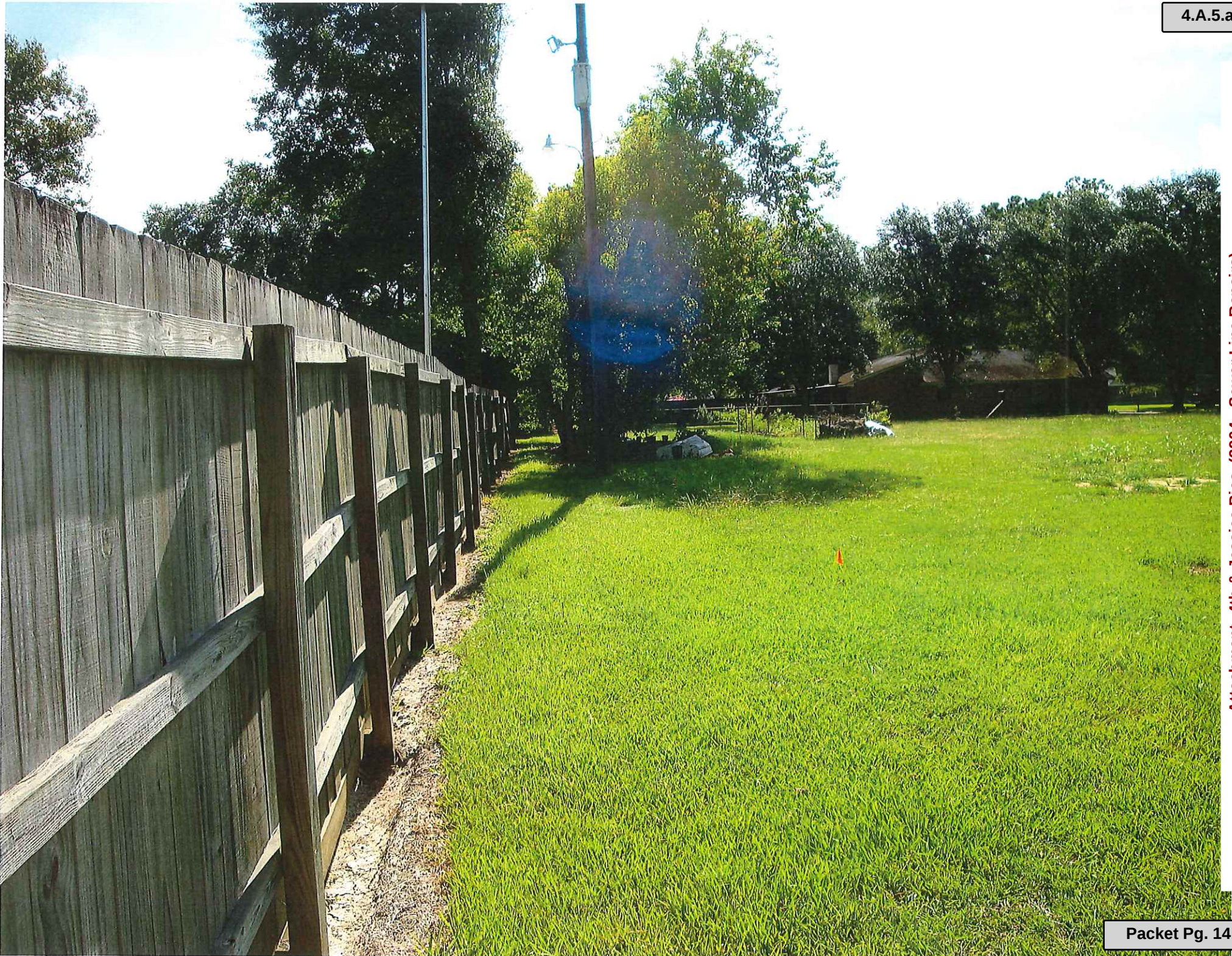
Attachment: 4th & Jessica Pics (3904 : Sewer Line Repairs)
