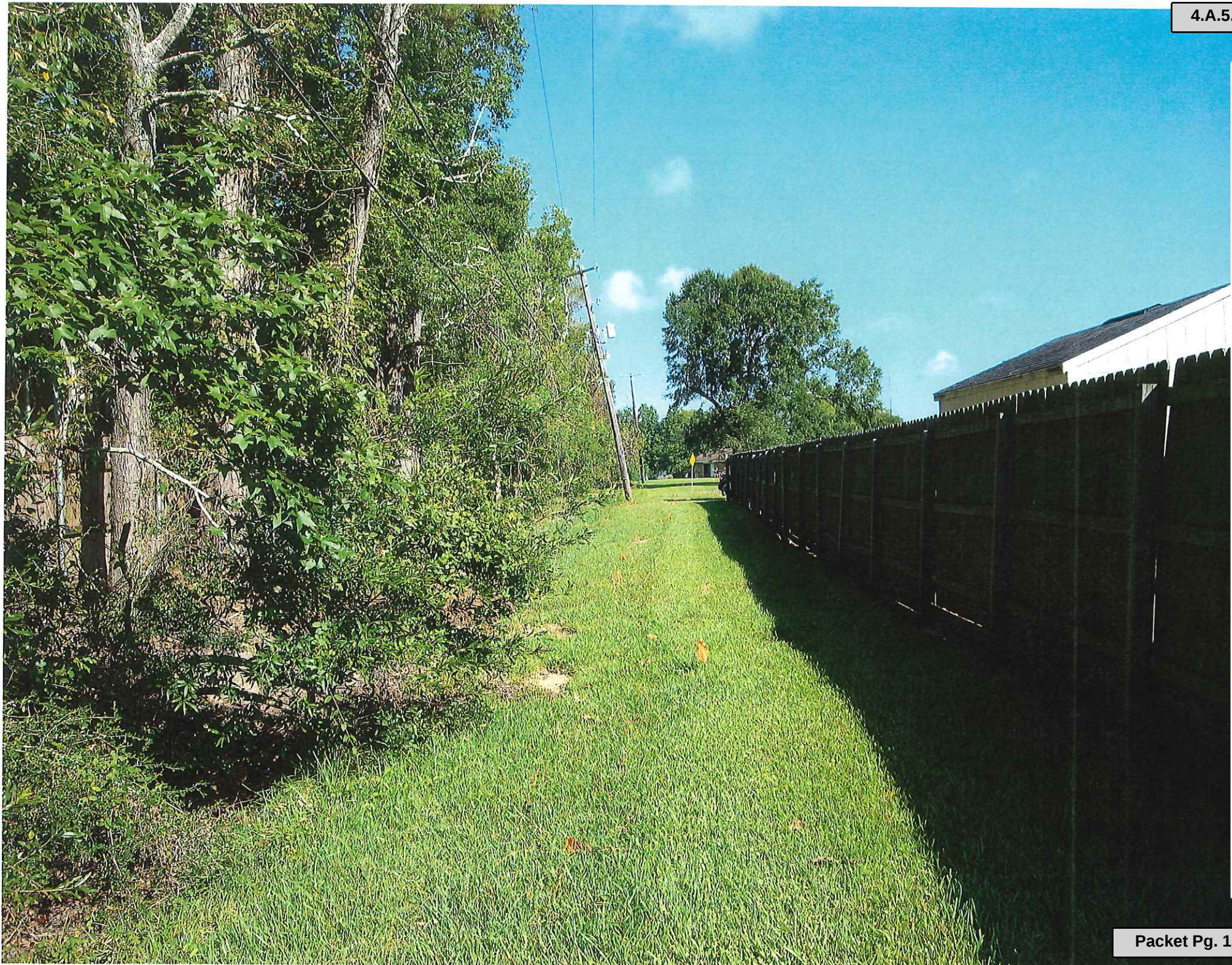
Attachment: 4th & Jessica Pics (3904 : Sewer Line Repairs)
