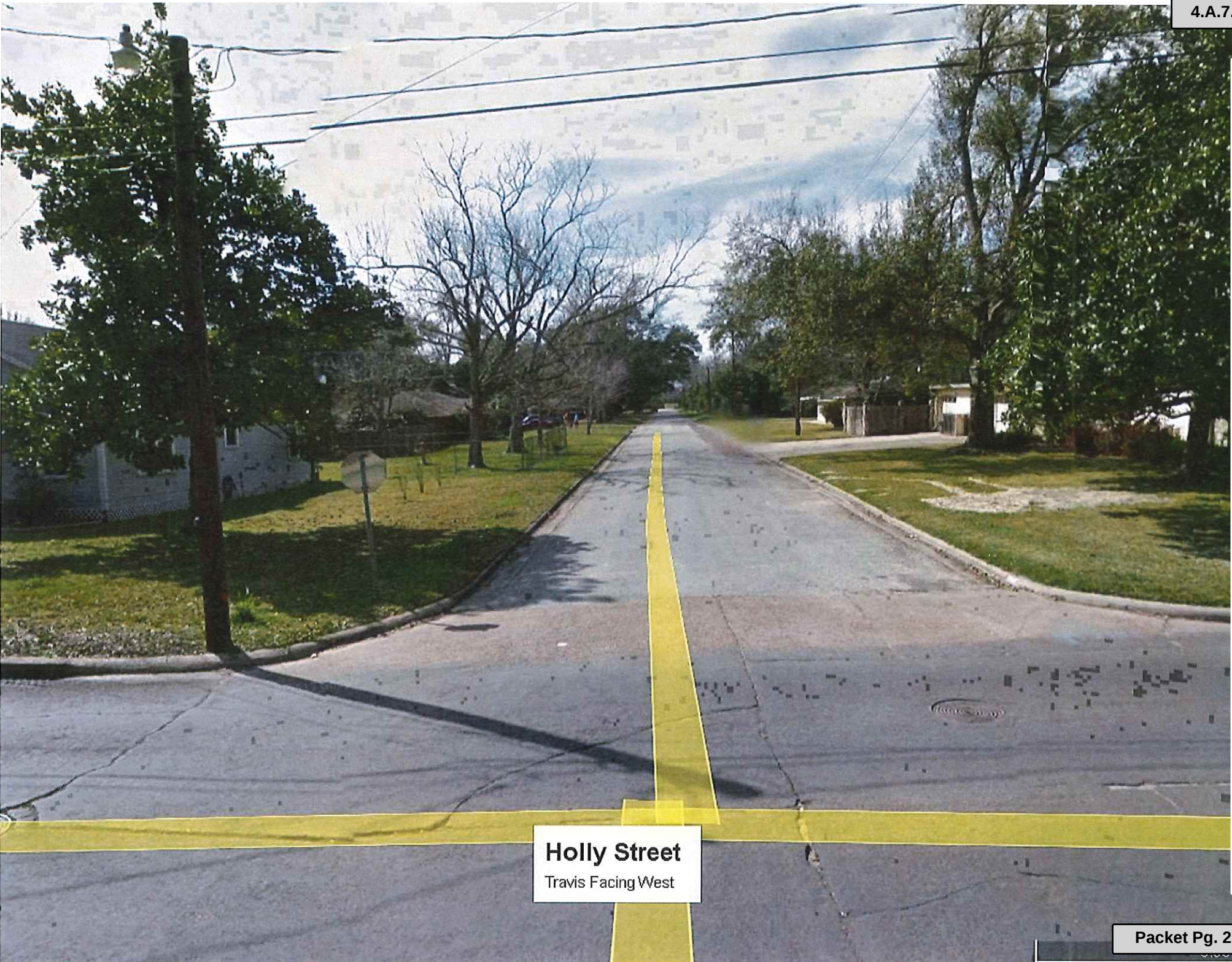
Attachment: Holly Street Pics (3906 : Drainage-Holly Street)
