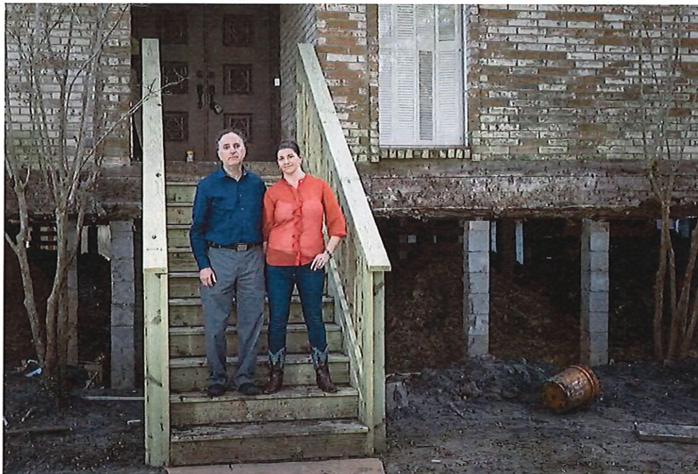
Dave Schwartz and Marni Axelrad at their home in Houston on Feb. 23, 2018. The house is being repaired and elevated due to significant damage from Hurricane Harvey, but Schwartz and Axelrad hope to move back in sometime in March. © Loren Elliott for The Texas Tribune
