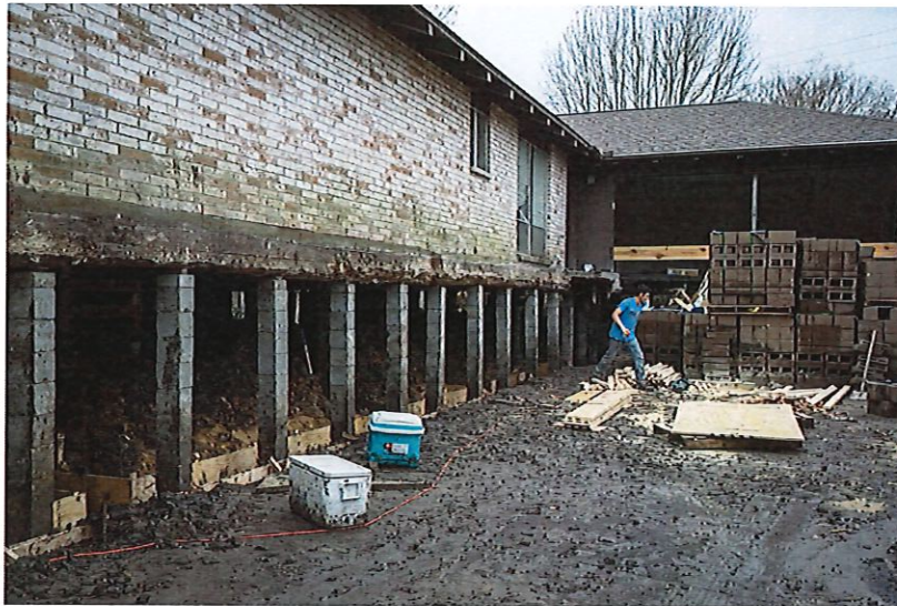
The Houston home of Marni Axelrad and her family being elevated and repaired on Feb. 21, 2018, after sustaining flood damage during Hurricane Harvey. Loren Elliott for The Texas Tribune
