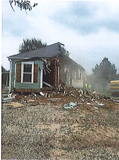
Randa Langerud's Wharton home being demolished due to damage sustained from Hurricane Harvey. Langerud's home was the first of 10 to be torn down in her neighborhood. Randa Langerud
