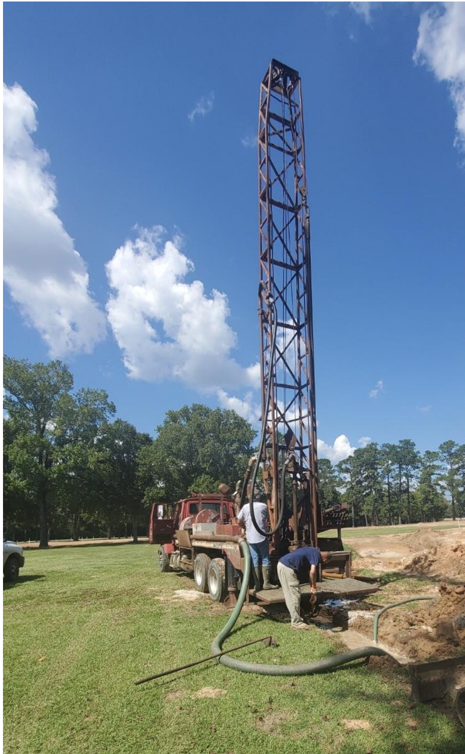
Contractor drilling test hole for new water well
