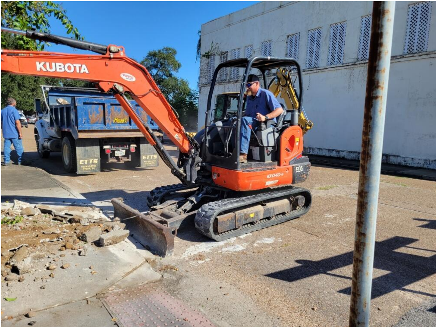
Water line repair at Main St and Trinity St: David Allison
