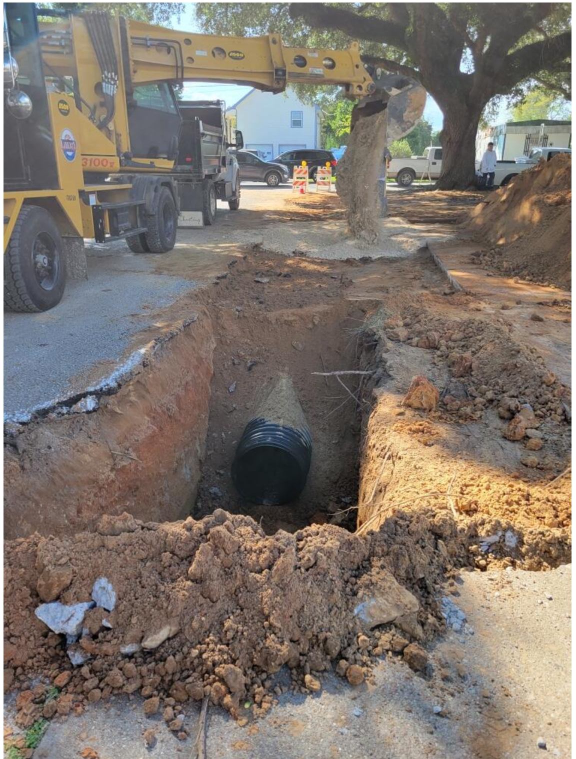
Heights St. storm drainage installation
