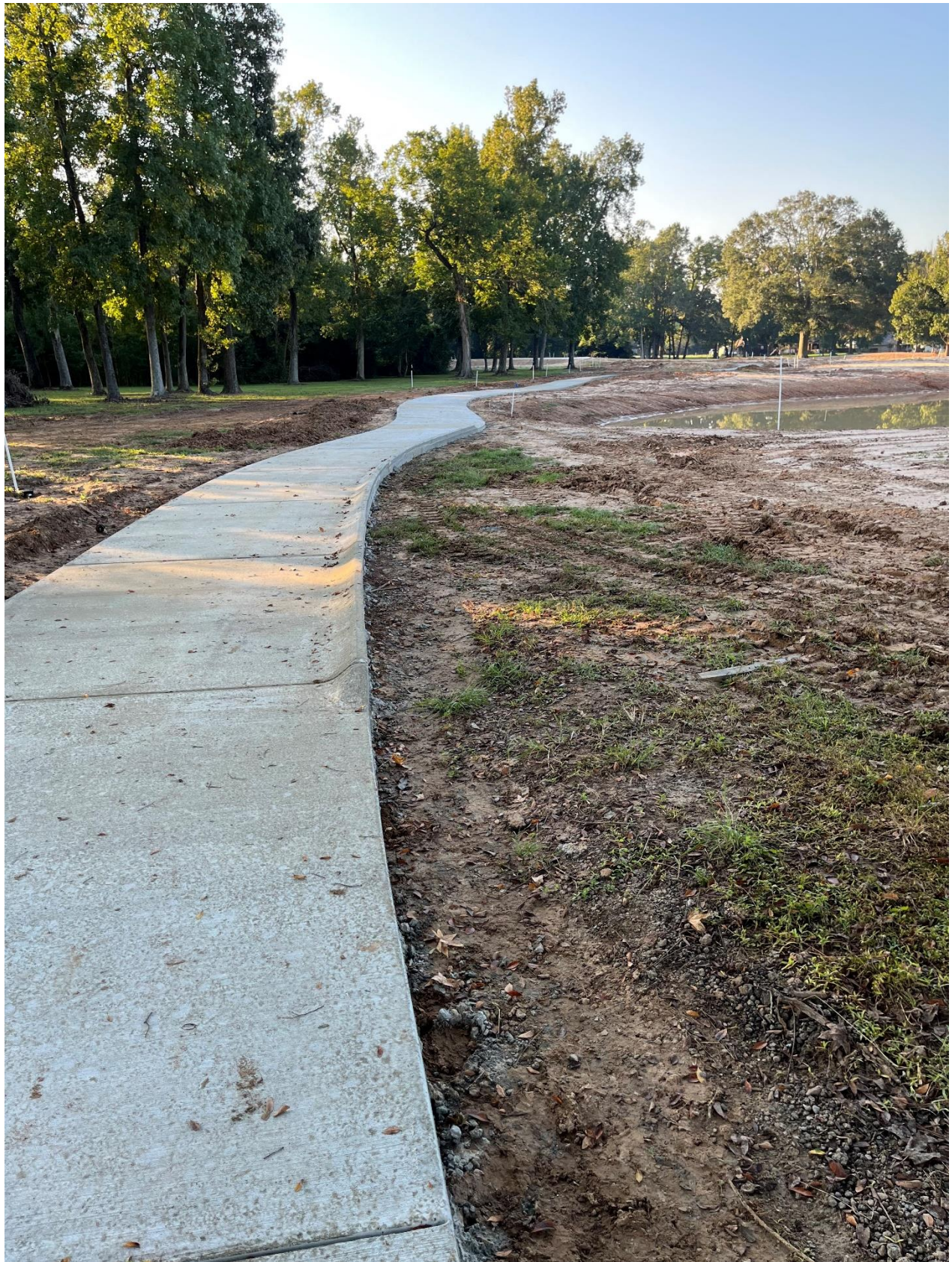
Concrete cart paths - #3 green (looking back toward tee)
