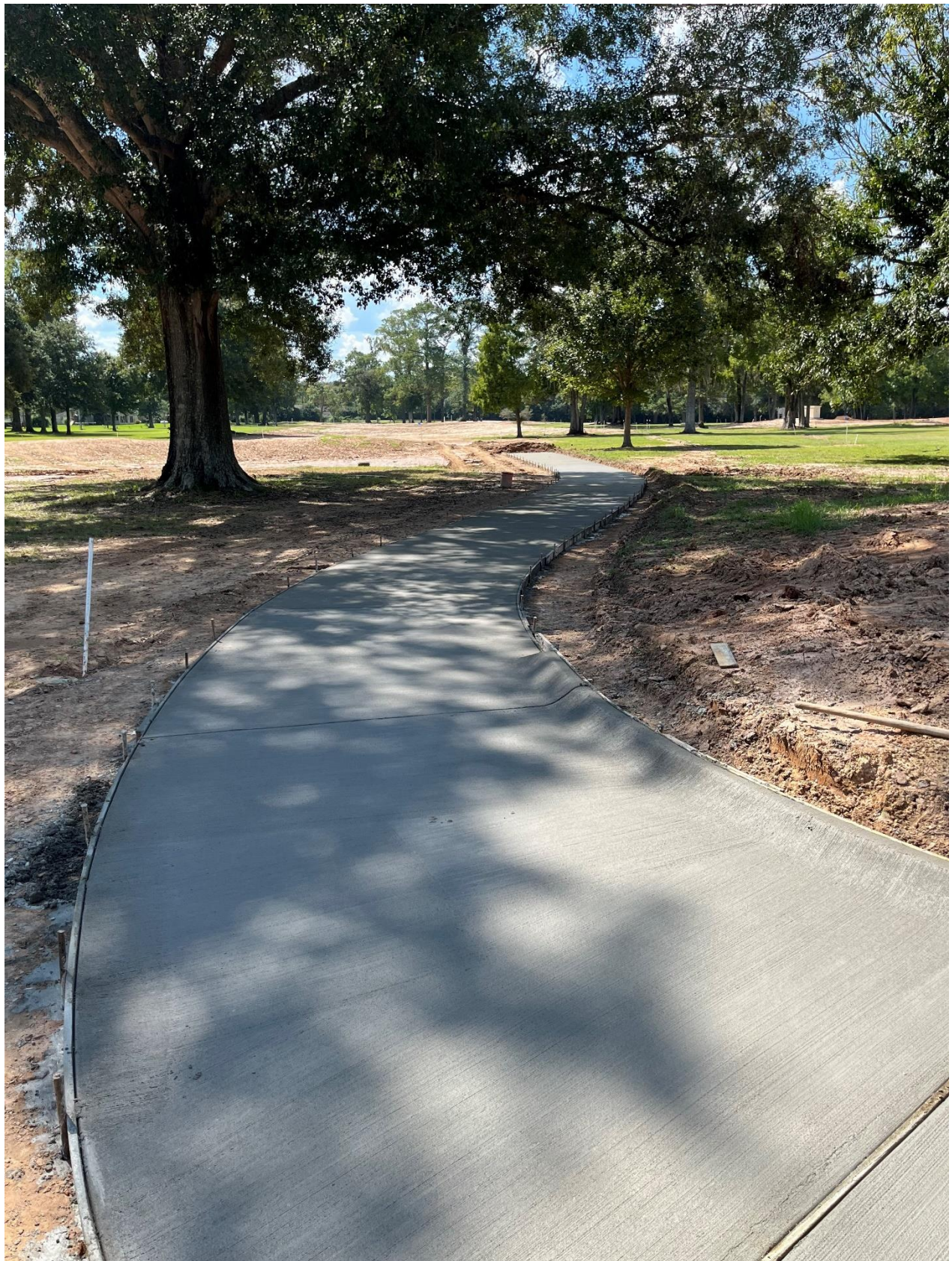
Concrete cart paths - #2 green (looking back toward fairway)
