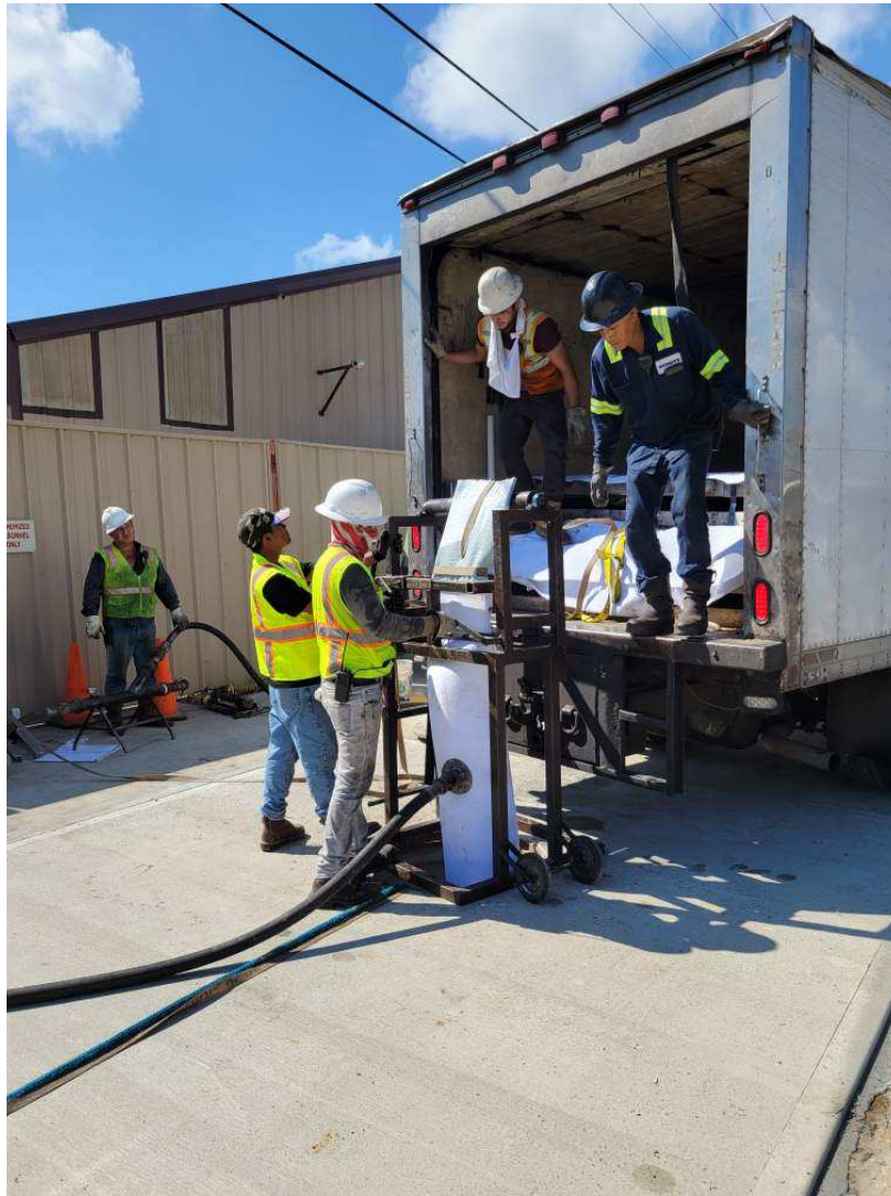
INSTALLATION OF CIPP (CURED IN-PLACE PIPE) FOR MLK TO US 90
