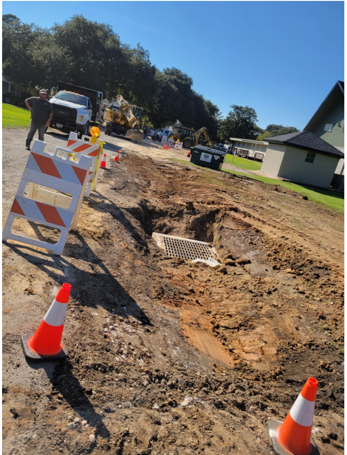
Heights St. storm drainage installation complete
