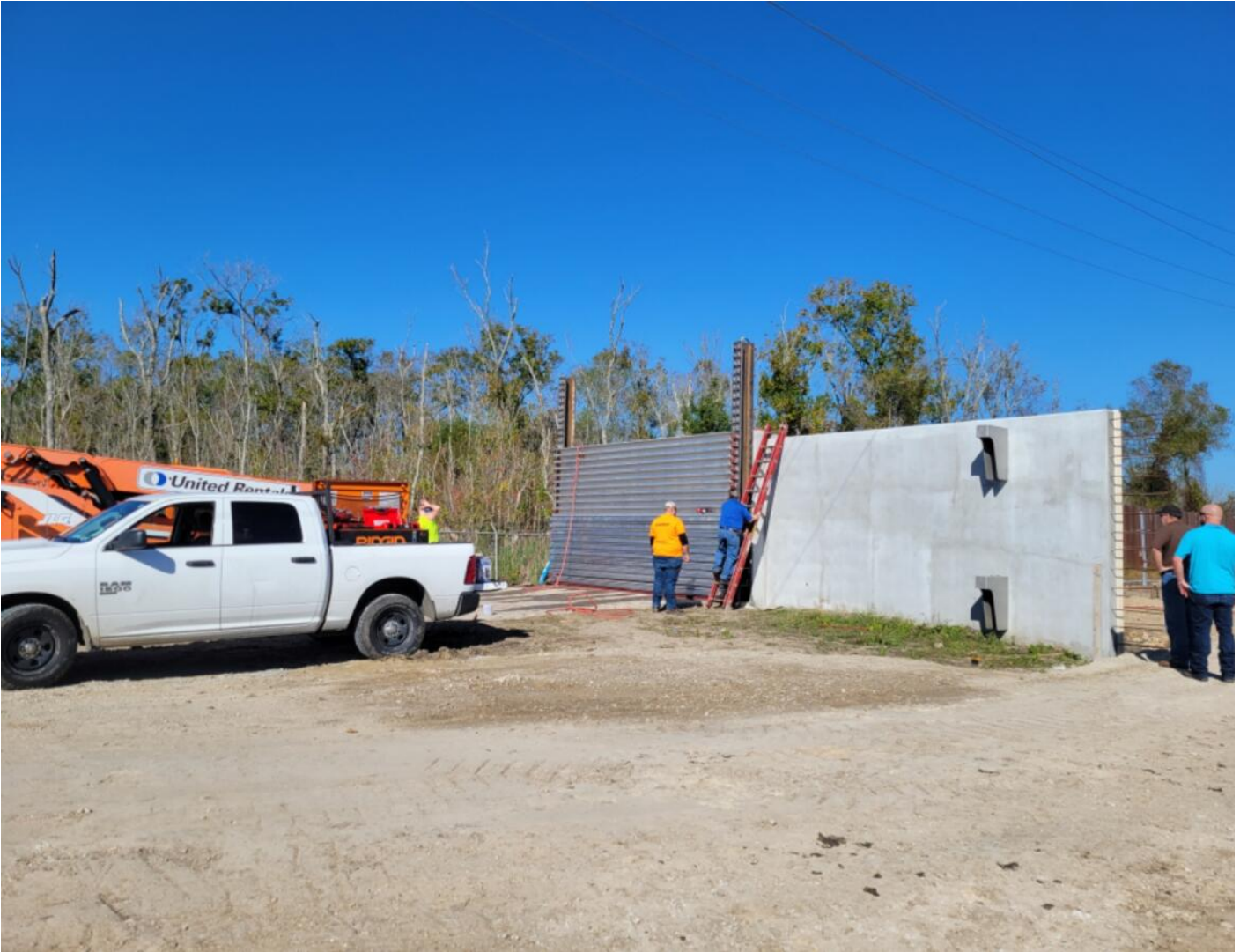
INSTALLATION OF FLOOD GATE
