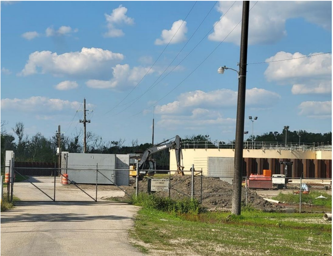
INSTALLATION OF FRONT WALL
