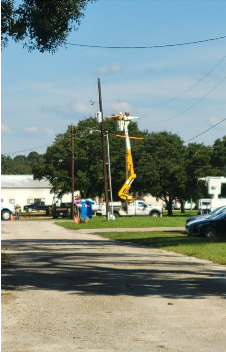
Texas Elite upgrading service on Chrysler St.
