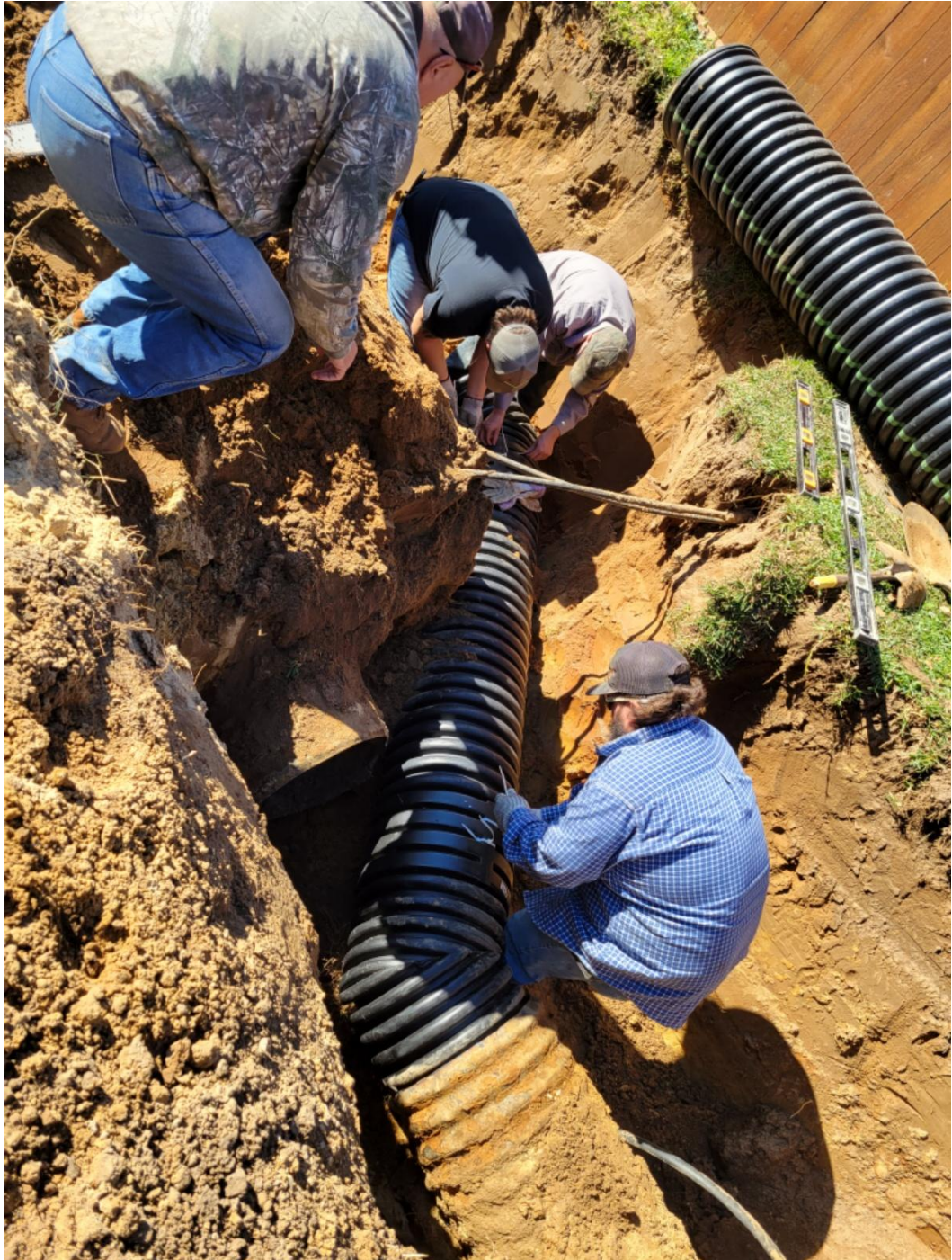
Kipling storm drainage installation complete; Brandon Taylor, Joey Widdon, Nathan David, Rick Ubnoskye
