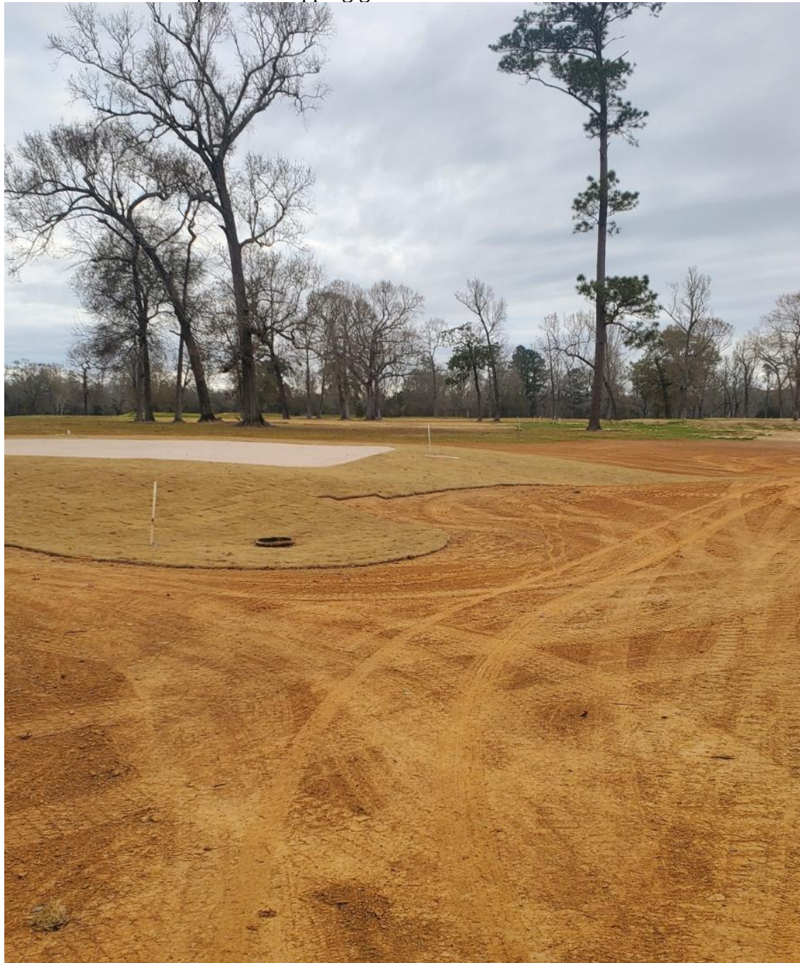
Sod installed around practice chipping green
