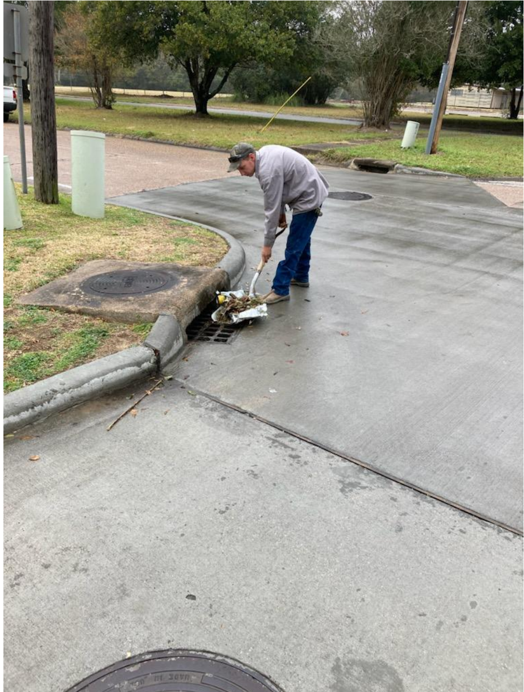
Storm drainage preparation – cleaning inlets on Grand St.; Nathan David
