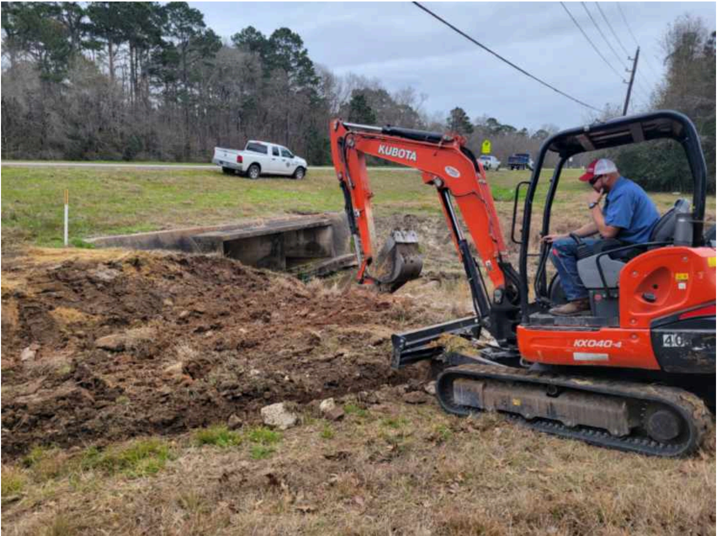
David Allison completing the backfill and grading for the waterline protection.
