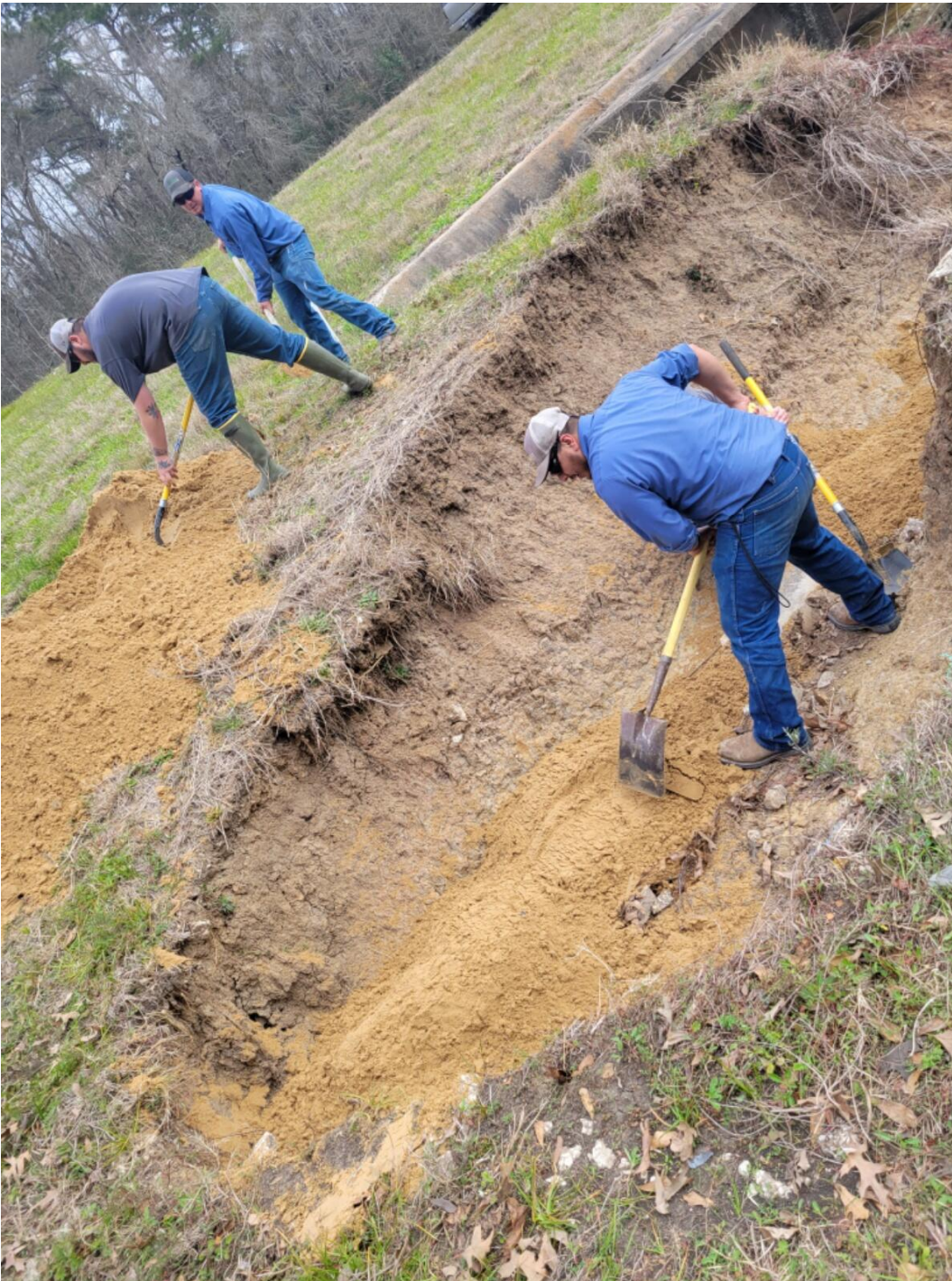
Water and Streets Departments working together to prevent a serious waterline failure on the Bypass near Grace Church – Stephen Davila, David Driskell and Joel Burris.
