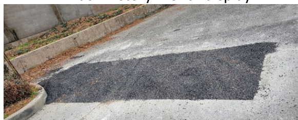
Completely repaired former sinkhole
