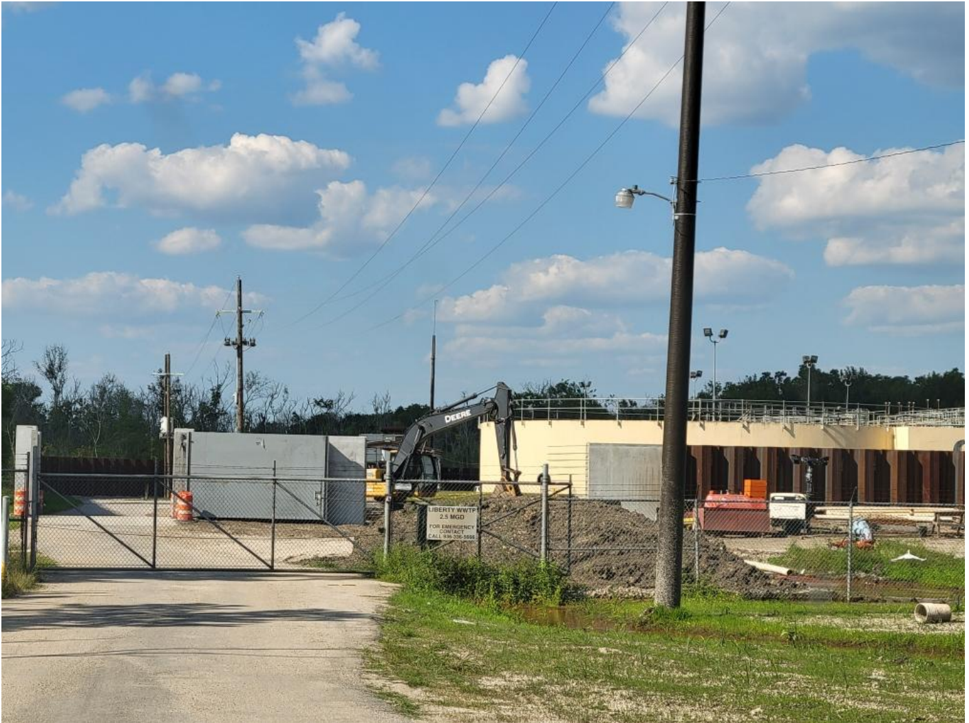
SHEET PILING ALONG THE FRONT OF THE WW TREATMENT PLANT. FLOOD GATE BEING INSTALLED
