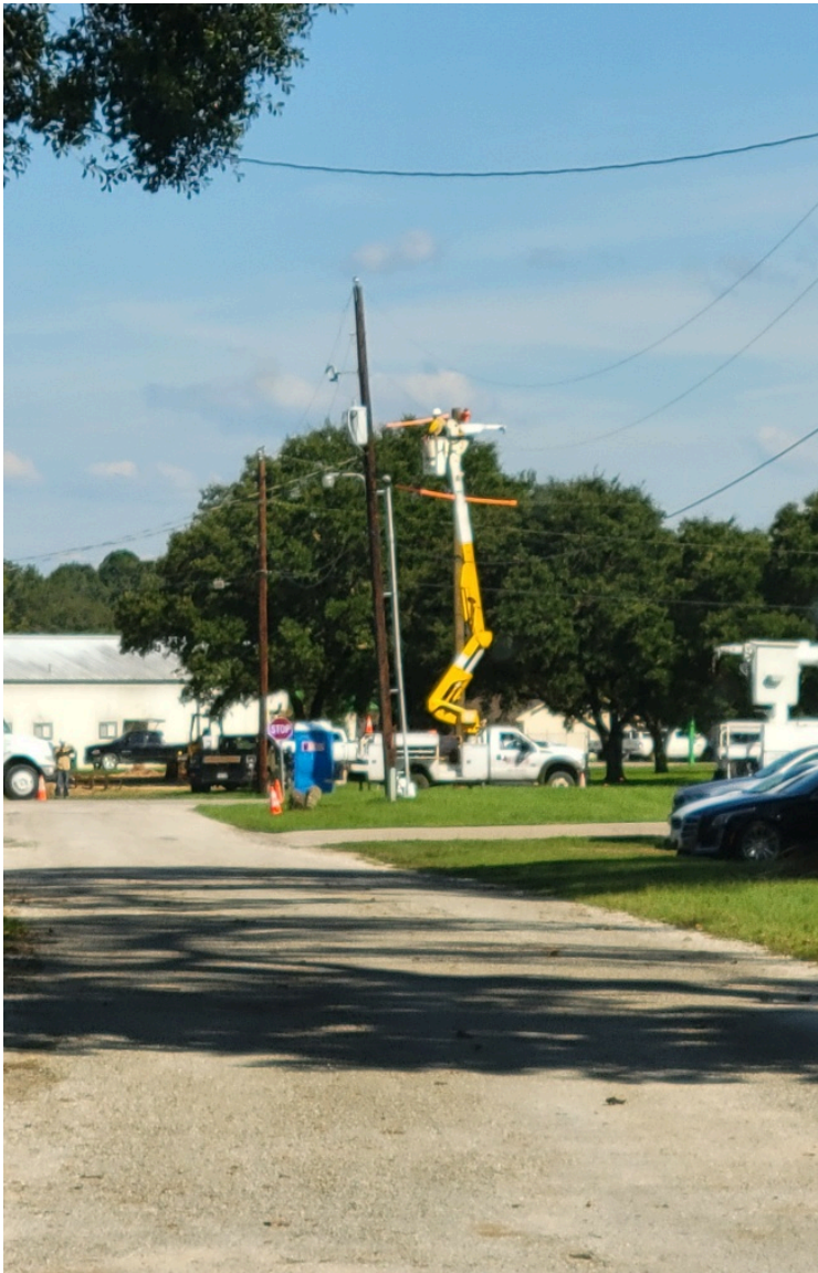
Texas Elite upgrading service on Chrysler St.
