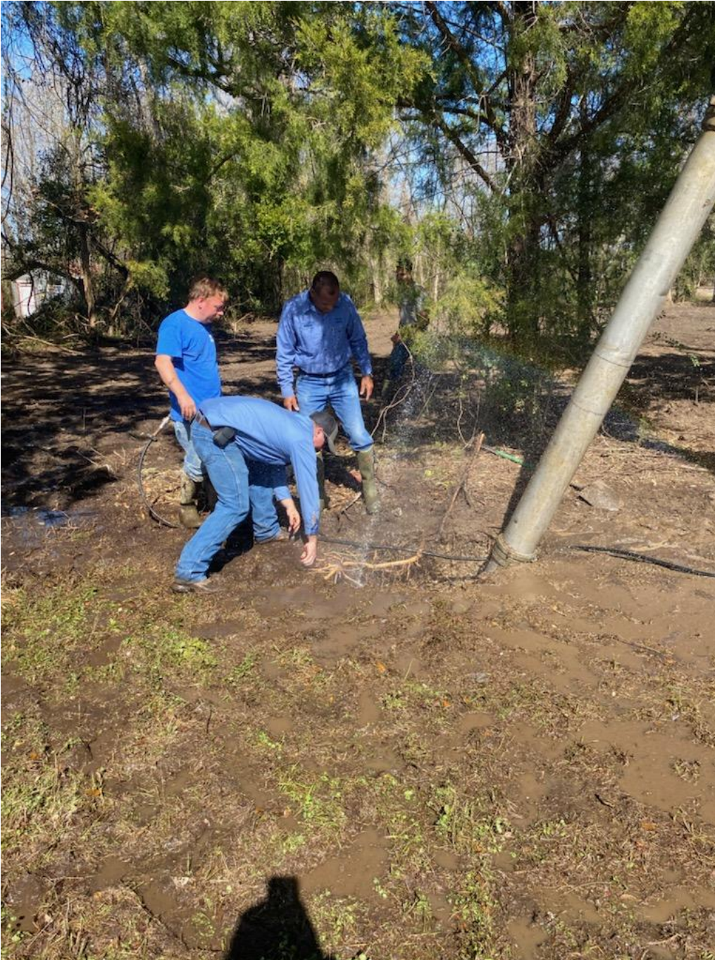
Water and Streets Departments working together to prevent a serious waterline failure on the Bypass near Grace Church – Wayne Burell, David Driskell and Robert Edmonds.
