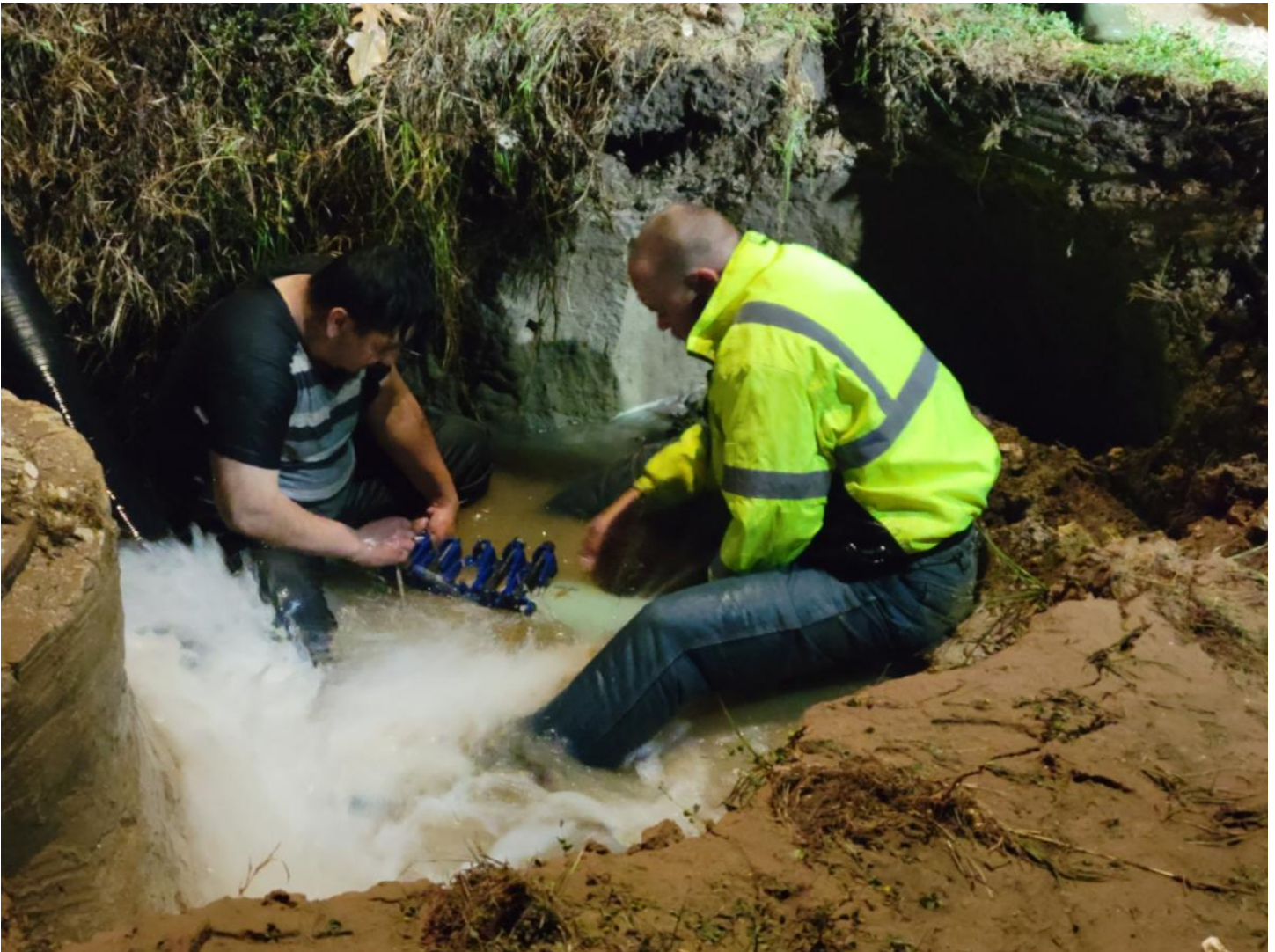
David Allison and Stephen Davila repairing a 6" water main on Crockett and M.L.K.
