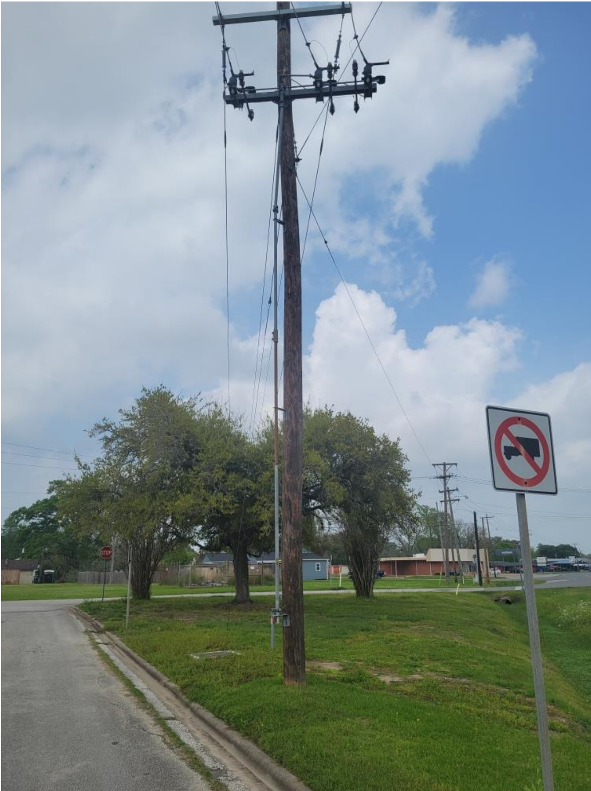
KNIFE BLADE SWITCH – Main St. and Monta St.
