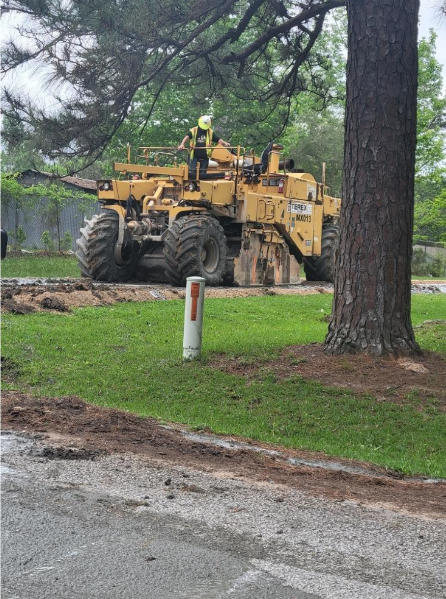
MIXING THE EXISTING PAVEMENT WITH THE CEMENT SLURRY ON AVENUE I
