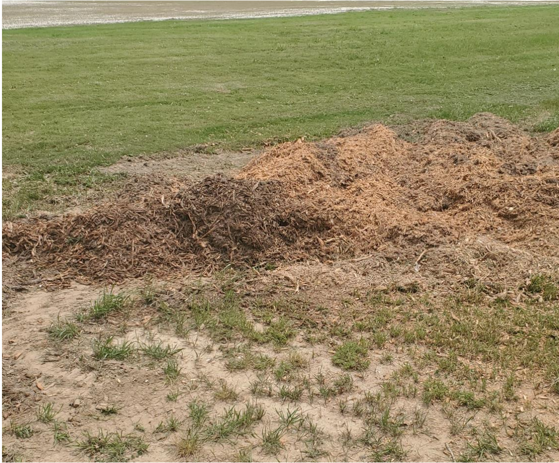
Contractor grinding stumps from trees that were recently cut down
