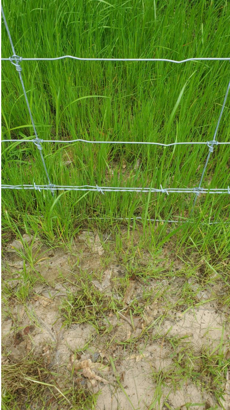
Contractor installing barbed wire on the hog fence
