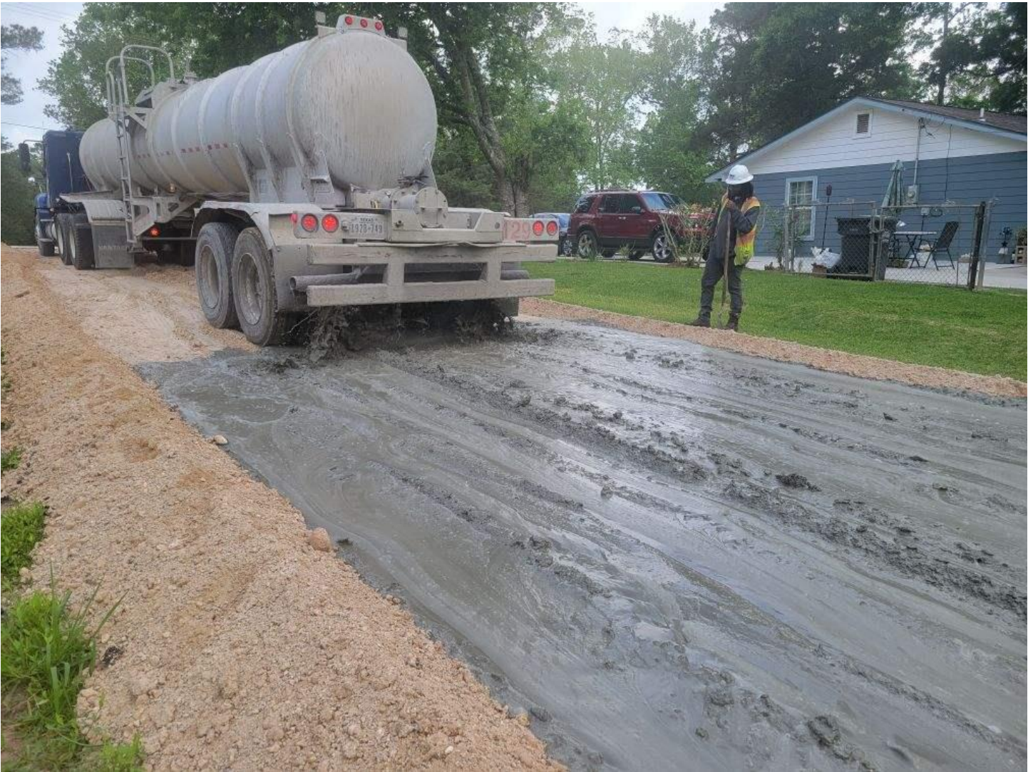
AVENUE H (4% TO 6%) CEMENT SLURRY STABILIZATION
