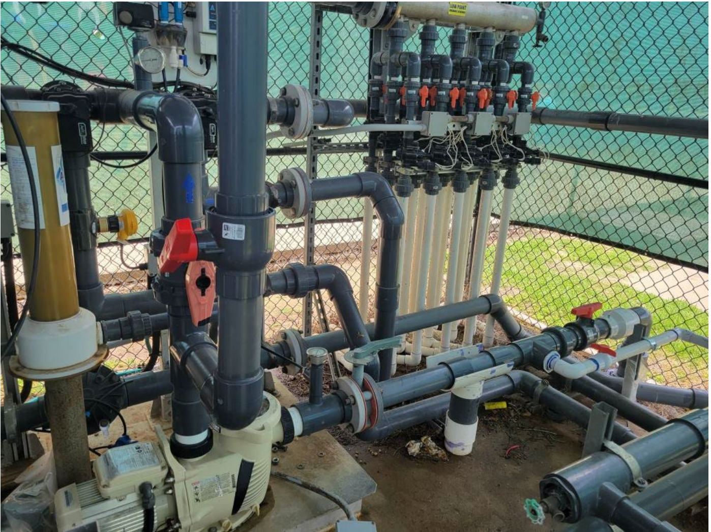
ALL THE WORK NEEDED TO GET THE SPLASH PAD OPERATIONAL
