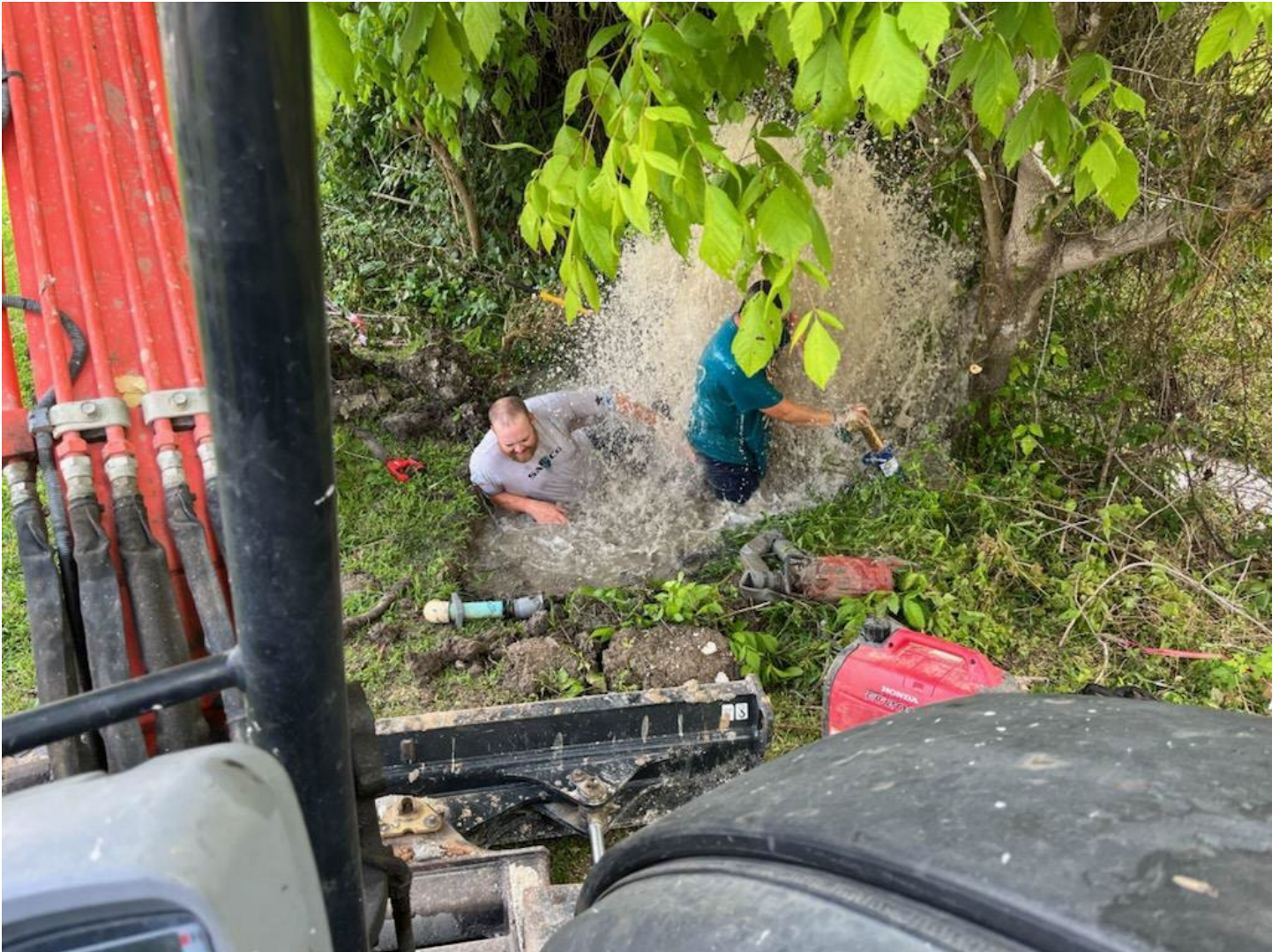
DALE AND DAVID FIXING A WATER LEAK BEHIND ALLEGIANCE BANK ON MAIN ST.
