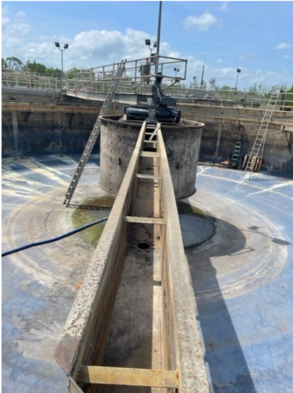
Wastewater Treatment Plant Clarifier Repair
