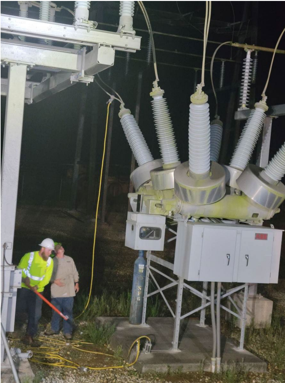
WORK DURING THE CITY-WIDE SCHEDULED OUTAGE AT LIBERTY AND BOOMERANG SUBSTATIONS
