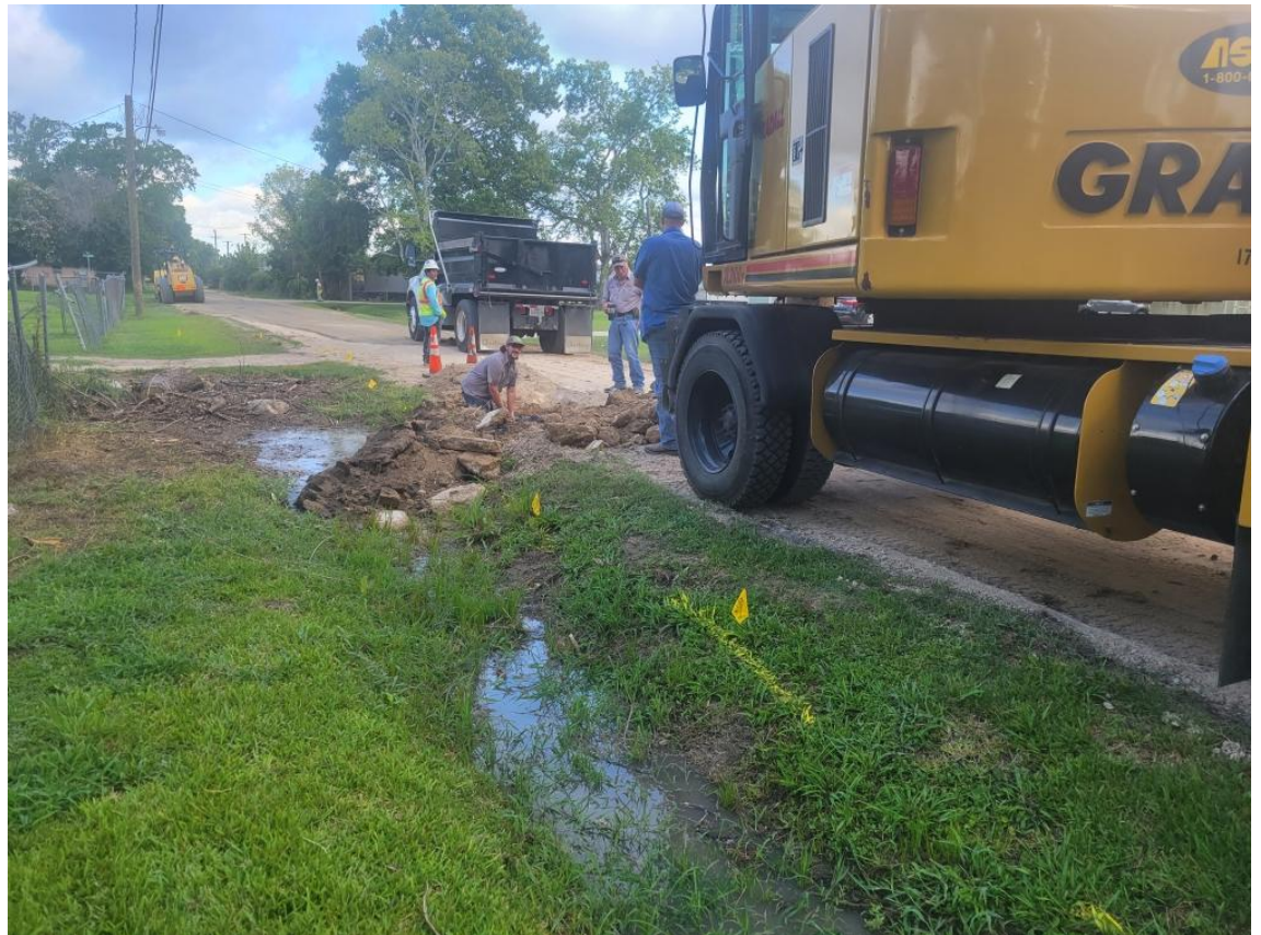
BRANDON IN STREETS FIXING A SEPARATED DRAINAGE CULVERT ON SANTA ANNA ST.
