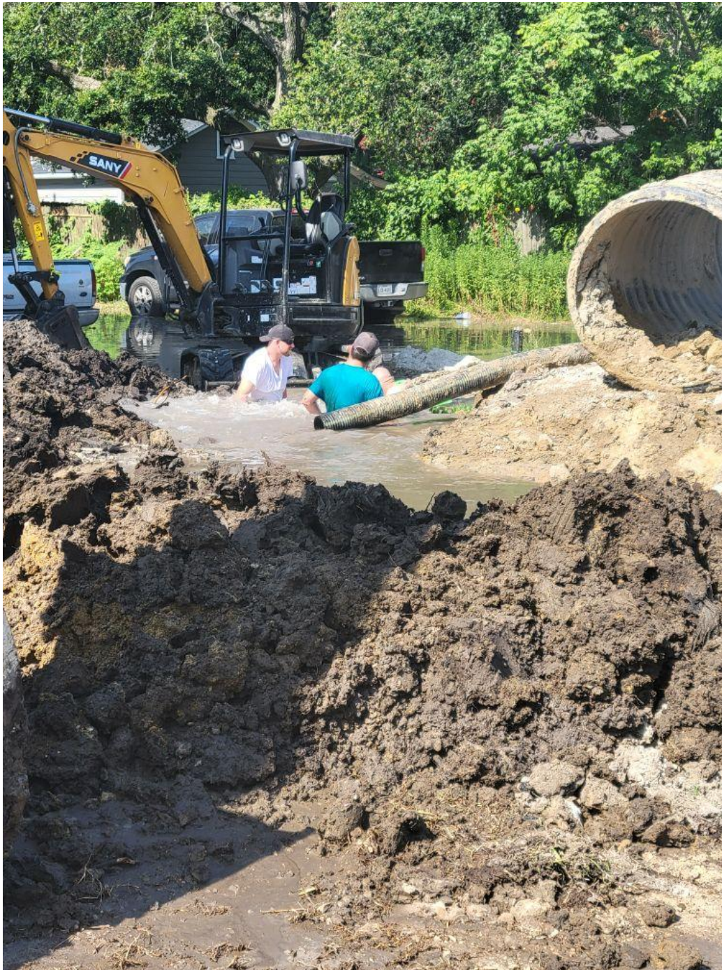
WATER DEPARTMENT AT IT AGAIN!!!! CHRISTIAN, DALE AND DAVID ON MONTA
