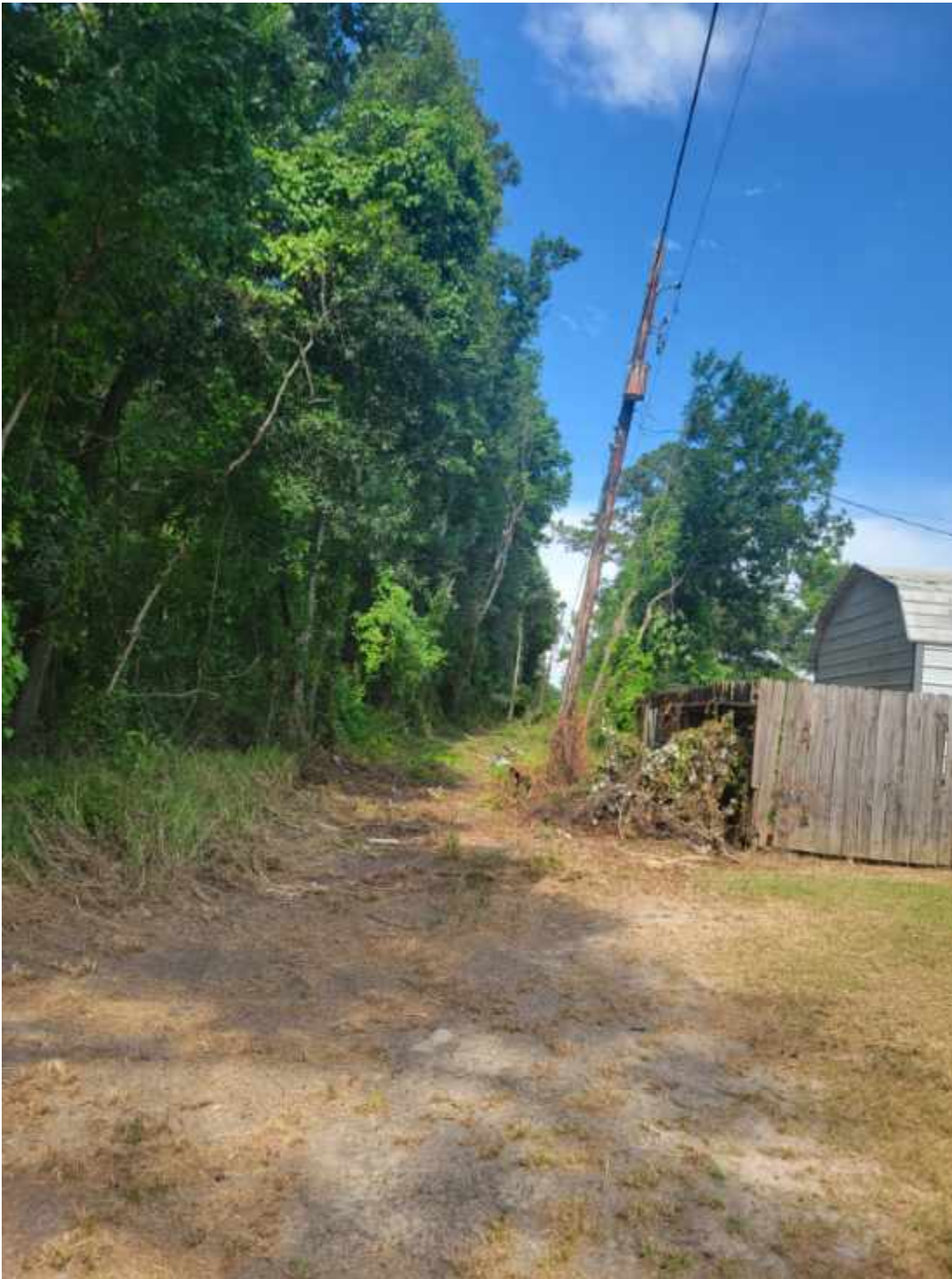
Briar St easement – done by Tree Trimmers
