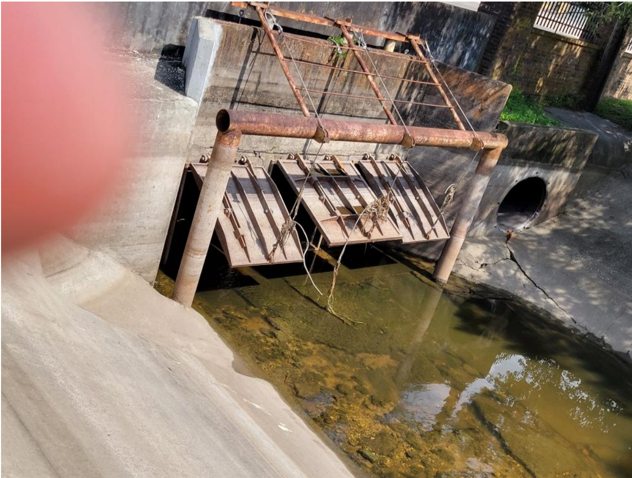
Main B with the flap gates opened on July 23, 2021 and remain open 6/30/2022
