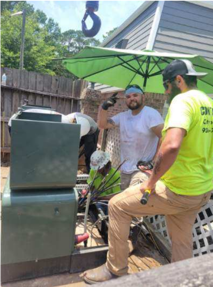
Travis Villa Apartments, replacing bad connections and primary by Texas Elite.
