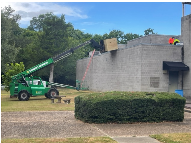
The repair project got underway on the roof.
