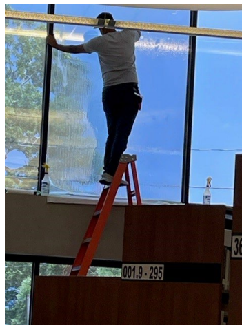
Installing new UV film on the east addition windows.
