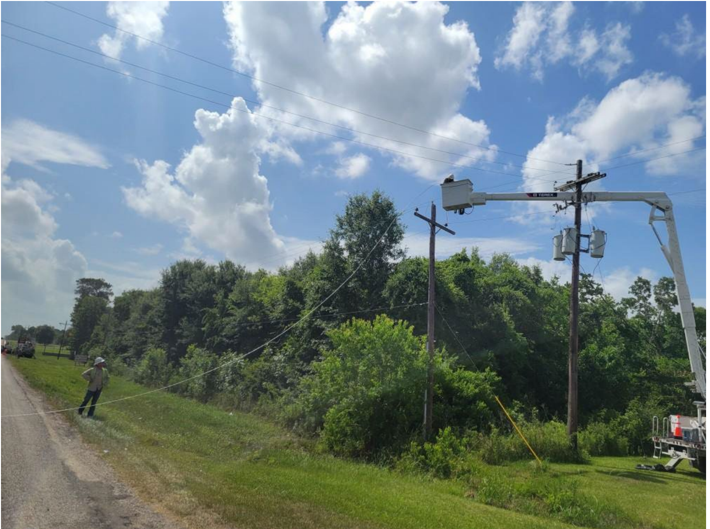
TEXAS ELITE REPAIRING A DOWNED POWER LINE ON US 90 BY AN OVERSIZED LOAD
