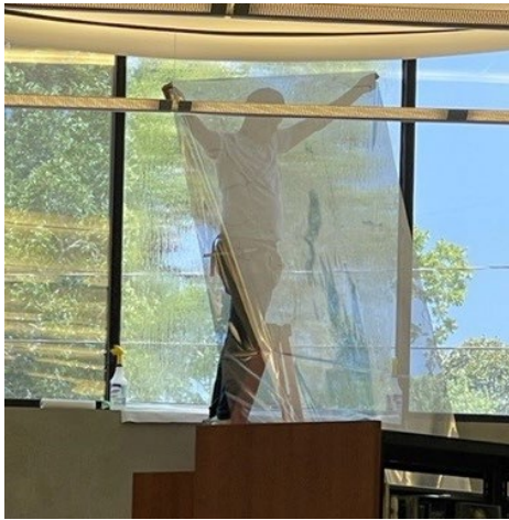
Installing new UV film on the east addition windows.
