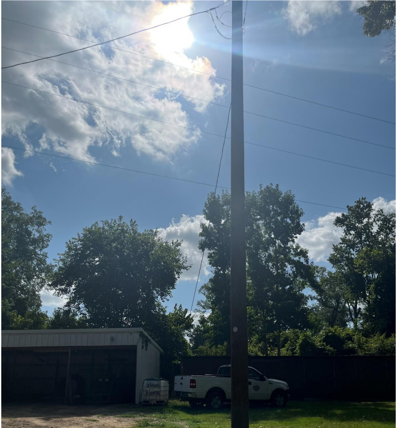
Entergy installing new pole to get lines off maintenance building
