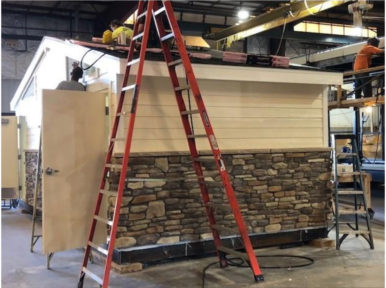
Photos of new restroom to be installed at golf course
