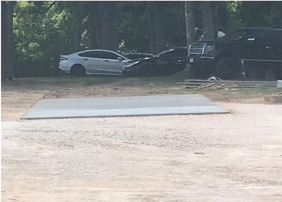
Concrete for new dumpster pad
