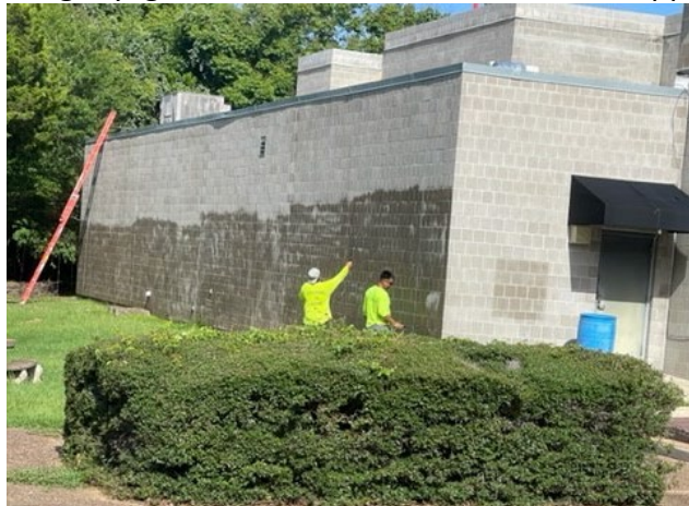
Hand-spraying the waterproofing.
