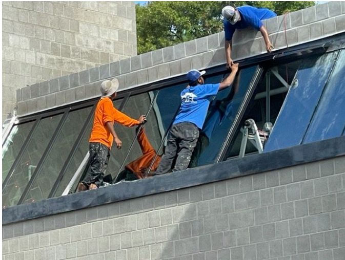
Workers installing skylights.
