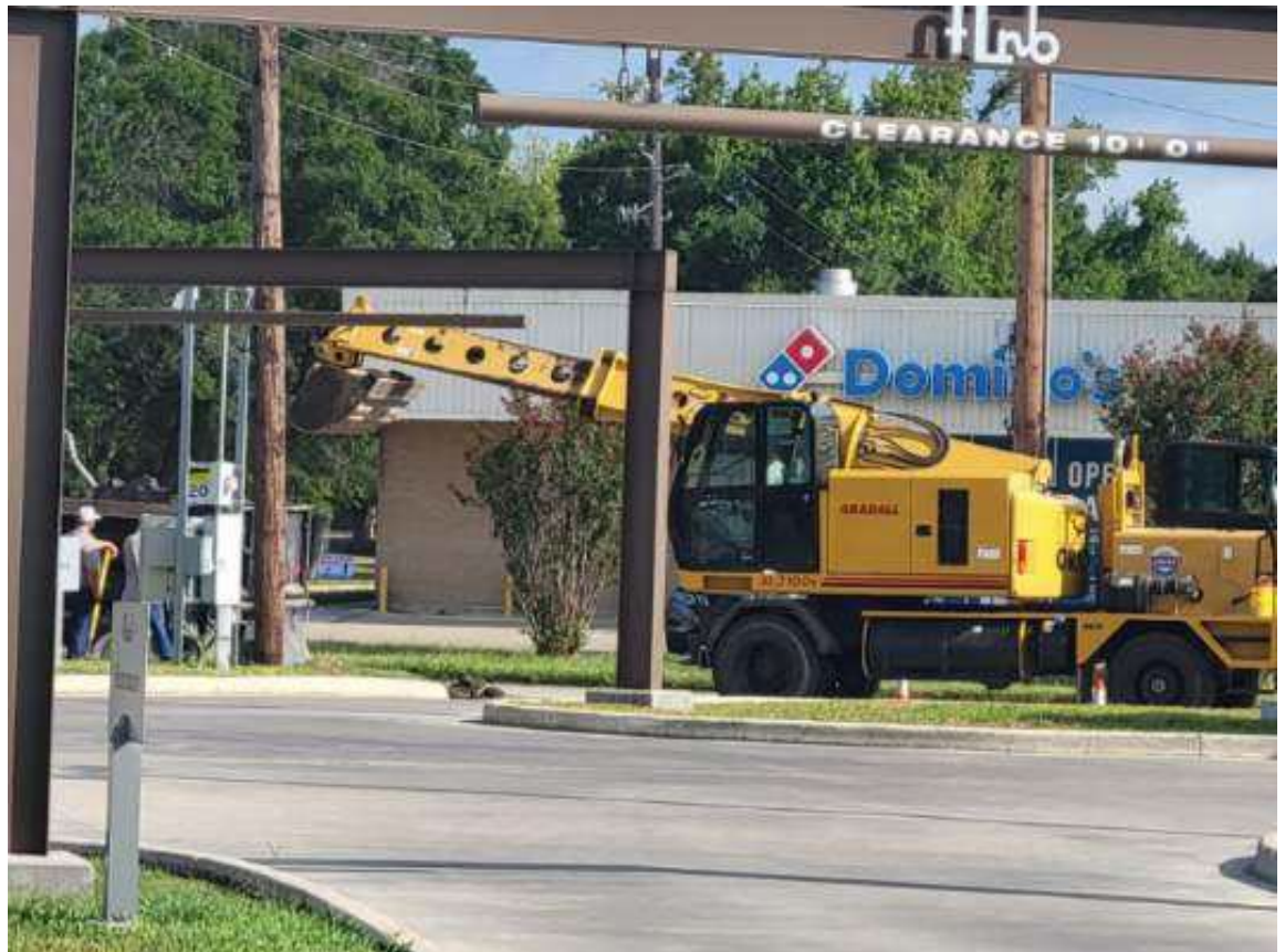
STREETS WORKING ON FIXING JEFFERSON ST AT MAIN ST.
