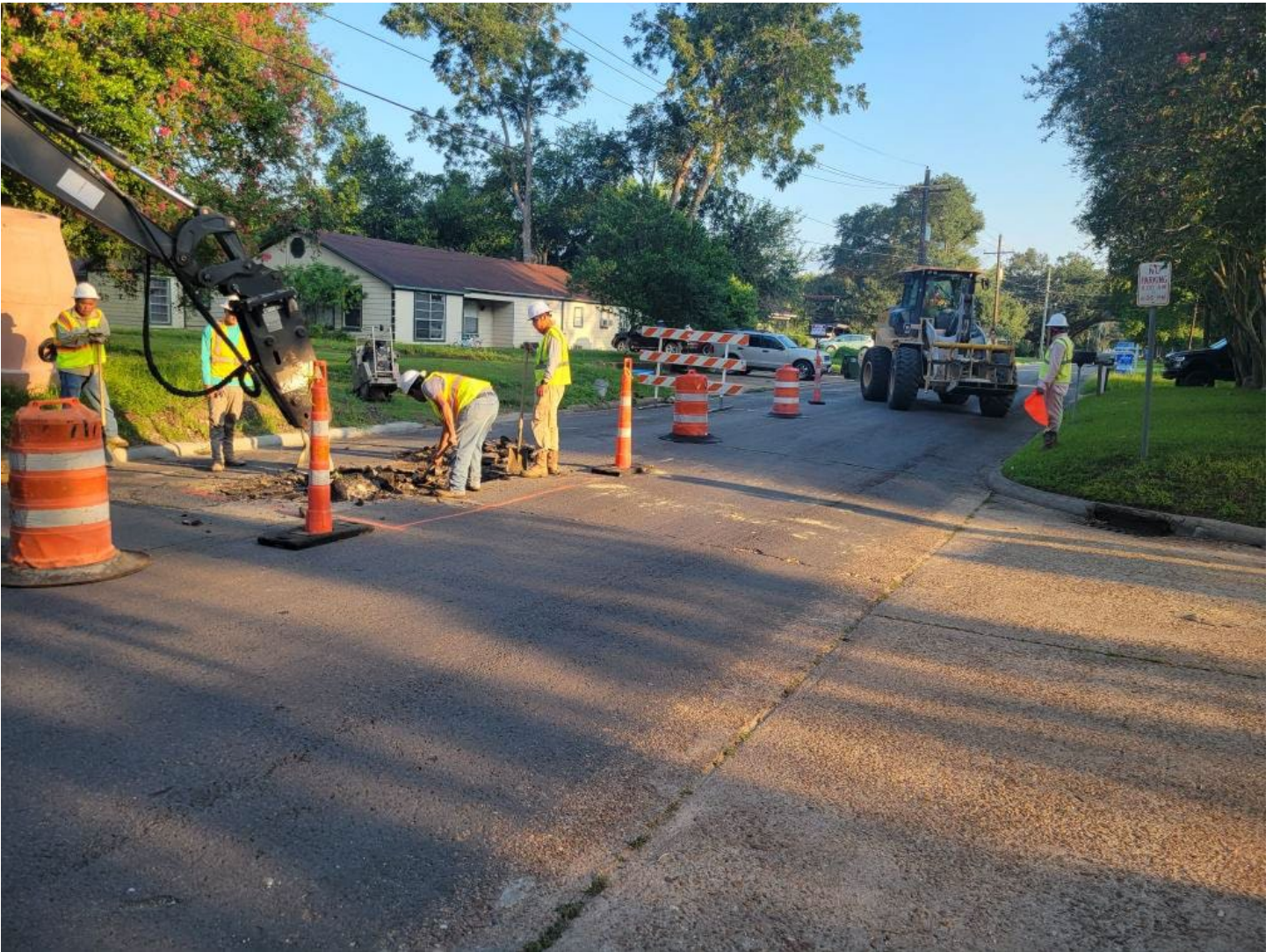
SANITARY SEWER WORK ON NORTH TRAVIS
