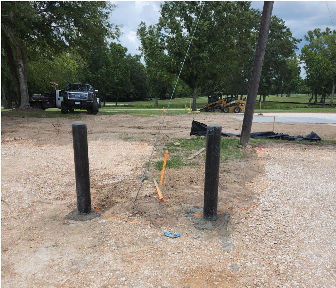
Bollards have been installed
