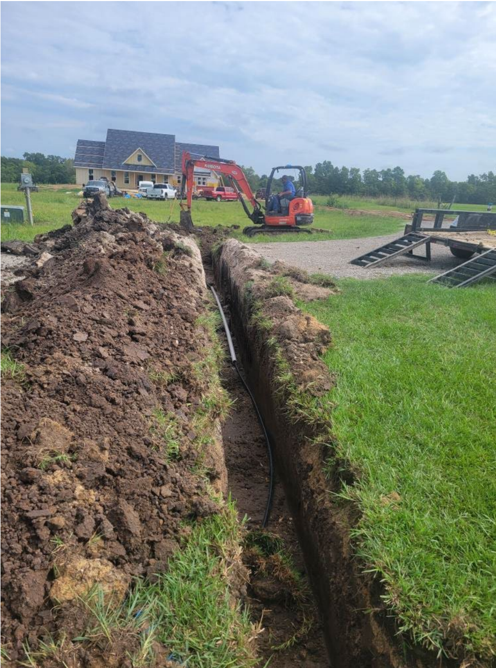
WATER TAP ON TIMBER RIDGE
