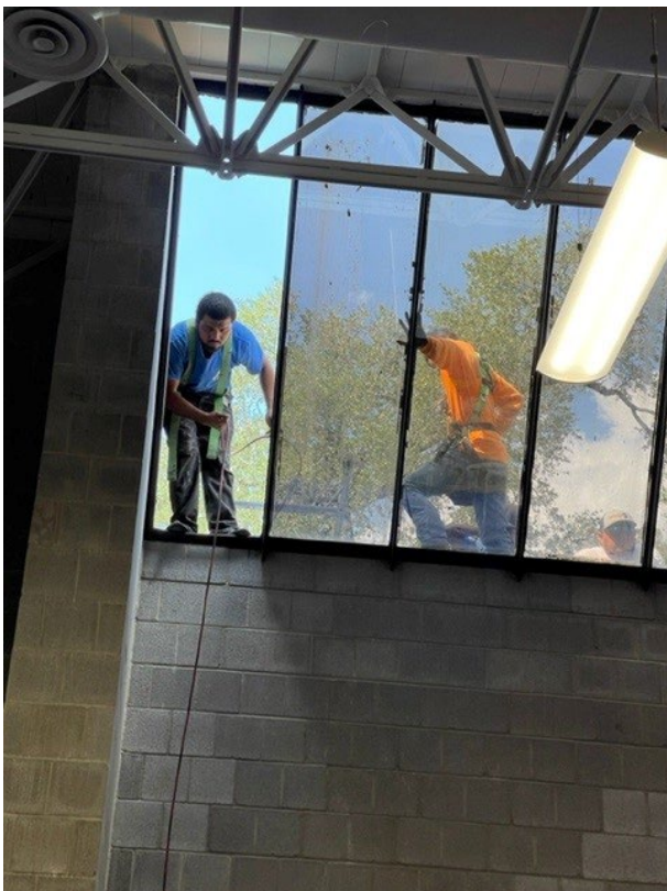
The first skylight has been removed.
