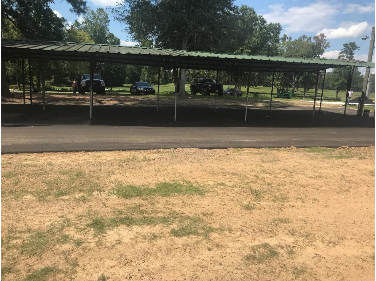
Paving under cart barn
