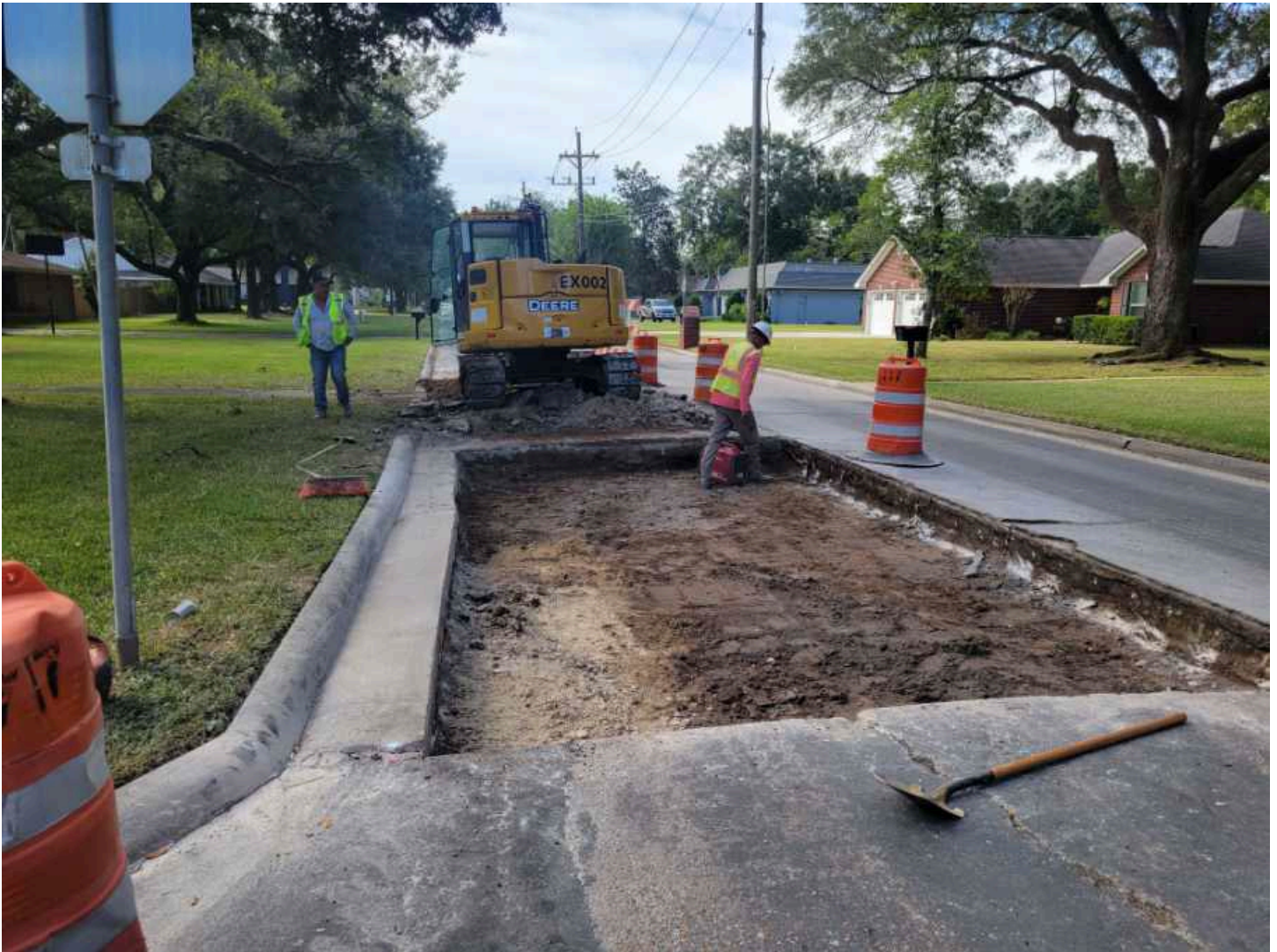
FULL_DEPTH CONCRETE REPAIR WORK ON NORTH TRAVIS AND JEFFERSON
