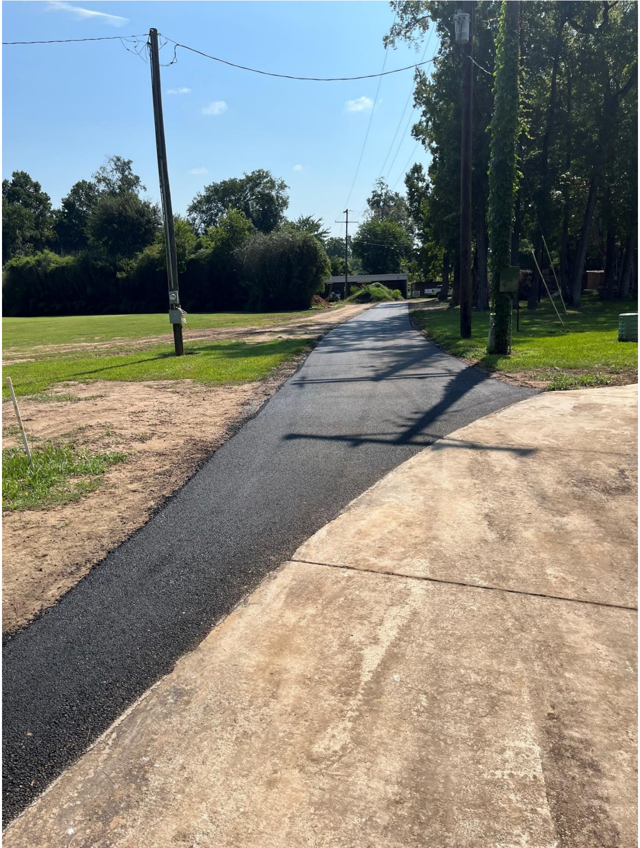
Paved road to the maintenance area
