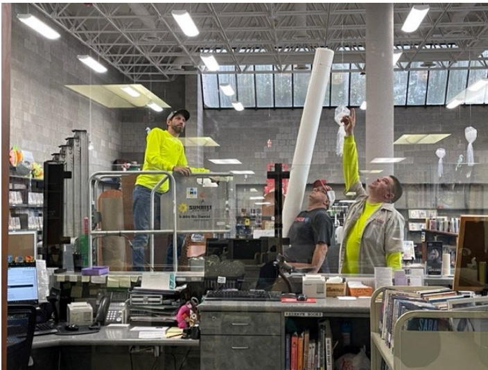
Plumbers consulting on the placement of pipe
