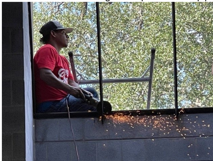
Cutting out old rusted skylight frames.
