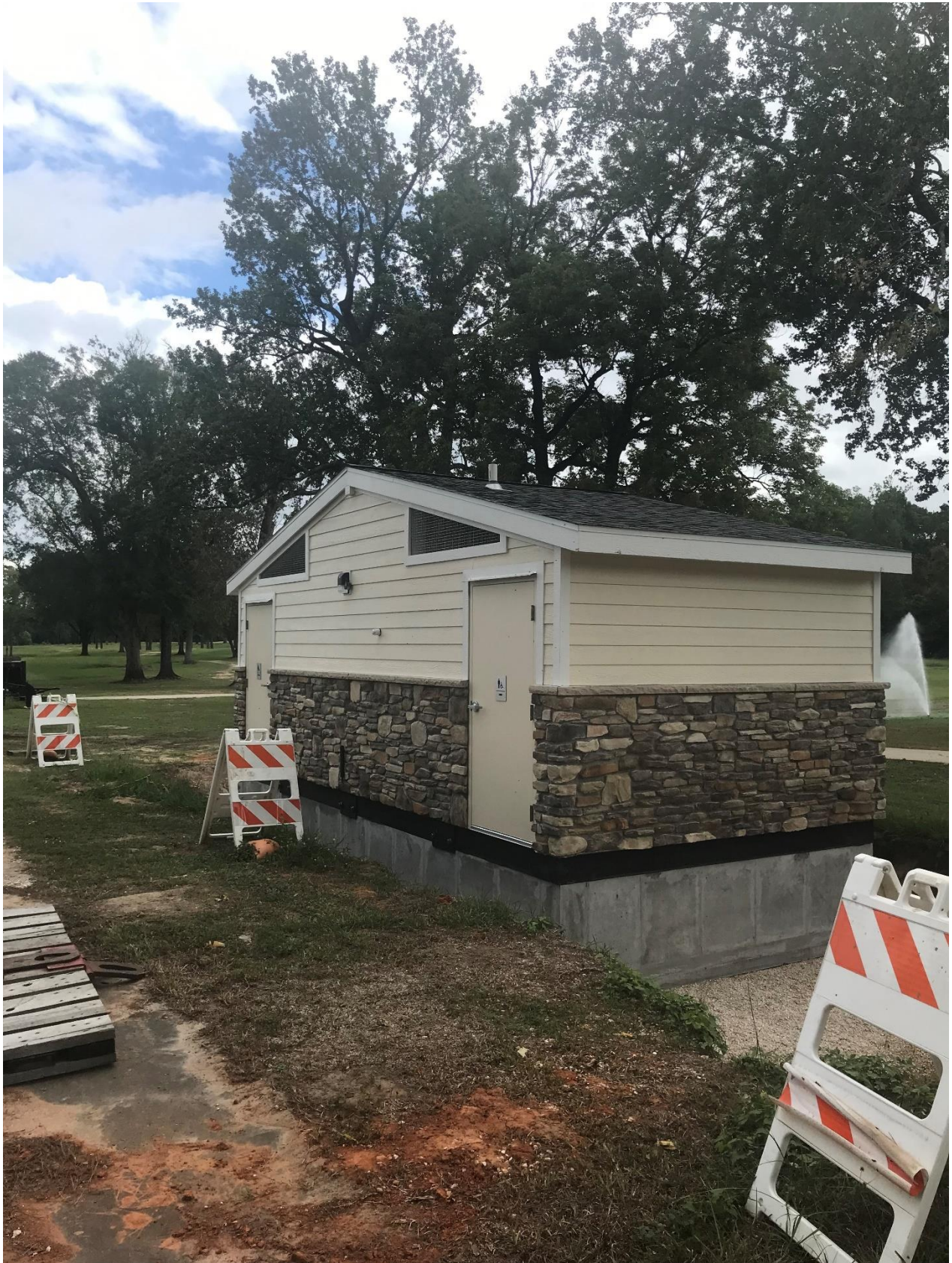
New restroom set in place
