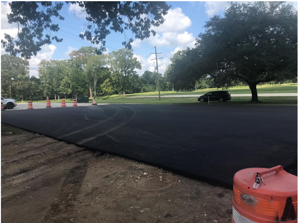
Expanded parking lot near clubhouse
