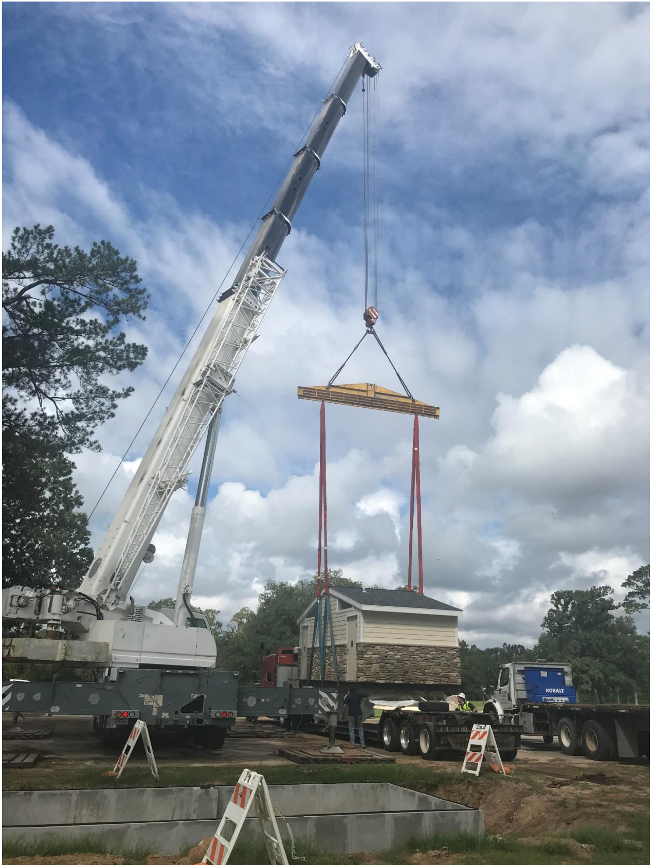
Crane lifting restroom into place
