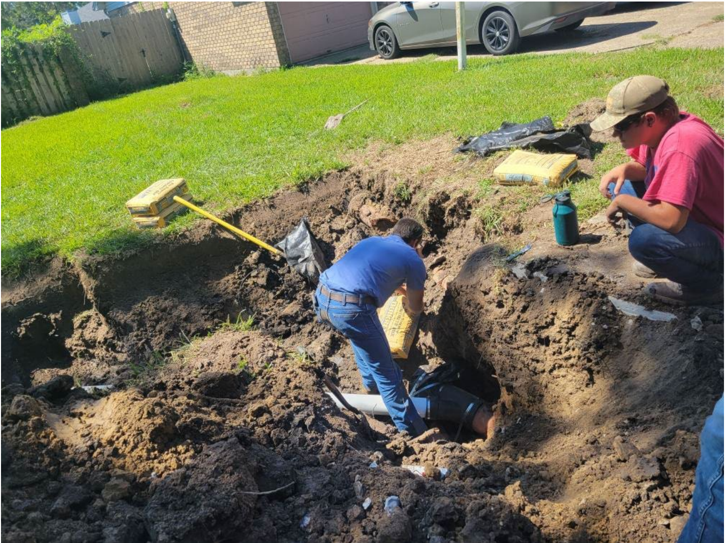
CHRISTIAN AND MICHAEL REPAIRING BROKEN SEWER PIPE ON VALLY DR.
