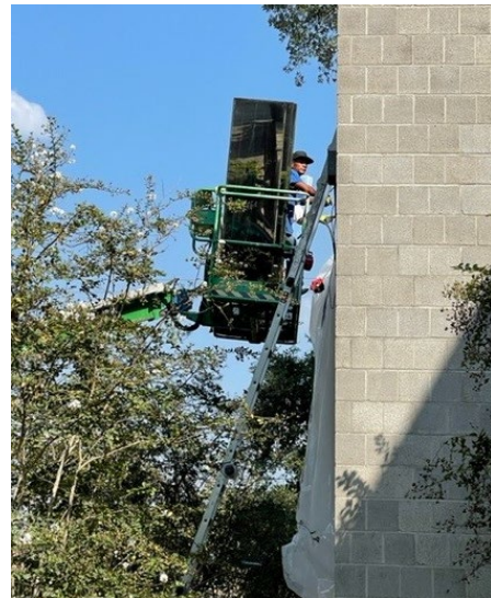
Outside skylight installation
