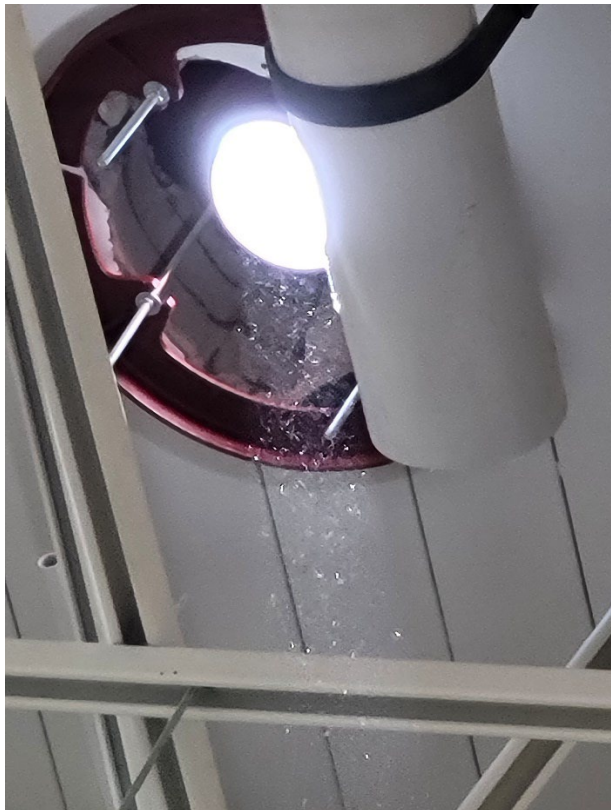
The air was full of construction dust.
