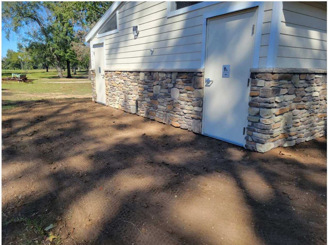
Water and electric installed and backfill complete around new restroom
