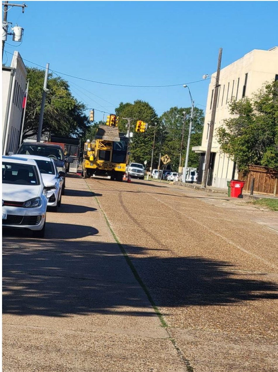
STREETS REPAIR A BAD BUMP ON SAM HOUSTON AND MAIN
