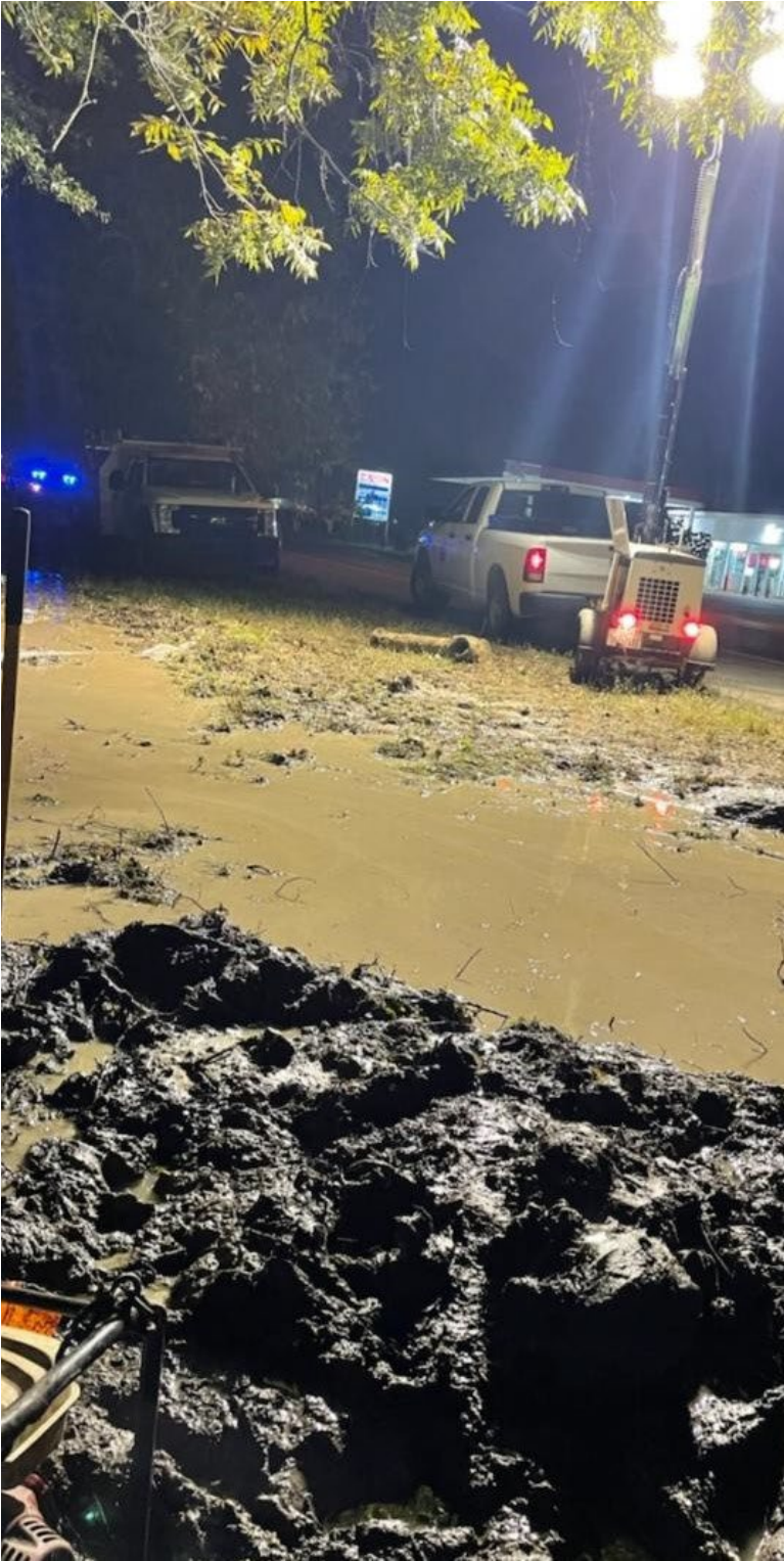
WATER LEAK ON NORTH MAIN ACROSS FROM RIDGEWOOD
