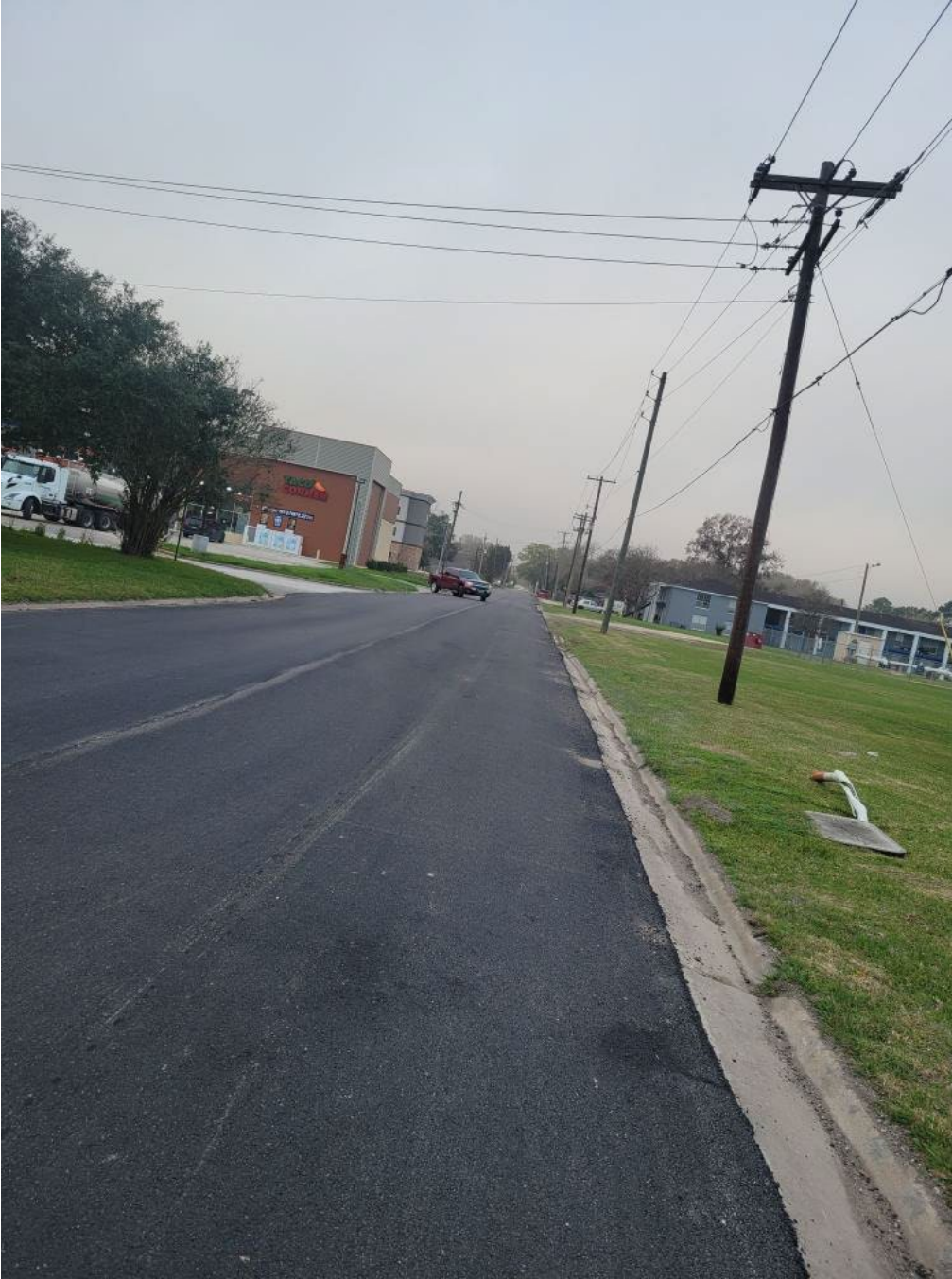
MONTA STREET WAS FRESHLY PAVED ON DECEMBER 5 TH
