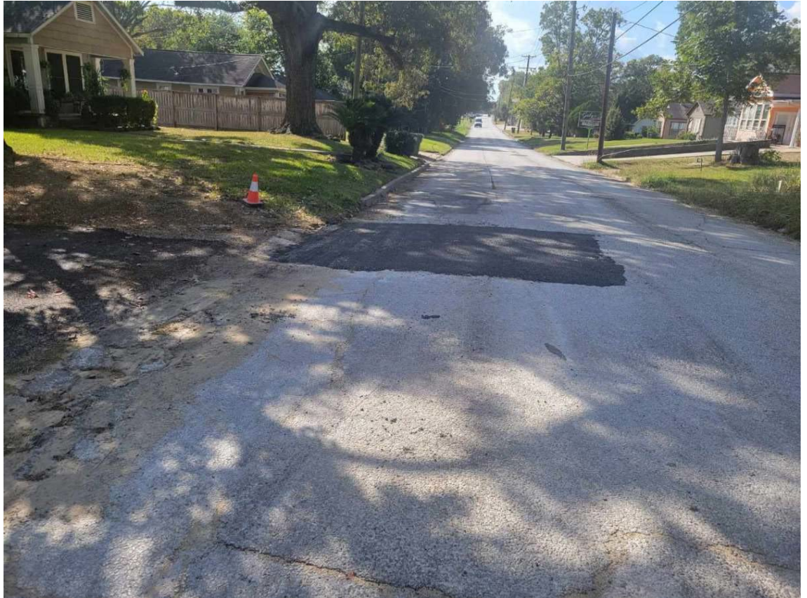
STREETS REPAIRED A UTILITY STREET CUT ON BEAUMONT ST
