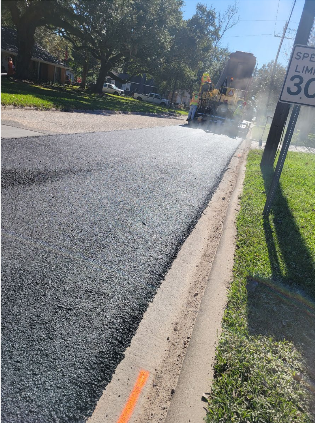
NORTH TRAVIS 1" LEVEL-UP SOUTHBOUND LANE DECEMBER 15 TH , 2022
