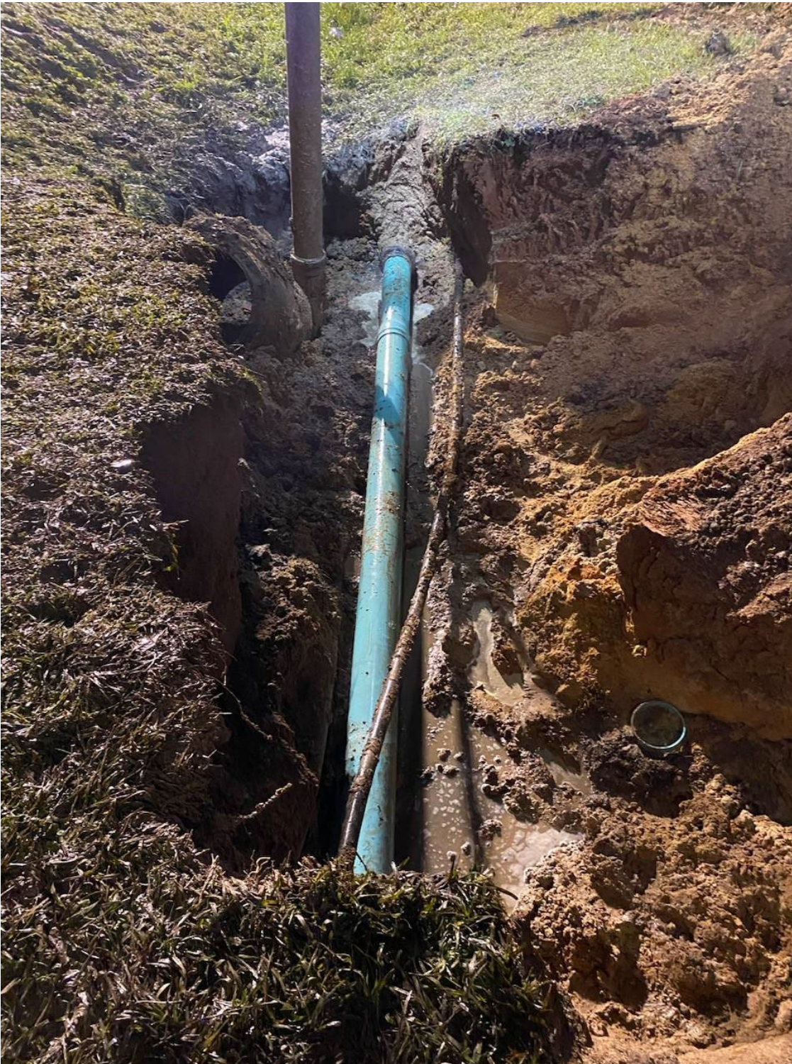
COMPLETED SEWER REPAIR IN FRONT OF SUBWAY
