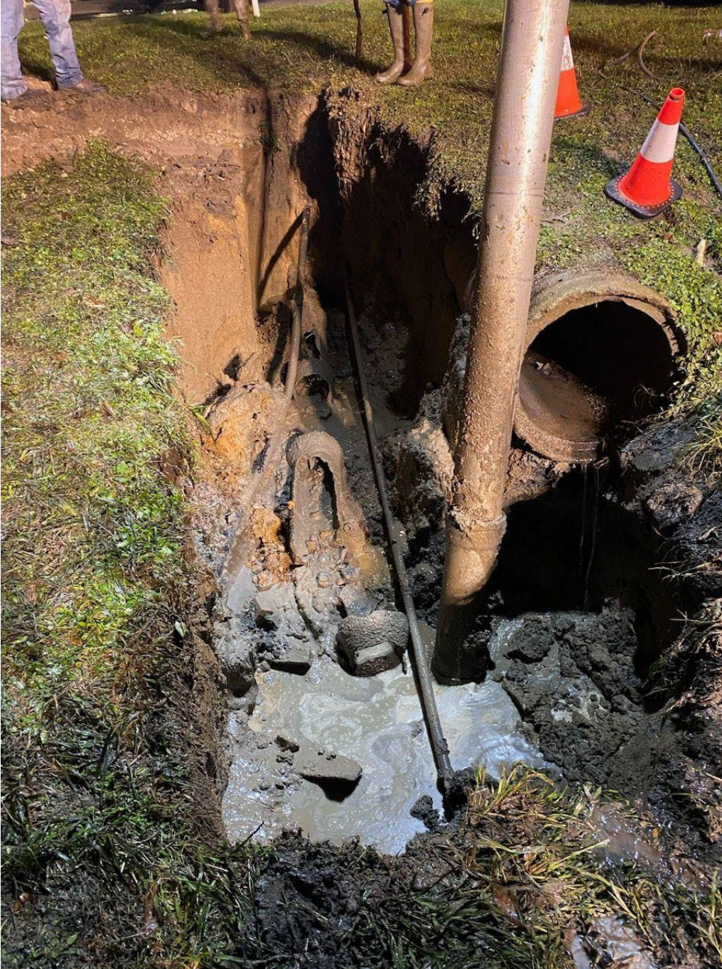
SEWER REPAIR ON MAIN ST IN FRONT OF SUBWAY
