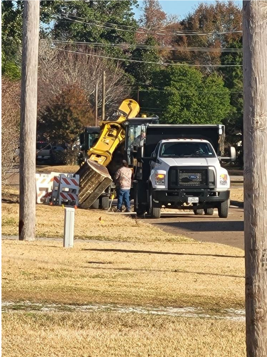
STREETS REPAIRED A UTILITY STREET CUT ON KIPLING ST
