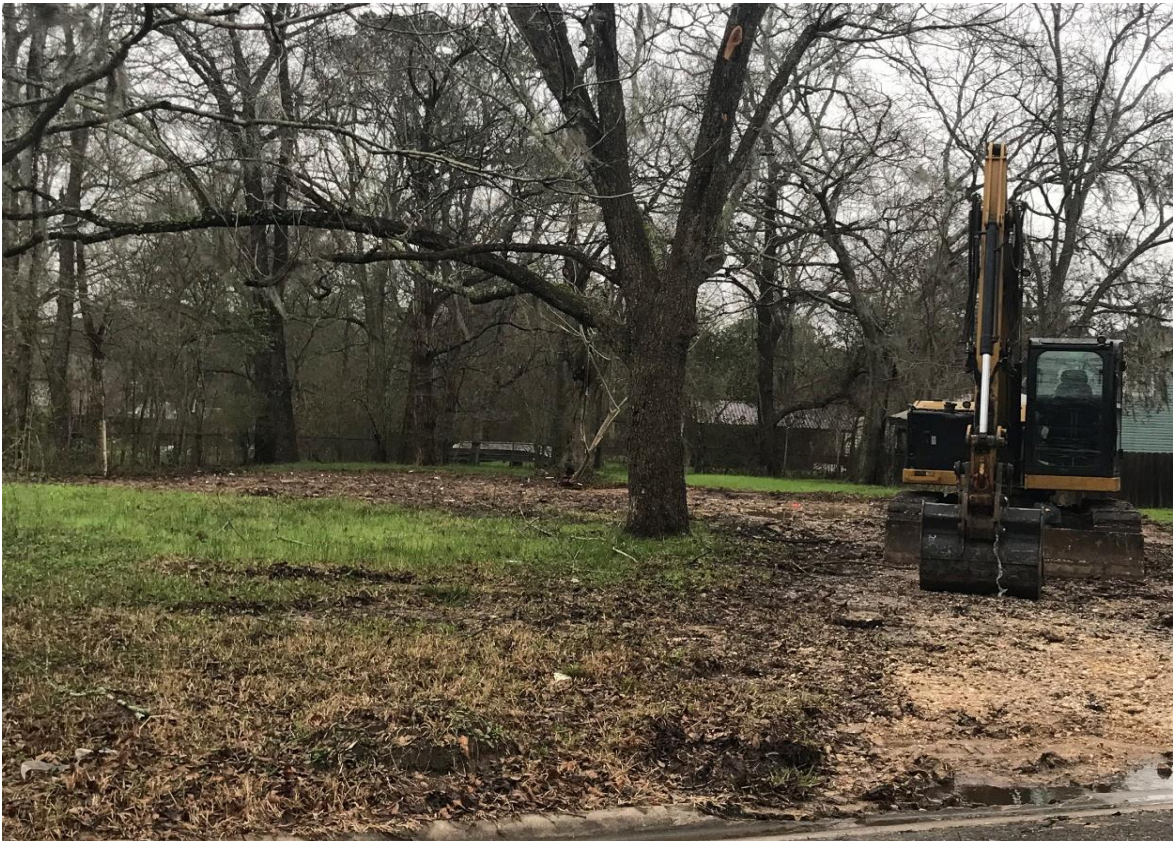
Completed demolition of 408 Independence
