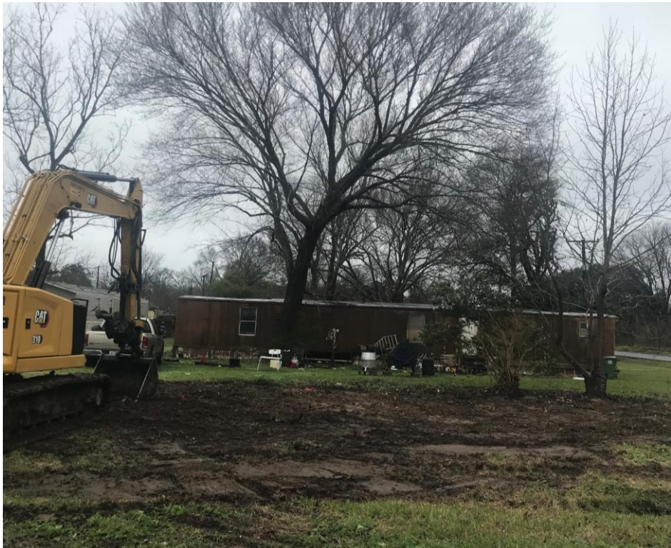
Completed demolition of 128 Carter (Unit A)
