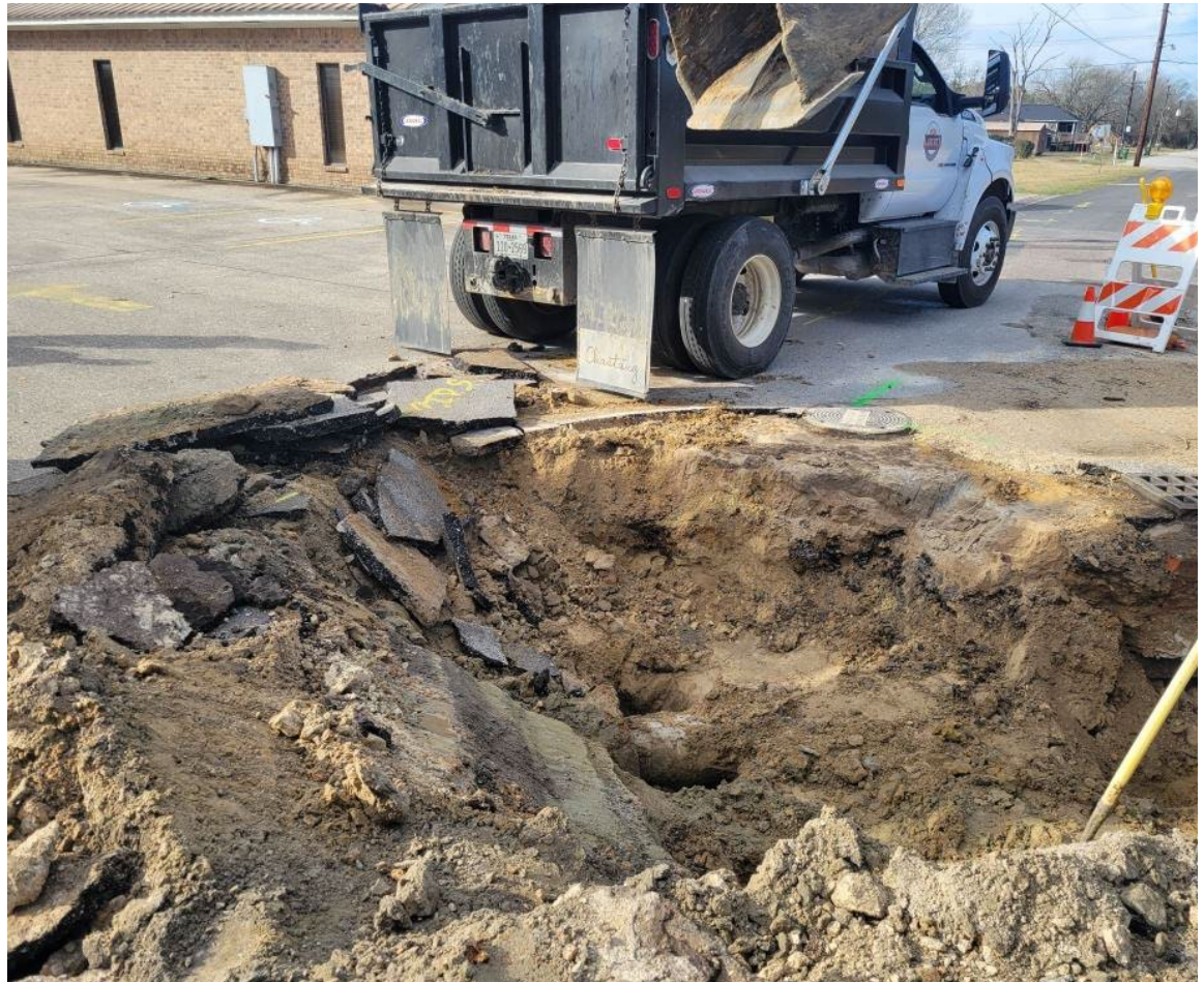
STORM SEWER REPAIR AT THE 800 BLOCK OF WASHINGTON
