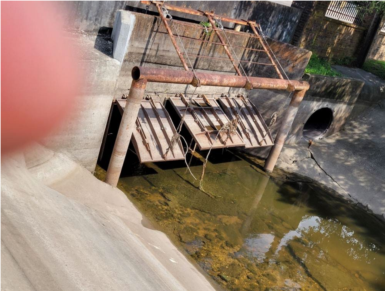
Main B with the flap gates opened on July 23, 2021 and remain open 1/31/2023.
