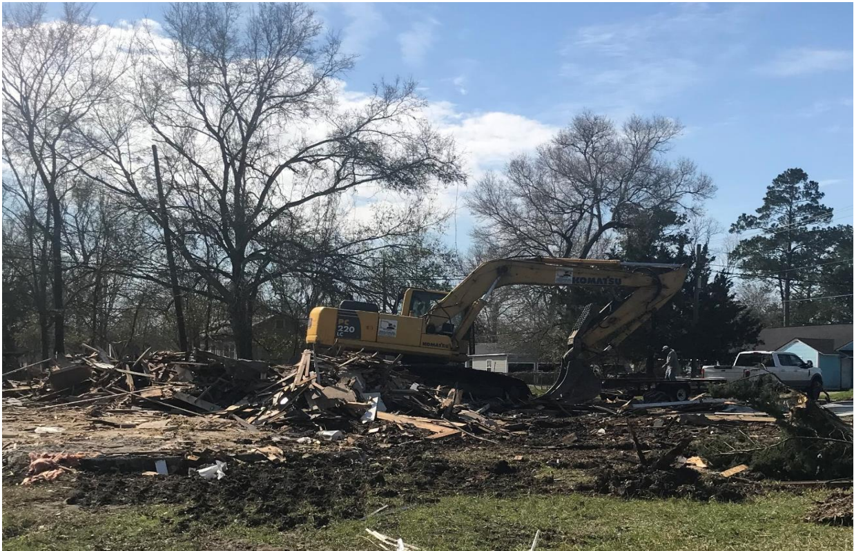
Voluntary demolition of 514 Davidge
