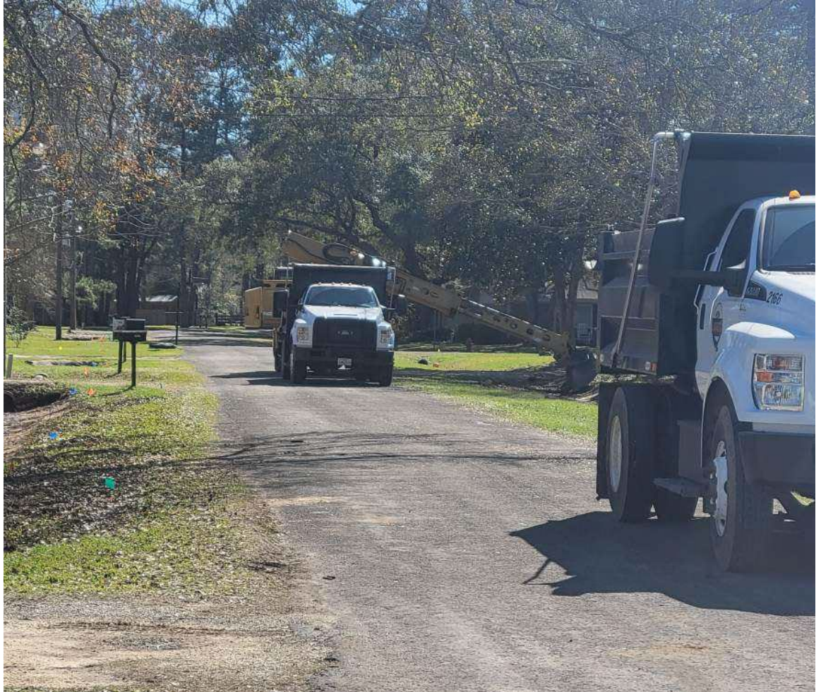
DITCHING IN RIDGEWOOD
