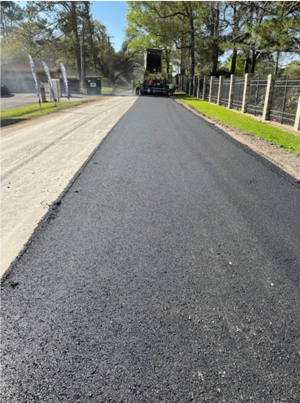
NORTH TRAVIS BETWEEN JEFFERSON AND THE TRAVIS PARK CROSSING 1" LEVEL-UP PLACEMENT
