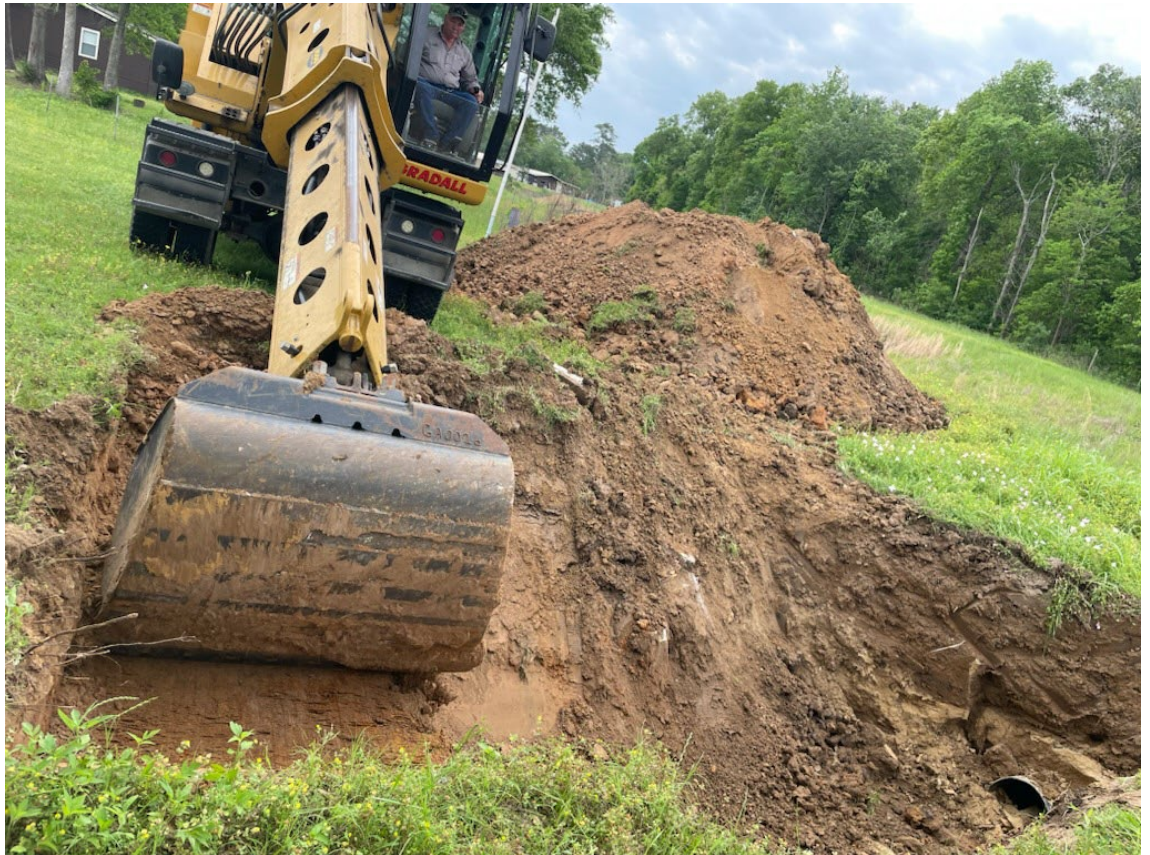
STORM SEWER REPAIR AT THE WEST END OF AVENUE B
