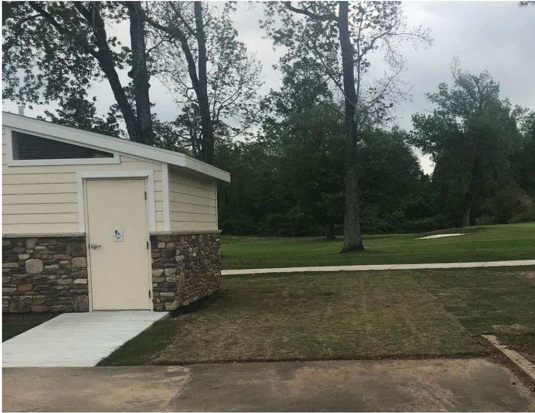
Sod laid around the new restroom
