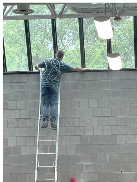
Installing foam gap filler to keep out debris
