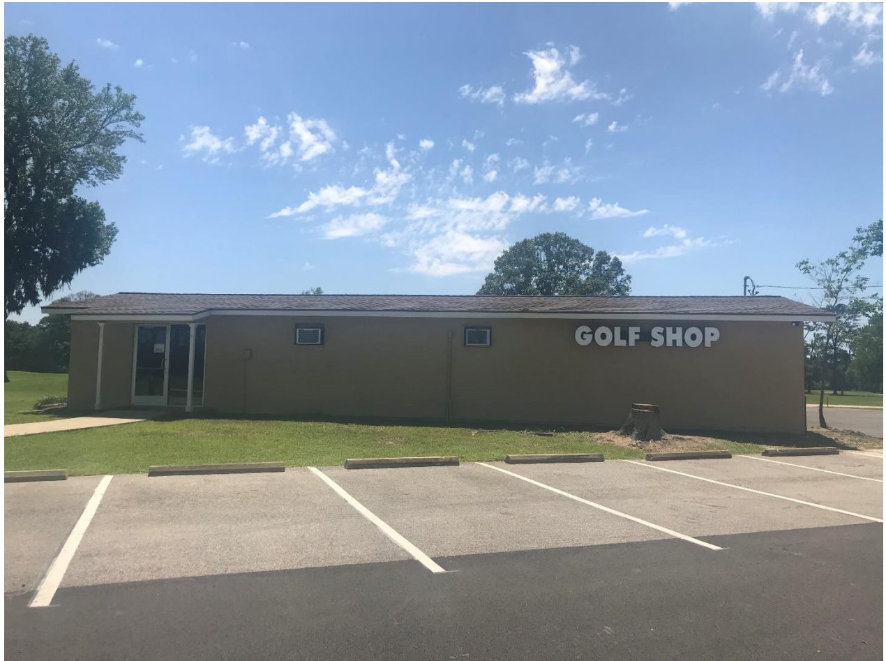
New sign installed on the golf shop
