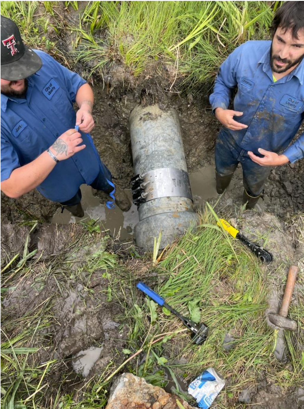
WATER LINE BREAK REPAIR– JOEL AND CHRISTIAN
