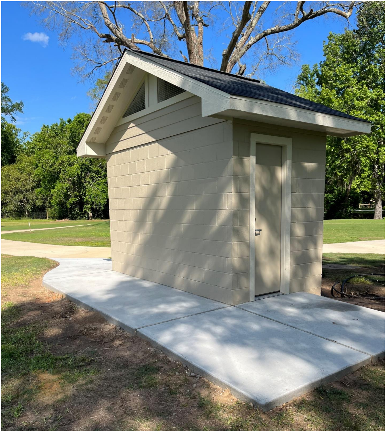
Restroom painted and new doors installed
