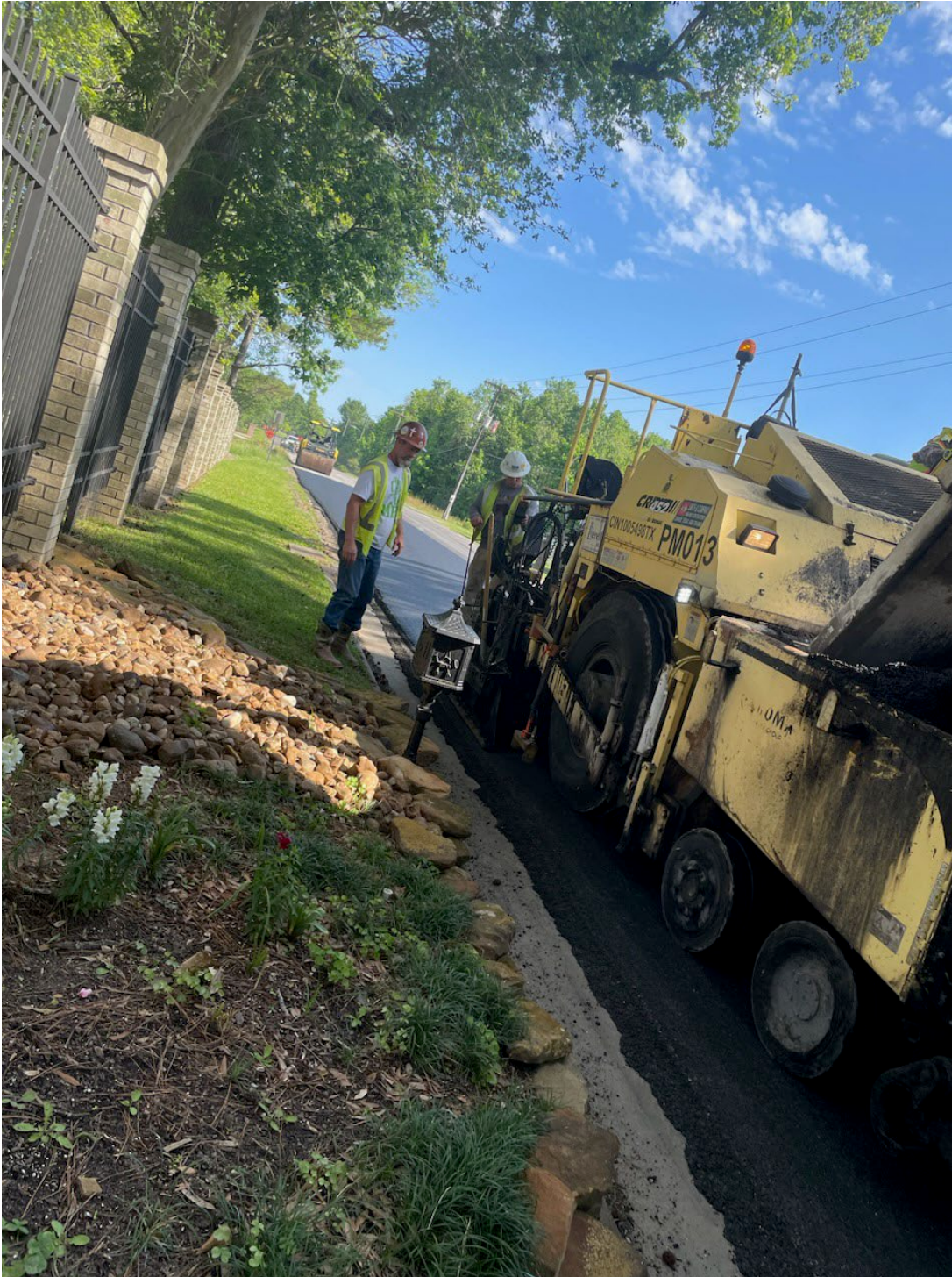
NORTH TRAVIS BETWEEN JEFFERSON AND THE TRAVIS PARK CROSSING 1.5" SURFACE
