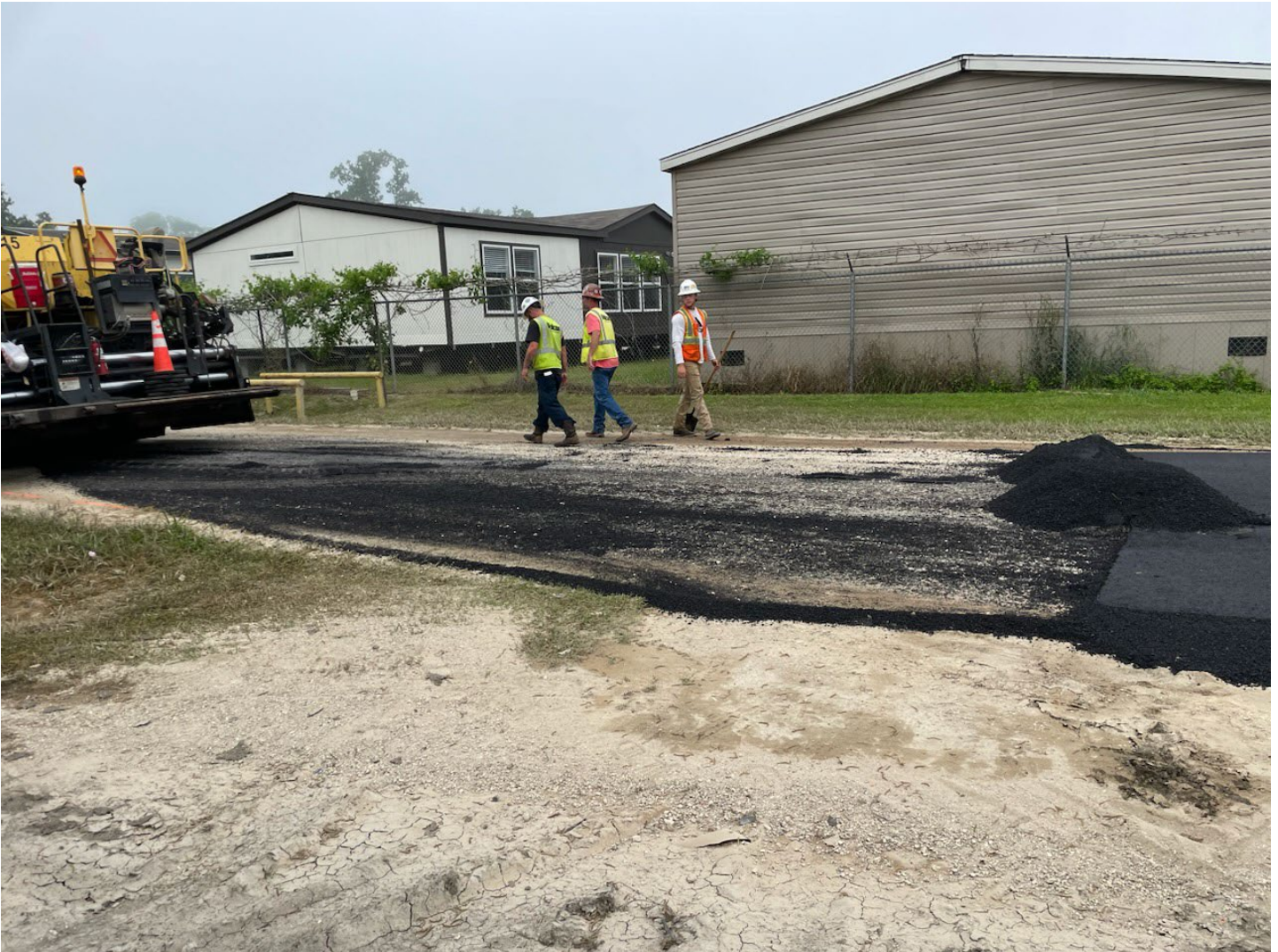
TENNESSEE ST. 2" ASPHALT SURFACE PLACEMENT
