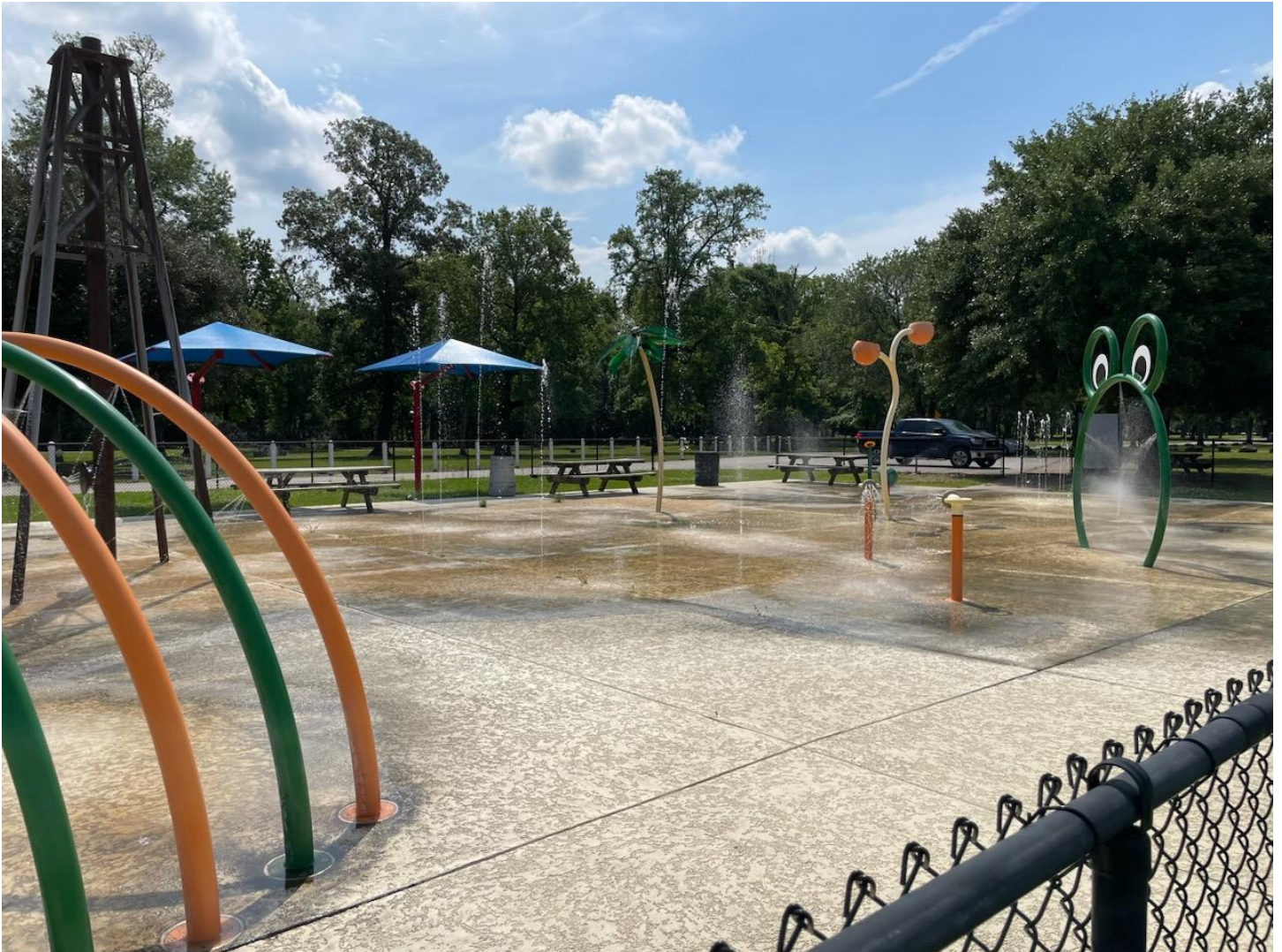
NEW CHEMICAL CONTROLLER FOR THE SPLASHPAD
