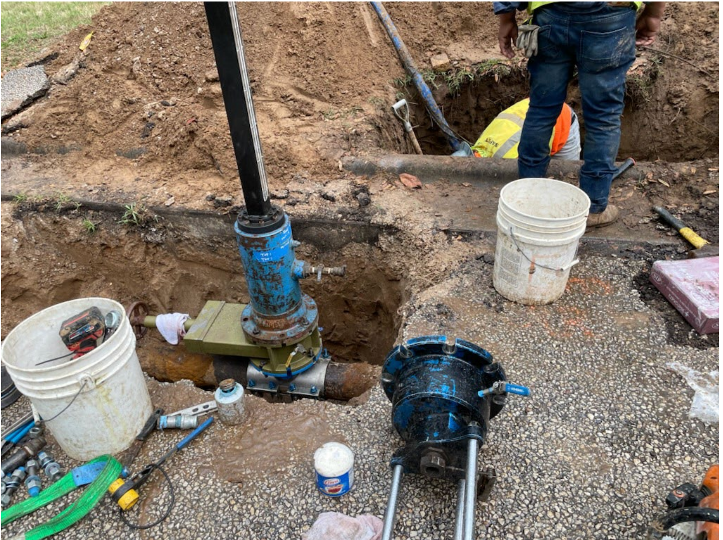
LINE STOP INSTALLED AT BOWIE AND TRINITY
