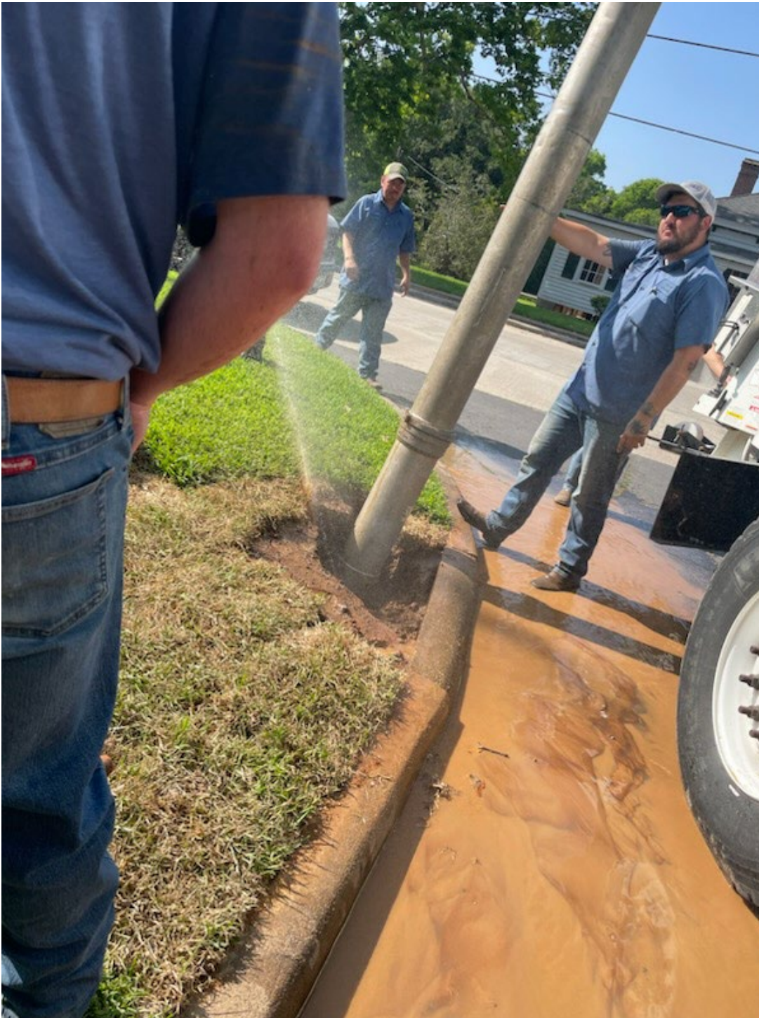
WATER LINE BREAK REPAIR– JOEL AND ROBERT ON GRAND AND SAN JACINTO
