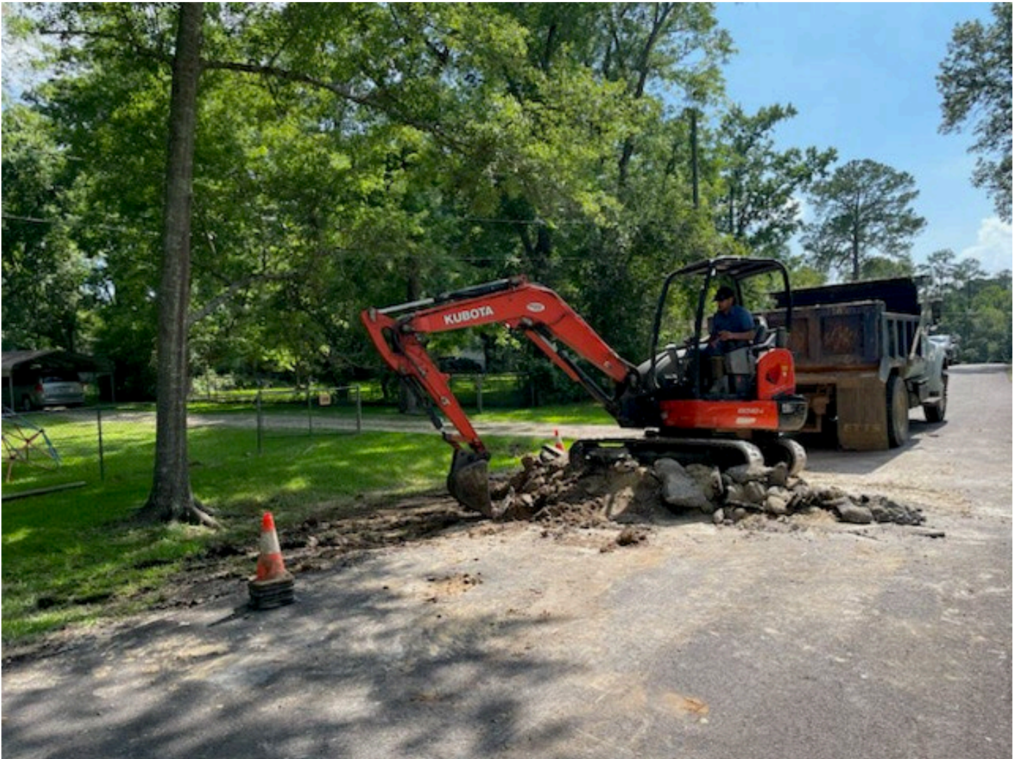
WATER LINE BREAK REPAIR– JOEL ON AVENUE G
