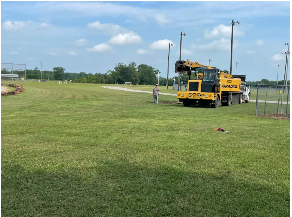
STREETS GRADING DITCH AT THE MUNICIPAL PARK.
