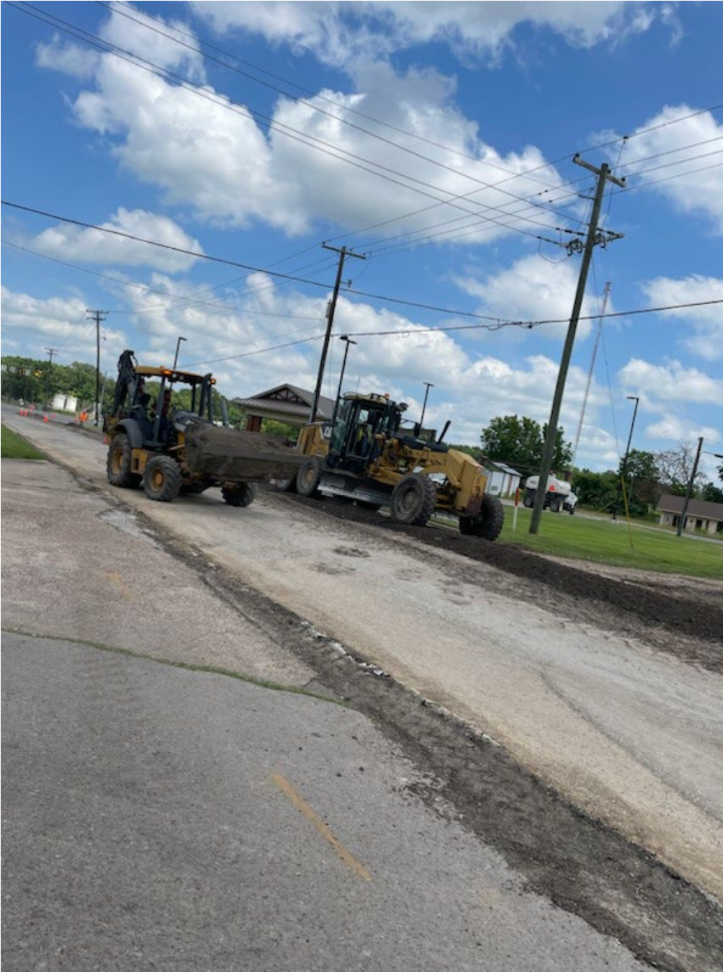
JEFFERSON (BETWEEN MAIN ST AND PANTHER LANE) STABILIZED BASE REHABILITATION
