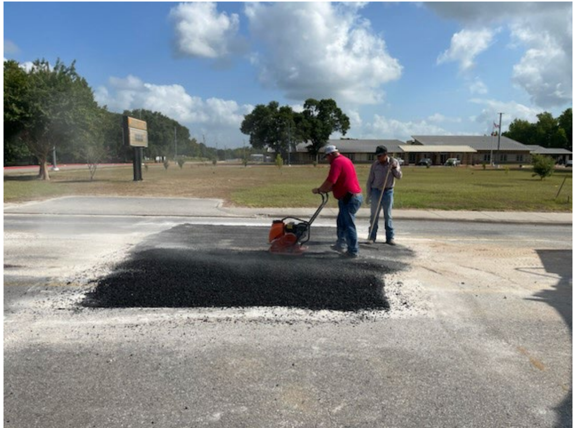
STREET REPAIR AT JEEFERSON AND TEXAS; VICTOR AND JAMES
