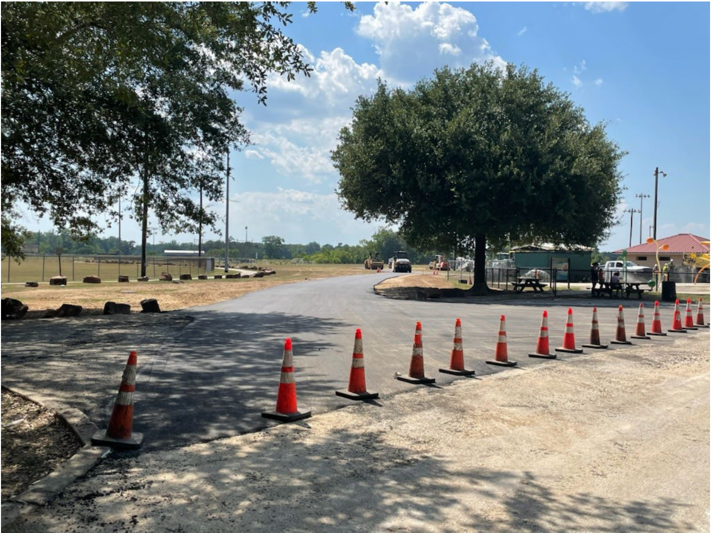
NEW ROAD TO THE CITY POND AT THE CITY PARK
