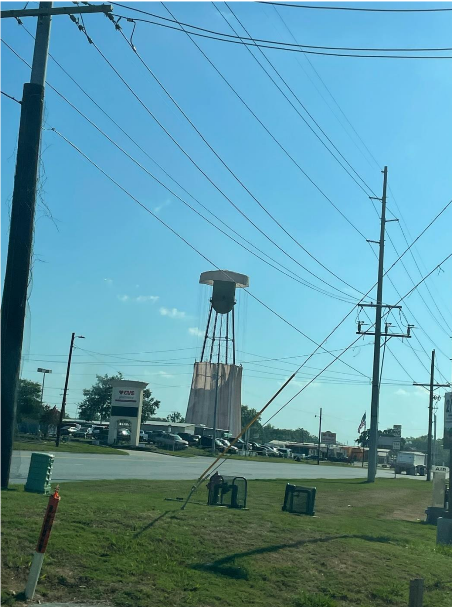
SAN JACINTO WATER TOWER CONTAINMENT INSTALLATION
