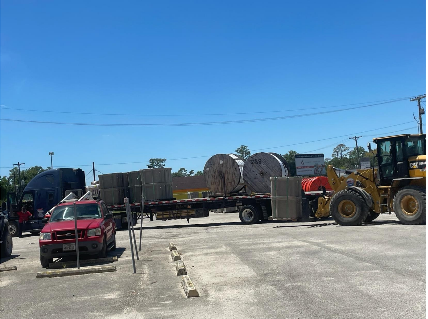
MATERIAL ARRIVING AT THE PUBLIC WORKS SERVICE CENTER FOR THE FIBER OPTIC PROJECT
