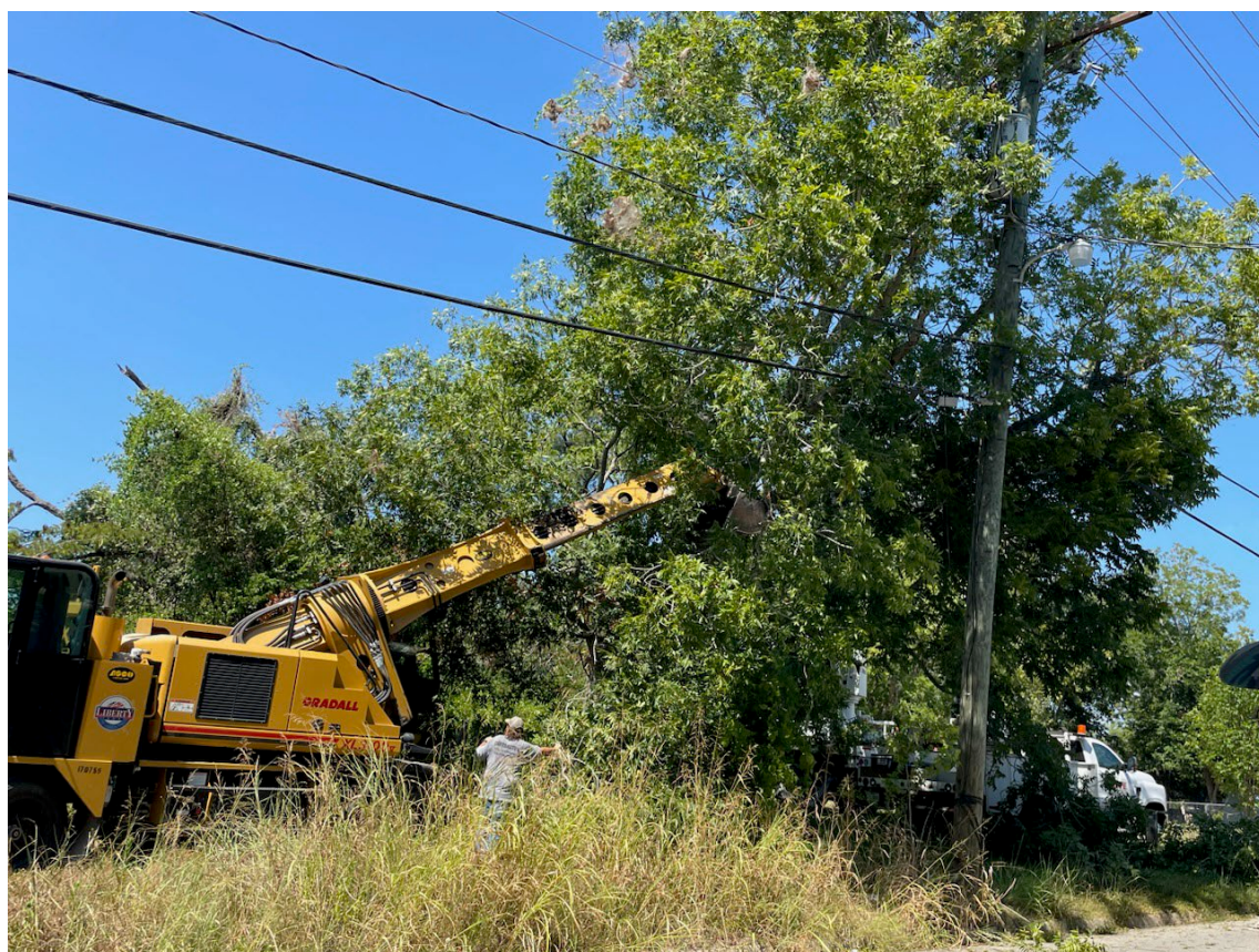
STREETS HELPING TEXAS ELITE REMOVE A TREE ON THE POWER POLE ON BEAUMONT.
