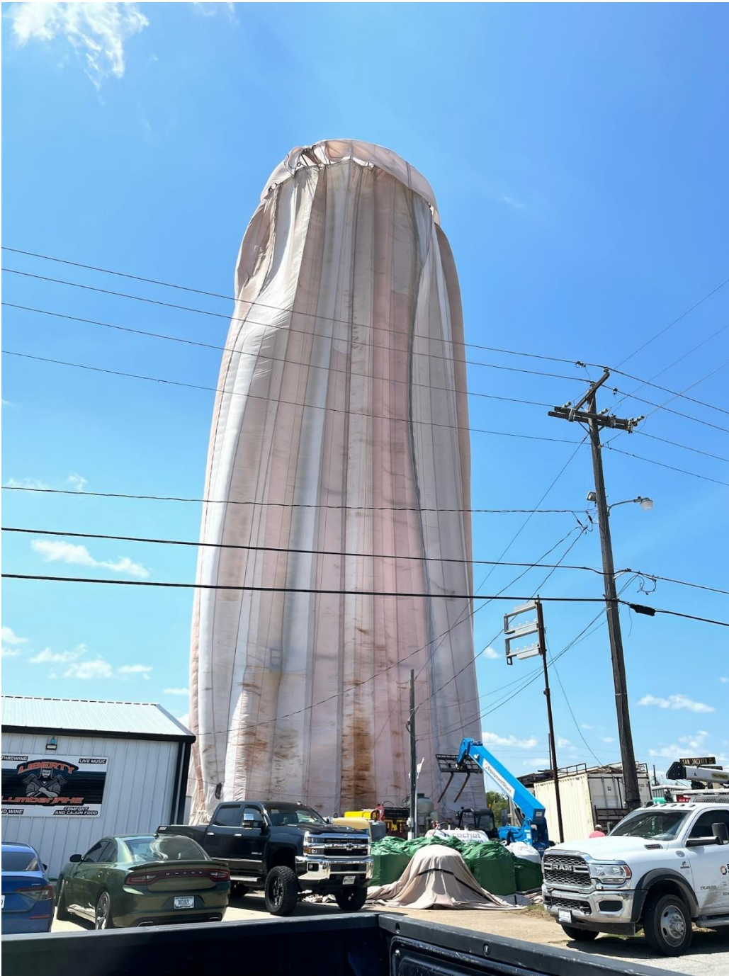
SAN JACINTO WATER TOWER REHABILITATION – SAND BLASTING
