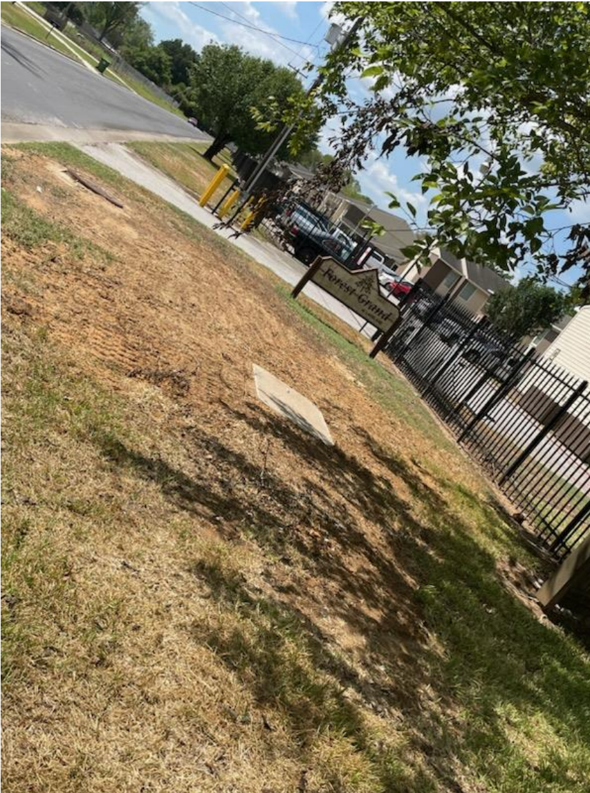
INSTALLED HAND HOLE ON LAKELAND NEAR GRAND
