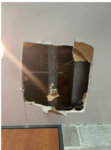
Before and after repairs from the fire pipe leak.
