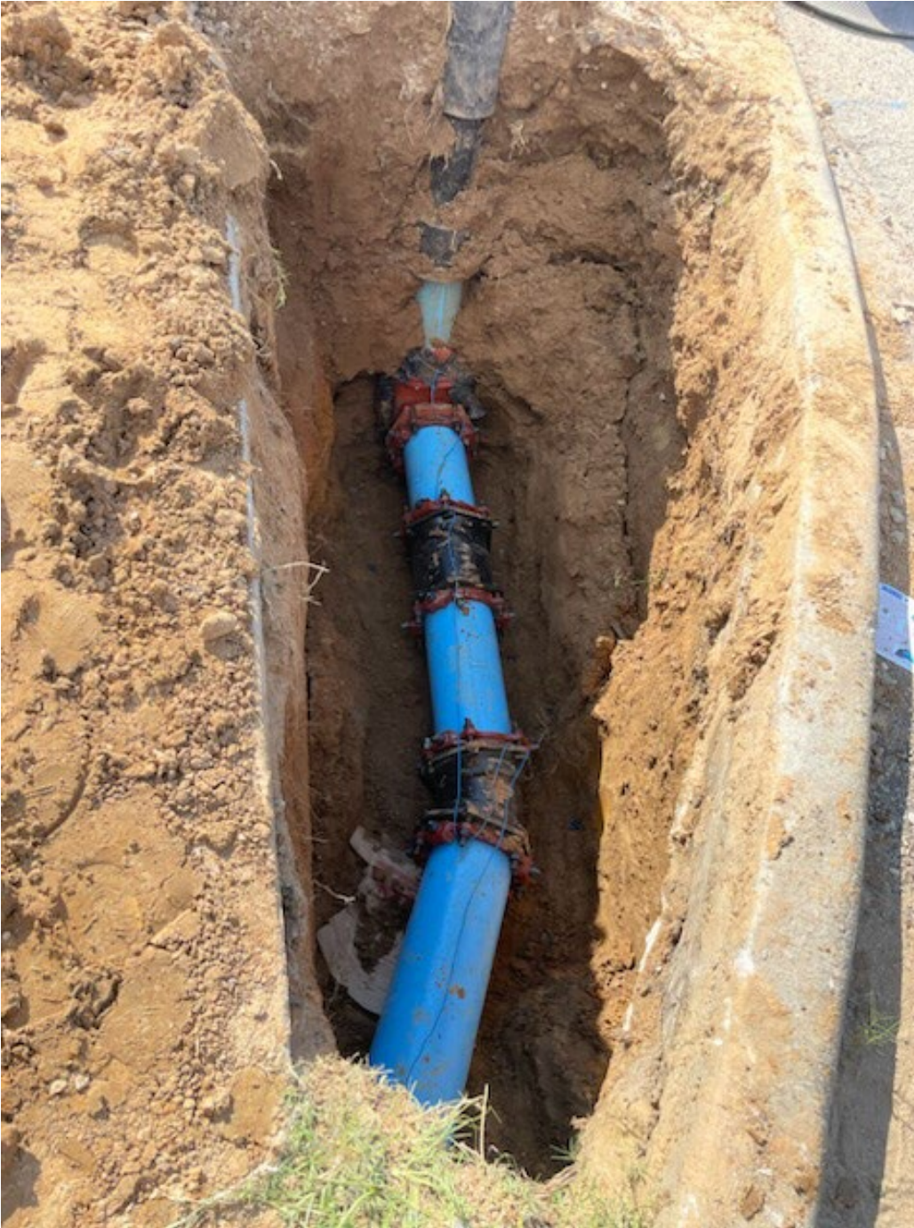
WATERLINE CONNECTION AT CROCKETT AND US 90
