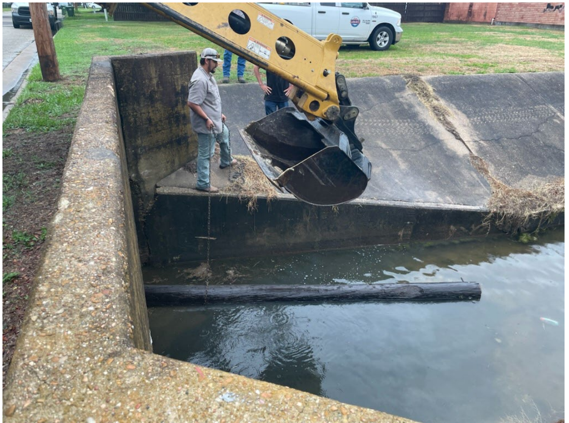
STREETS REMOVING POWER POLE IN MAIN B CHANNEL AT WOODS ST.
