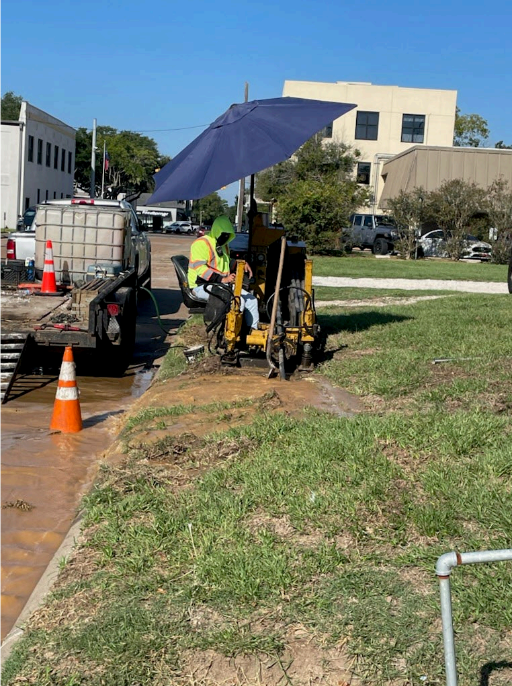
CONTRACTOR INSTALLING CONDUIT ON SAM HOUSTON ST
