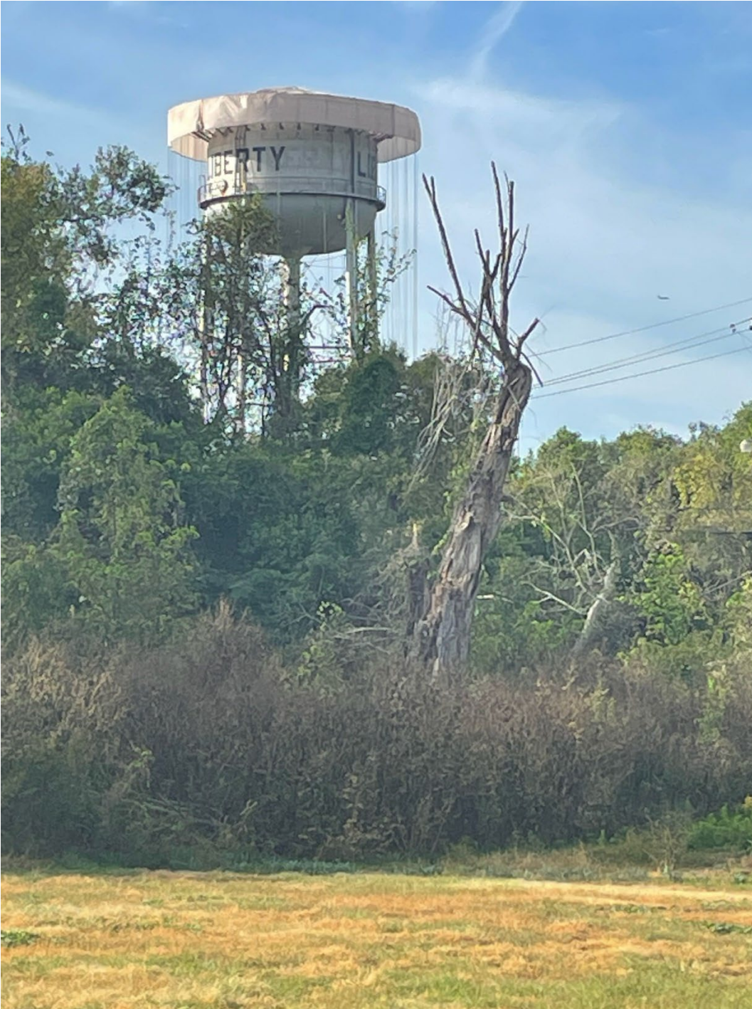
PALMER WATER TOWER CONTAINMENT INSTALLATION
