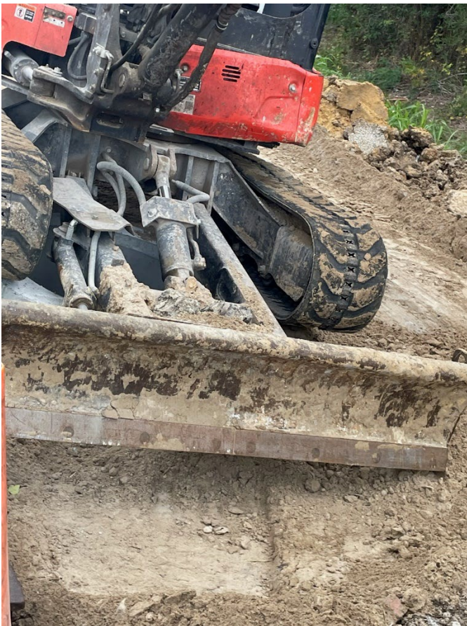
REPLACED MANHOLE ON TEXAS ST.
