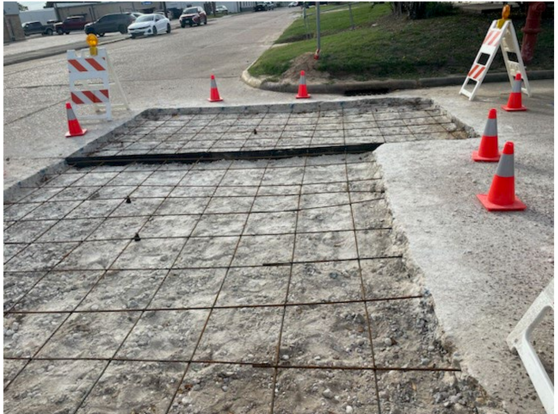
CONCRETE STREET REPAIR AT SAM HOUSTON AND FANNIN.
