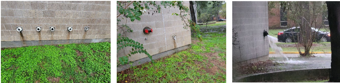
Outside drains October 3, 2023
