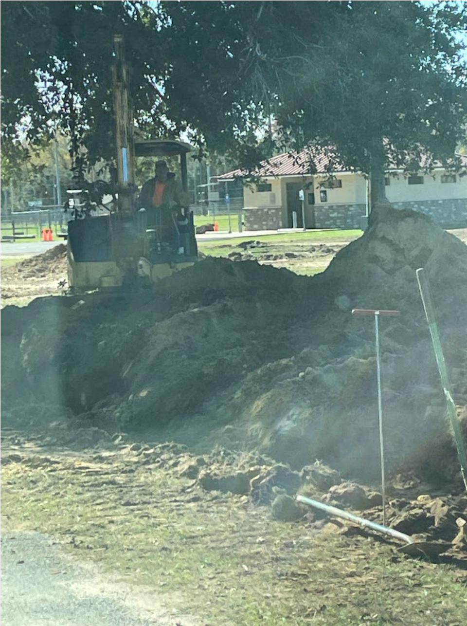
SANITARY SEWER LINE INSTALLATION AT CITY PARK
