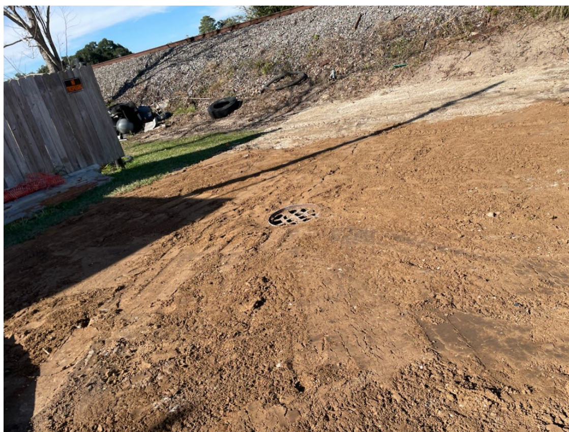
REPAIRED STORM SEWER CAVITY BEHIND 2223 MLK
