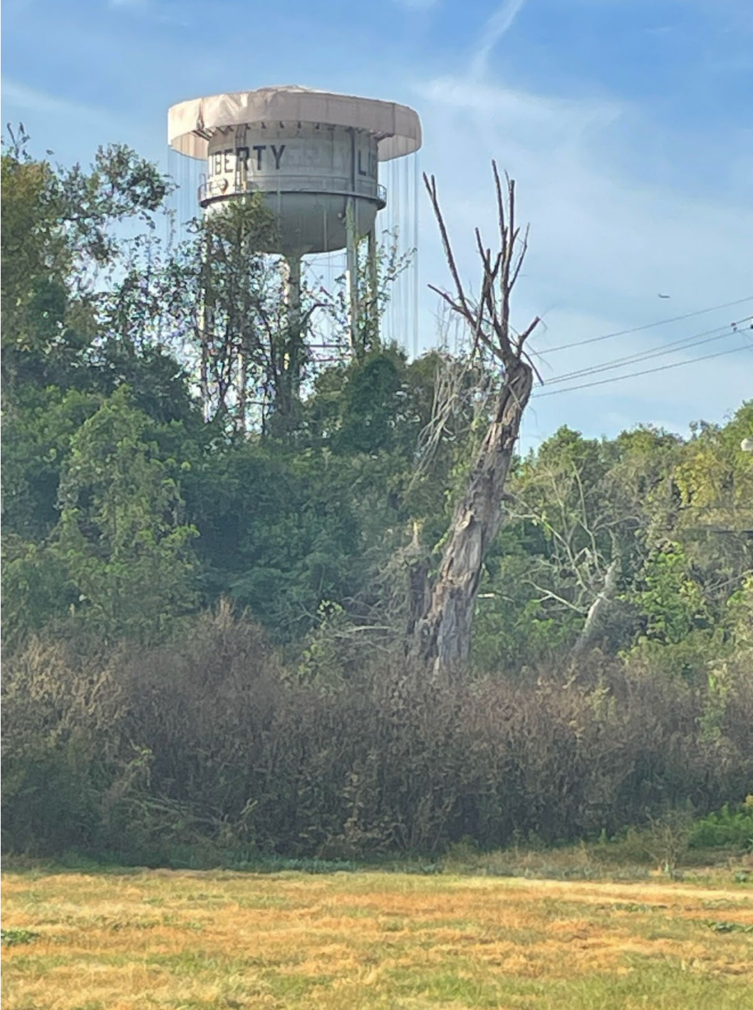
PALMER WATER TOWER CONTAINMENT INSTALLATION
