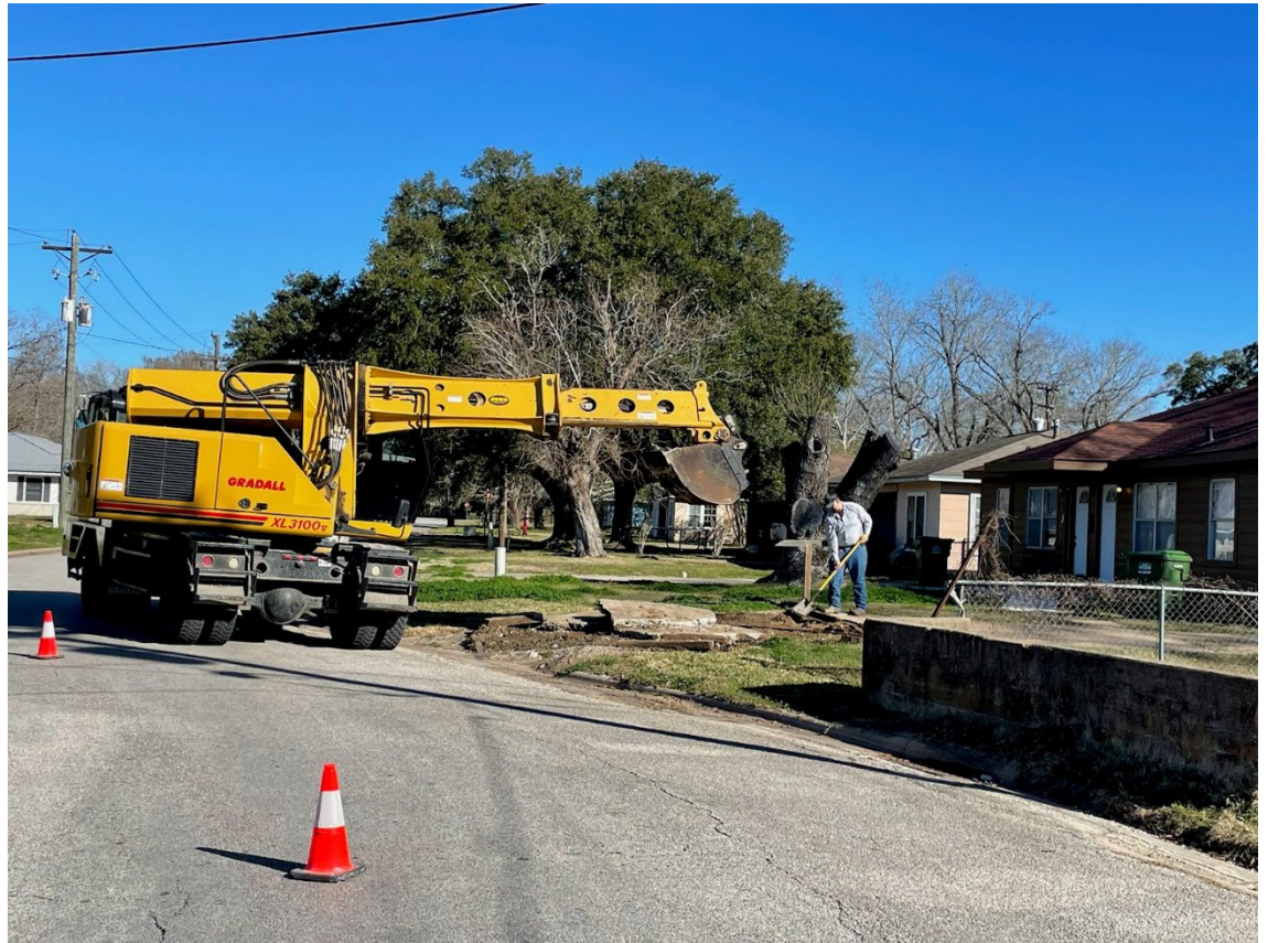
REPAIR WATER LEAK IN DRIVEWAY ON MILAM ST.
