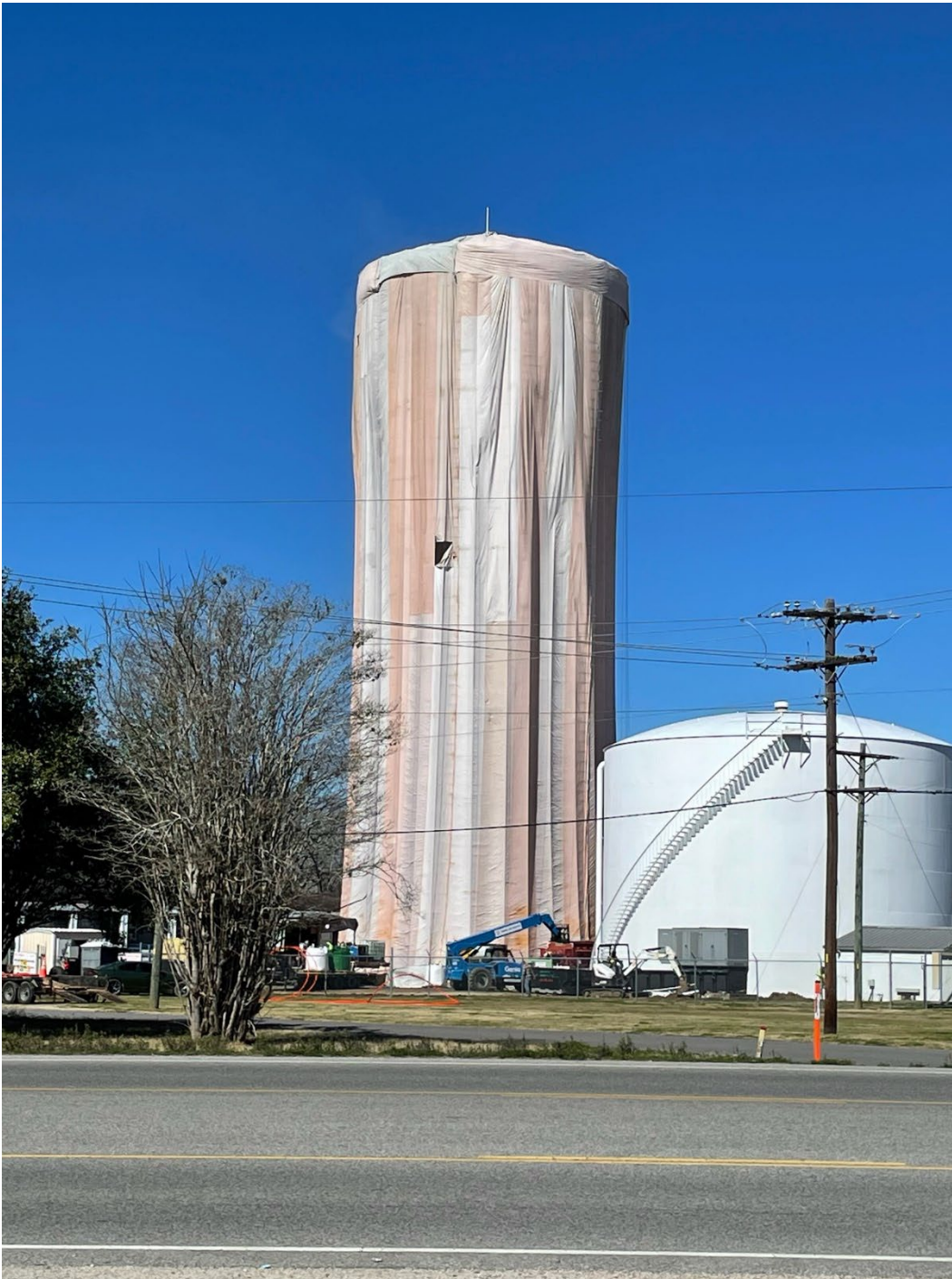
MONTA WATER TOWER CONTAINMENT AREA FOR SANDBLASTING AND PAINTING
