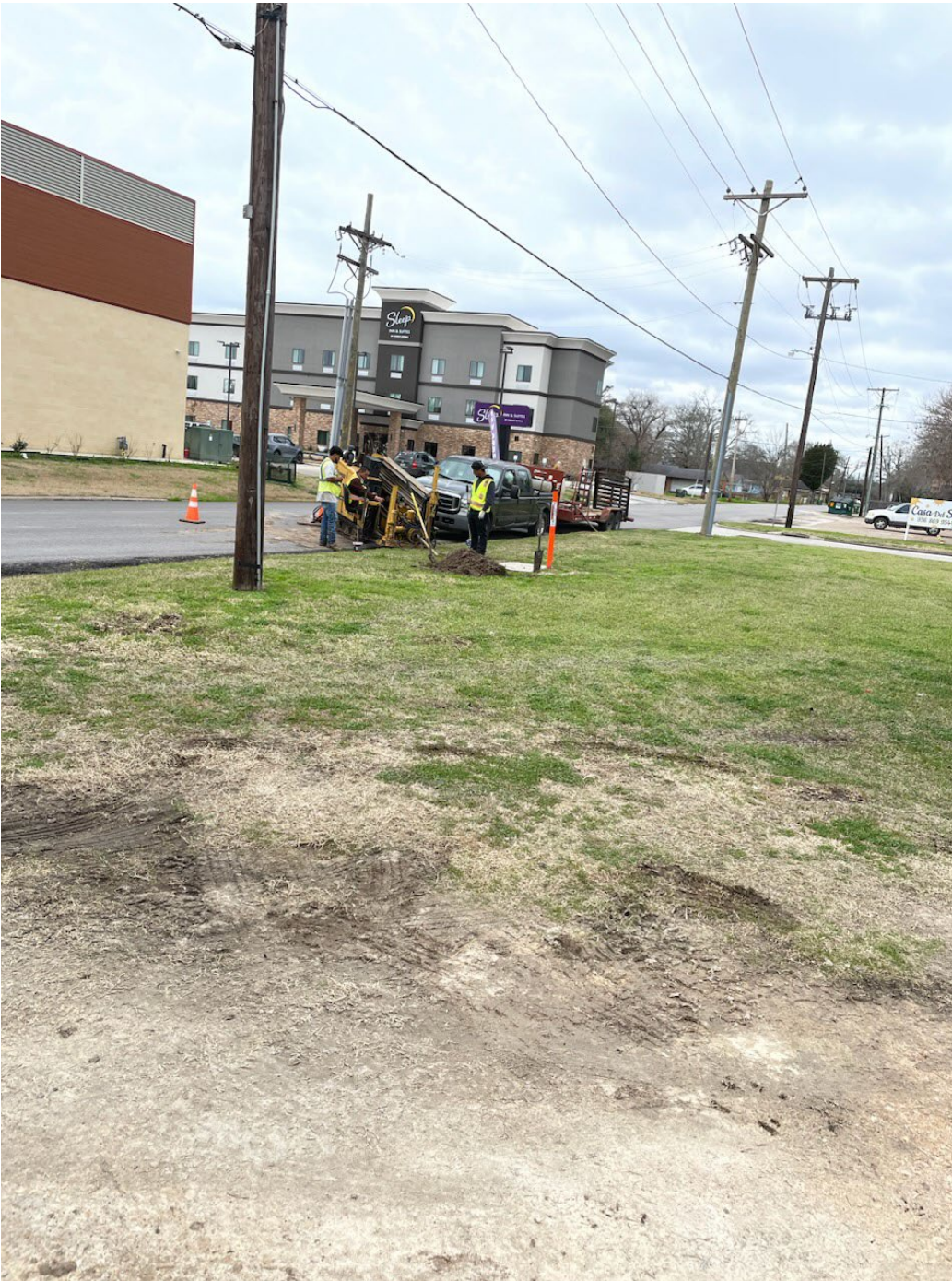
INSTALLATION OF CONDUIT AT MONTA WATER PLANT
