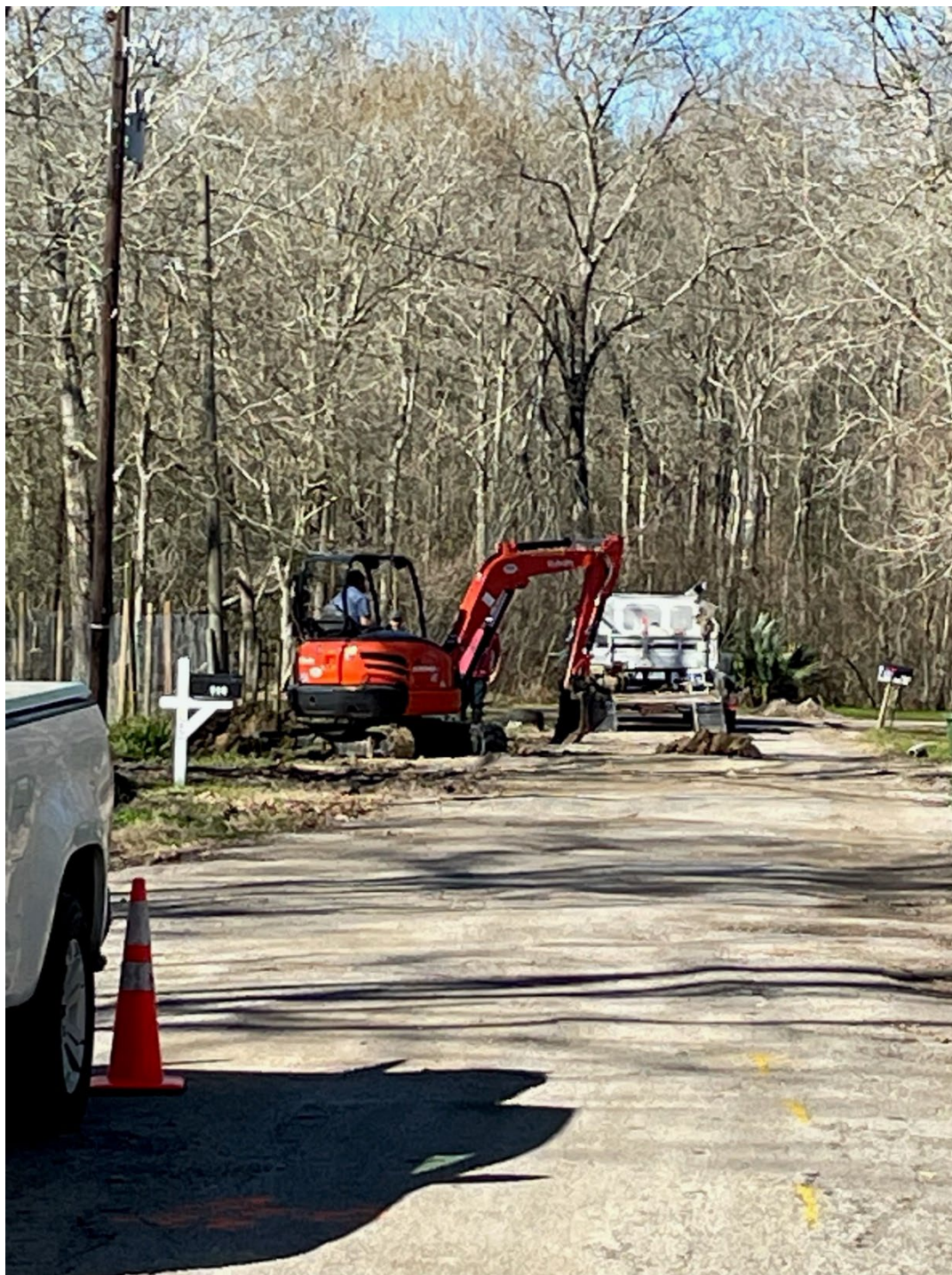
SANITARY SEWER TAP AT THE END OF GLENN ST.
