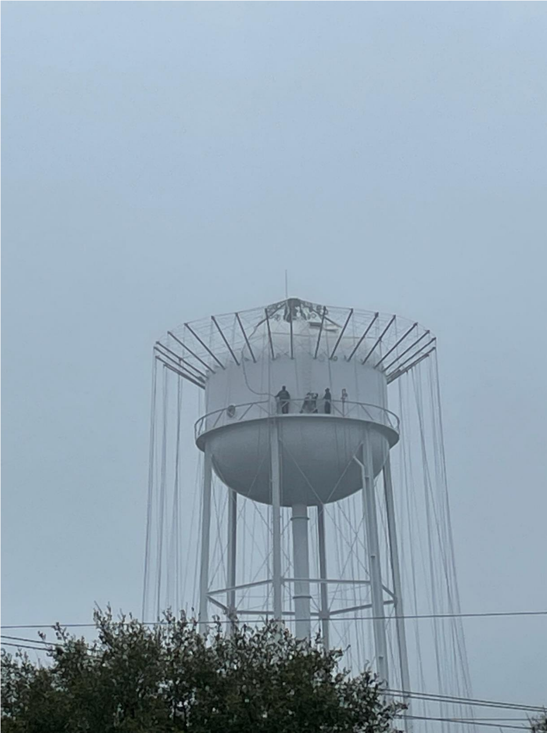
MONTA WATER TOWER PAINTING
