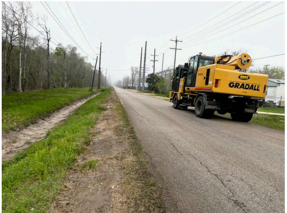
DITCH WORK ON BEAUMONT BETWEEN BYPASS AND INDEPENDENCE.
