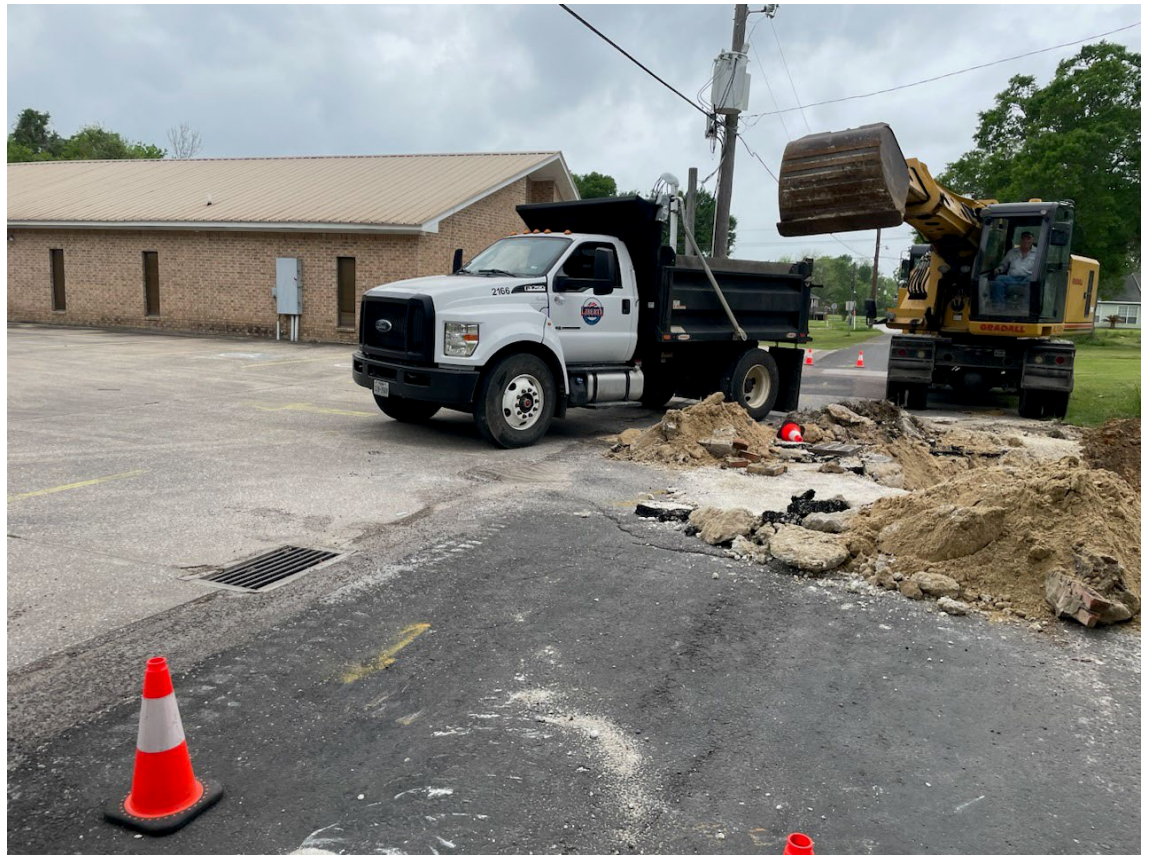
STORM SEWER REPAIR ON WASHINGTON ST.
