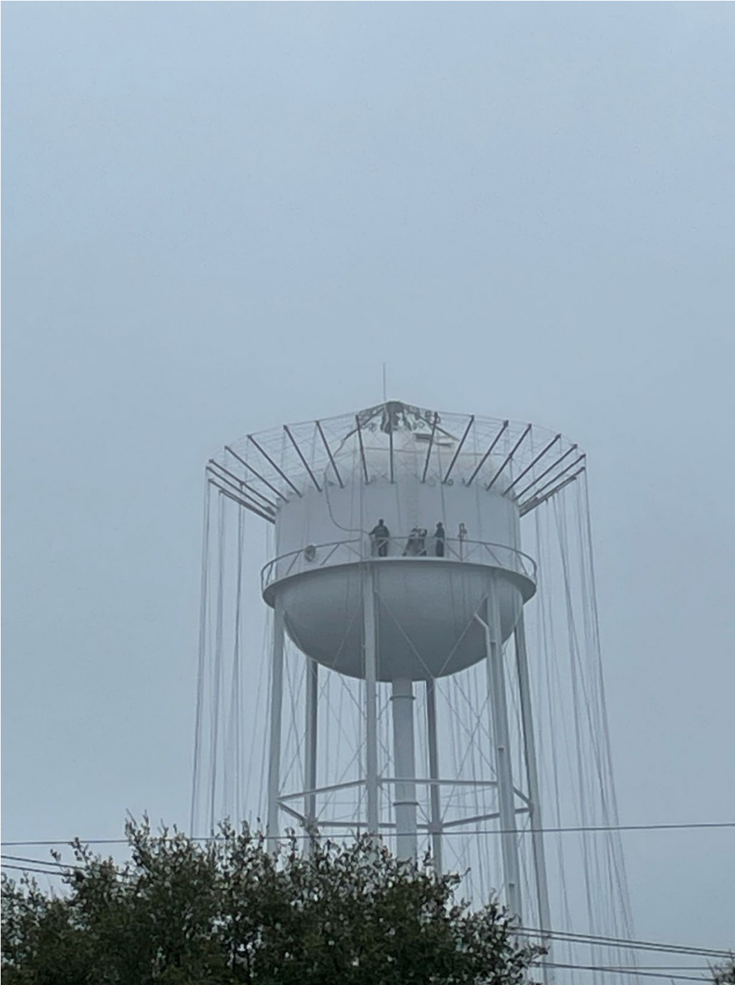
MONTA WATER TOWER PAINTING
