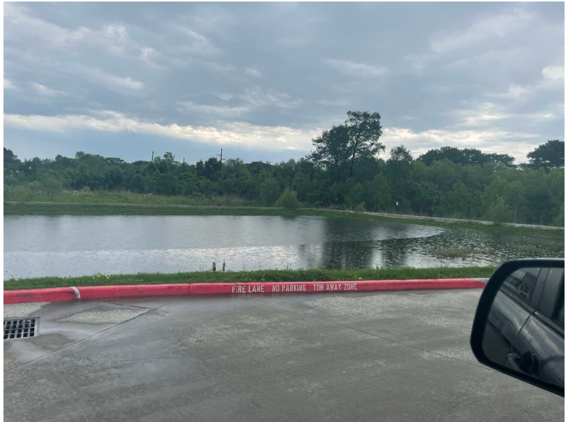
7-ELEVEN DETENTION POND (FM 2684 AND US 90)
