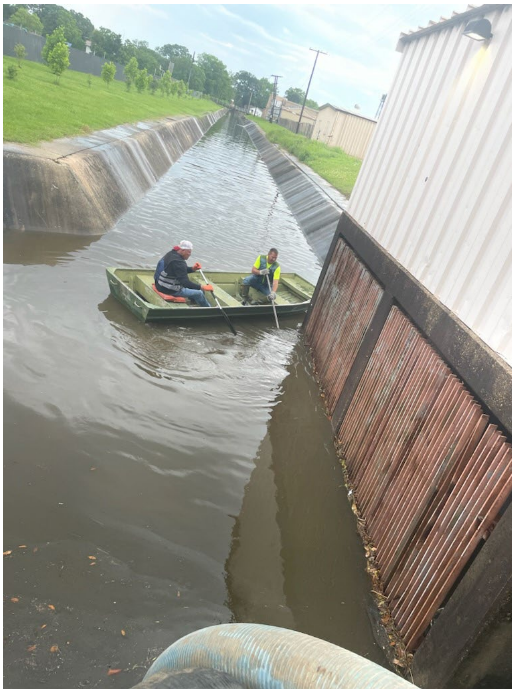
MAIN B STREETS KEEPING PUMP HOUSE GRATES FREE FROM DEBRIS
