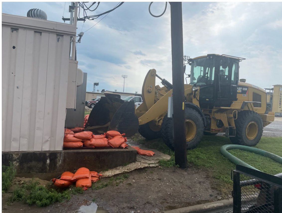
MAIN B PUMP HOUSE
