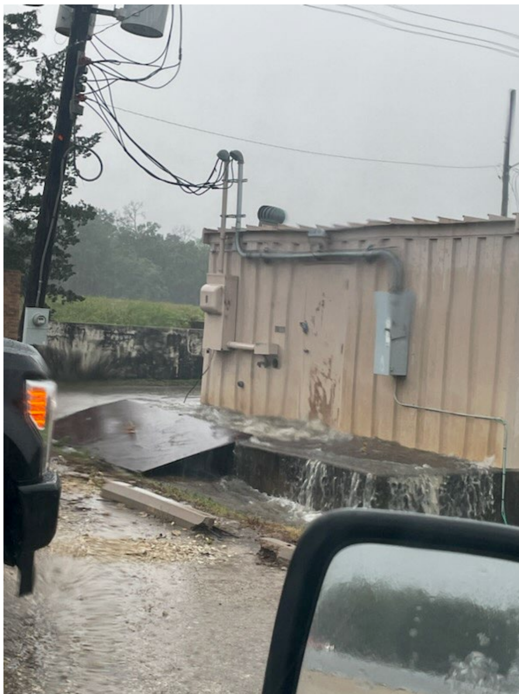
MAIN B PUMP HOUSE
