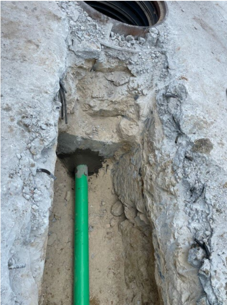
Sanitary sewer tap into a manhole
