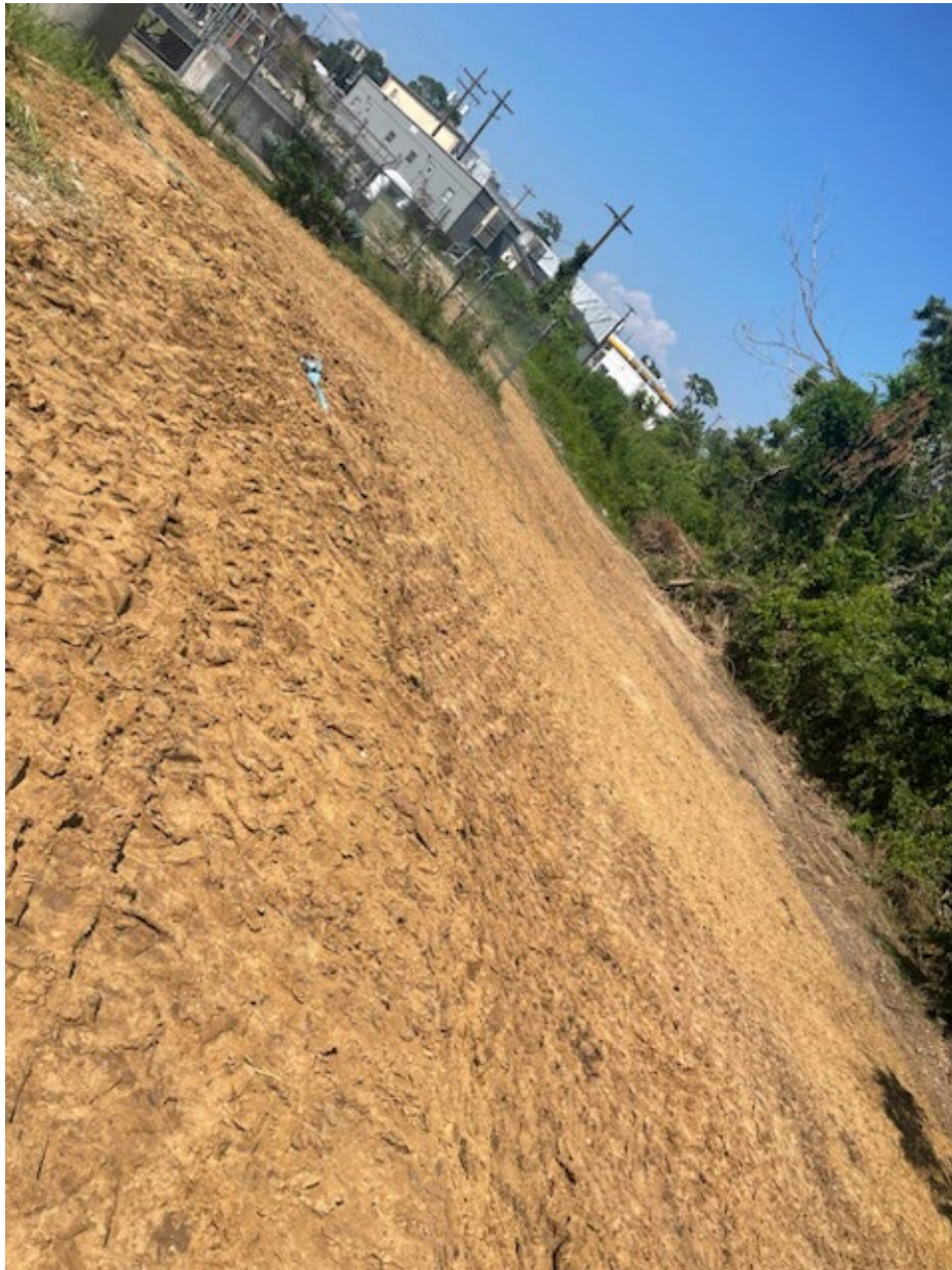
Dirt work at the end of Bowie St.
