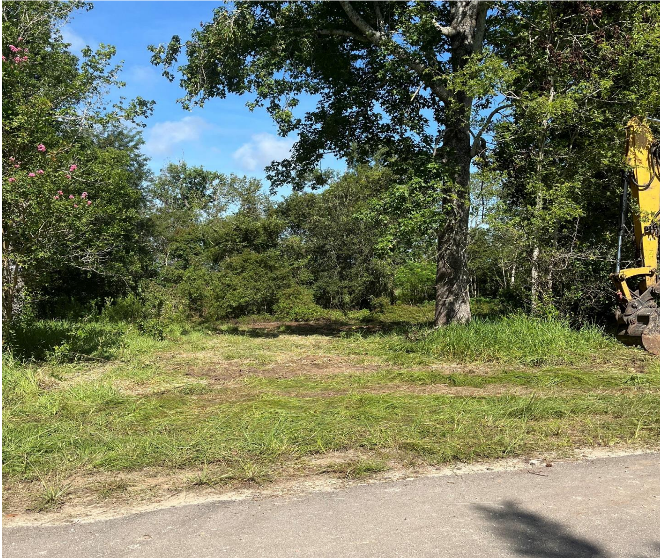
Completed demolition of 3805 Oilfield
