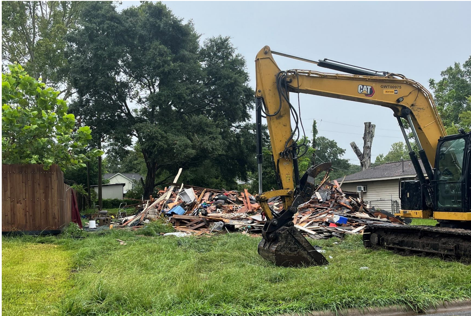
Completed demolition of 2612 Newman
