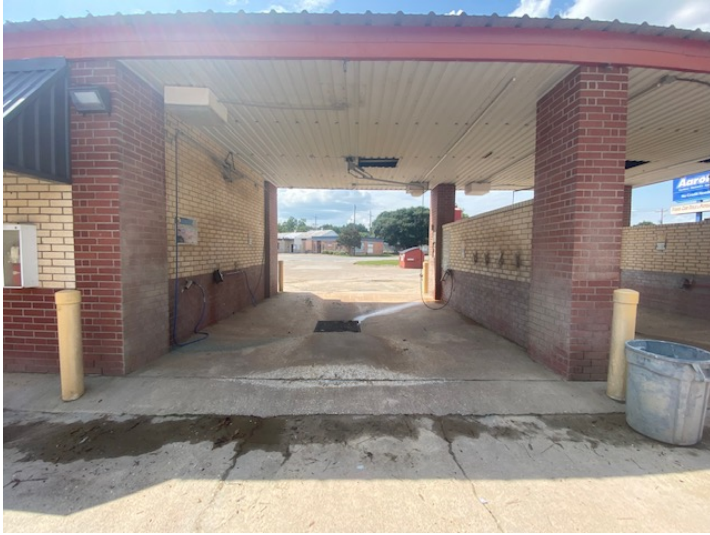
Current interior roof of wash bay.
