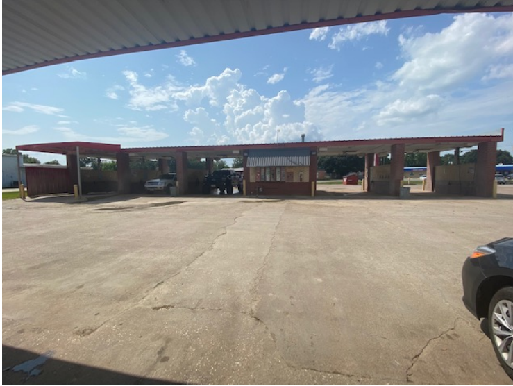
Current flat roof with canvas awning covering the Automatic Bay exit
