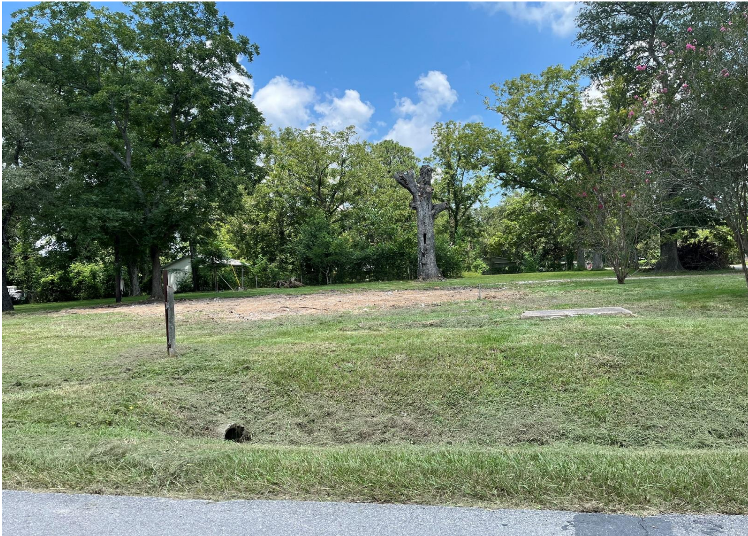
Completed demolition at 101 Elm
