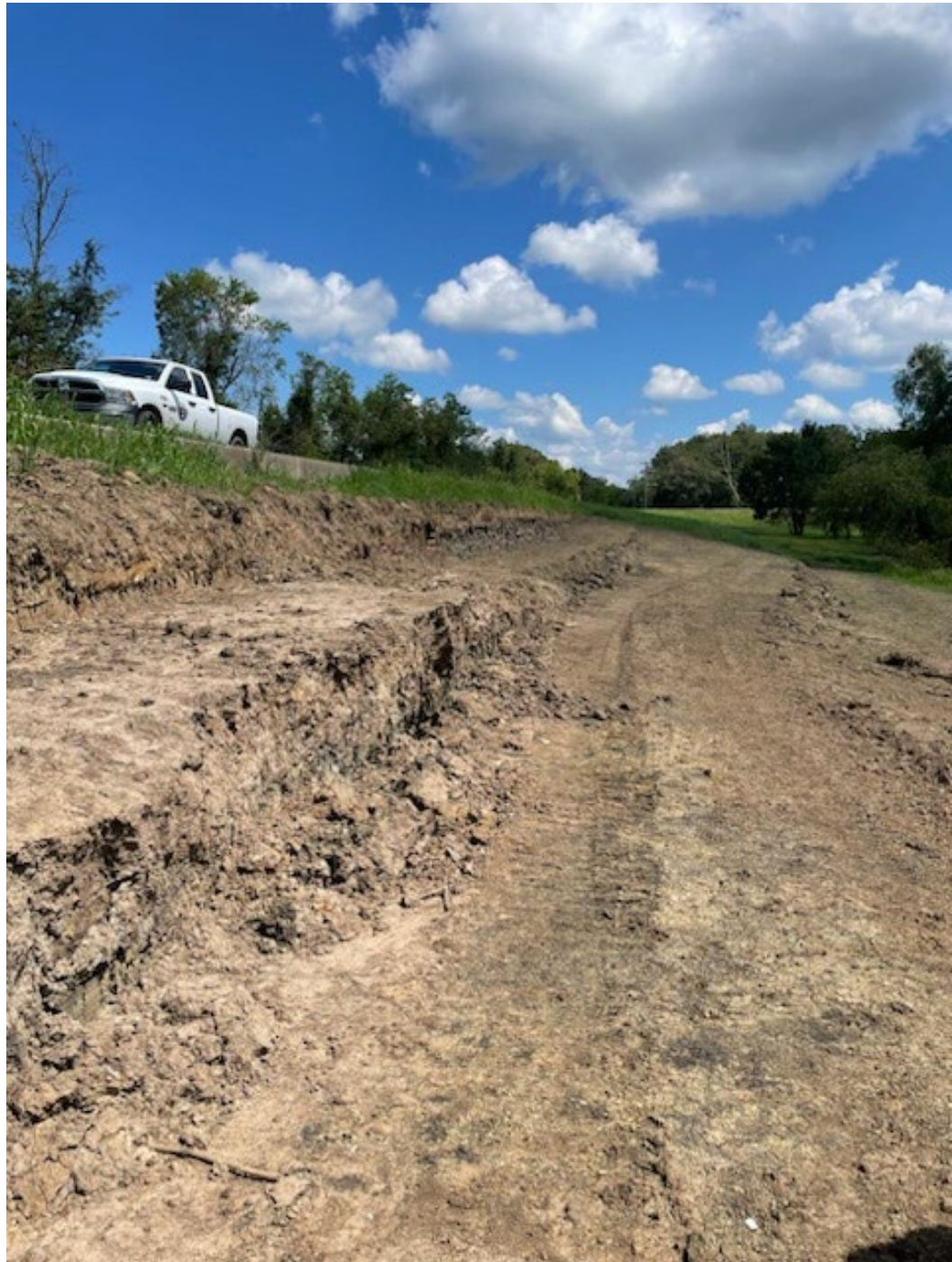
Main A Levee being repaired – Stair Step Method
