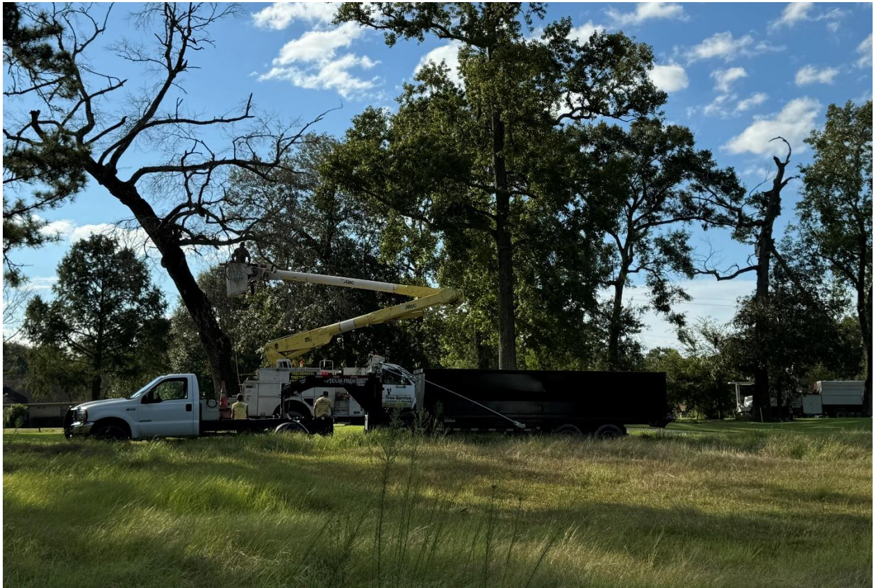
Contractors cutting down trees at the golf course
