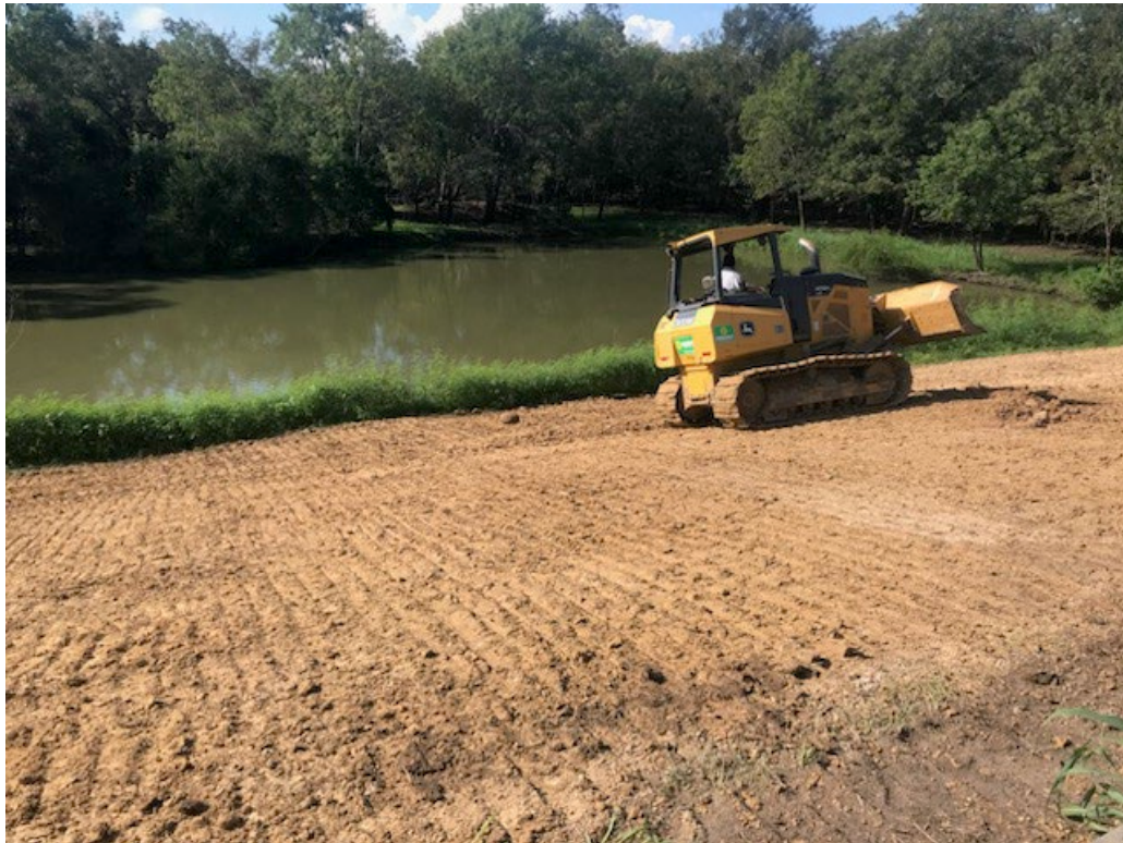
Main A levee repair completed with City Street Staff
