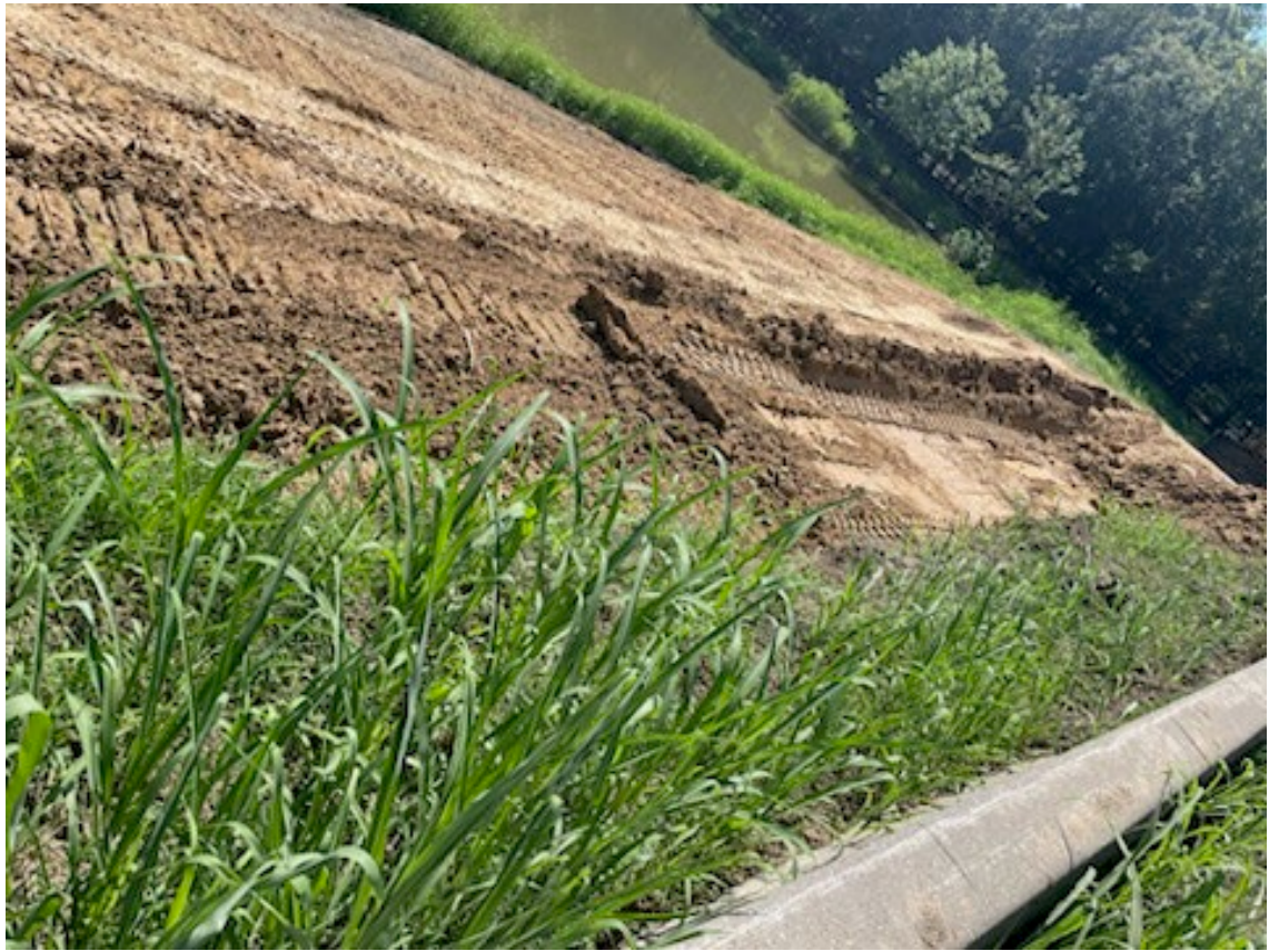
Main A levee slope repair
