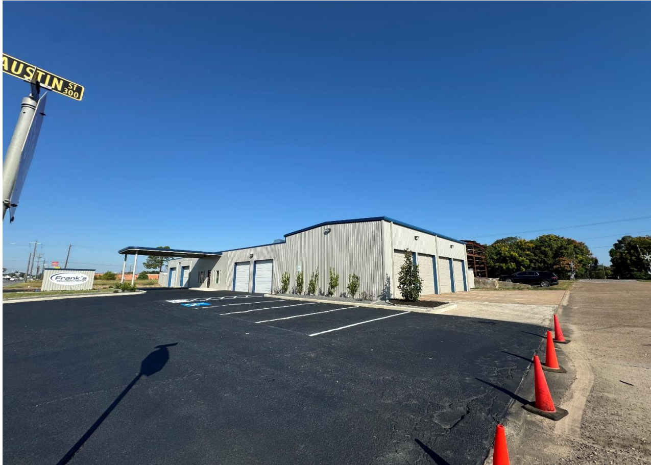
Frank's Collision Repair after renovation
