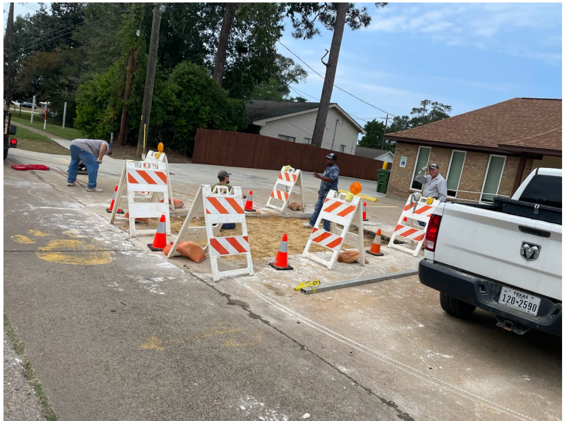
STREETS REPAIRING STREET CUT ON GRAND ST.
