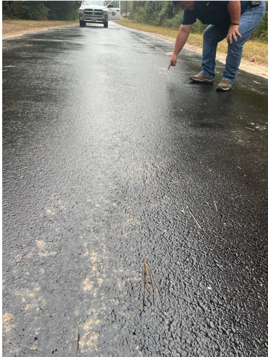
JAMES REDDING INSPECTING REHABILITATED STREET (ABLE)
