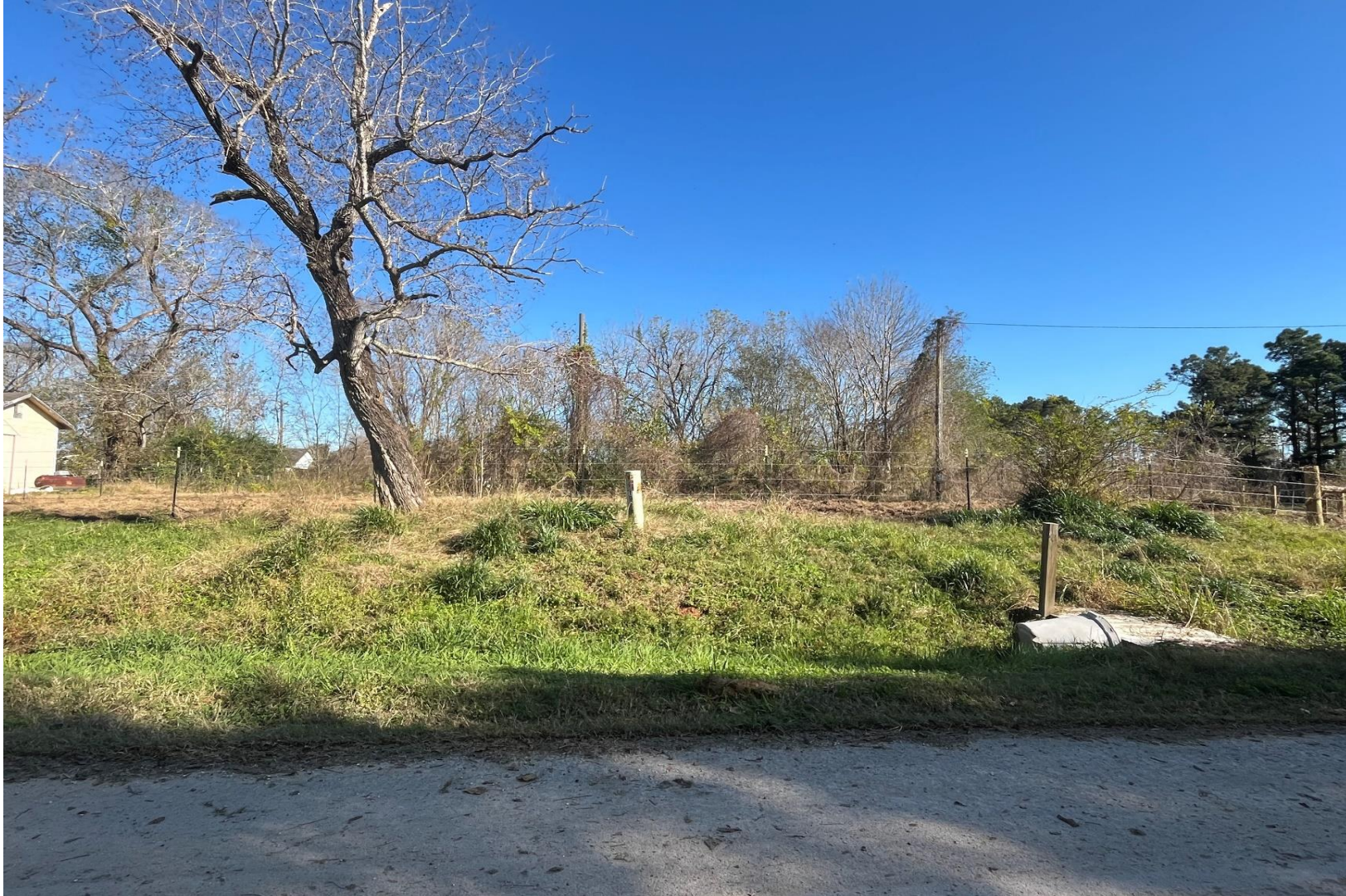
Completed demolition of 3812 Oilfield Road
