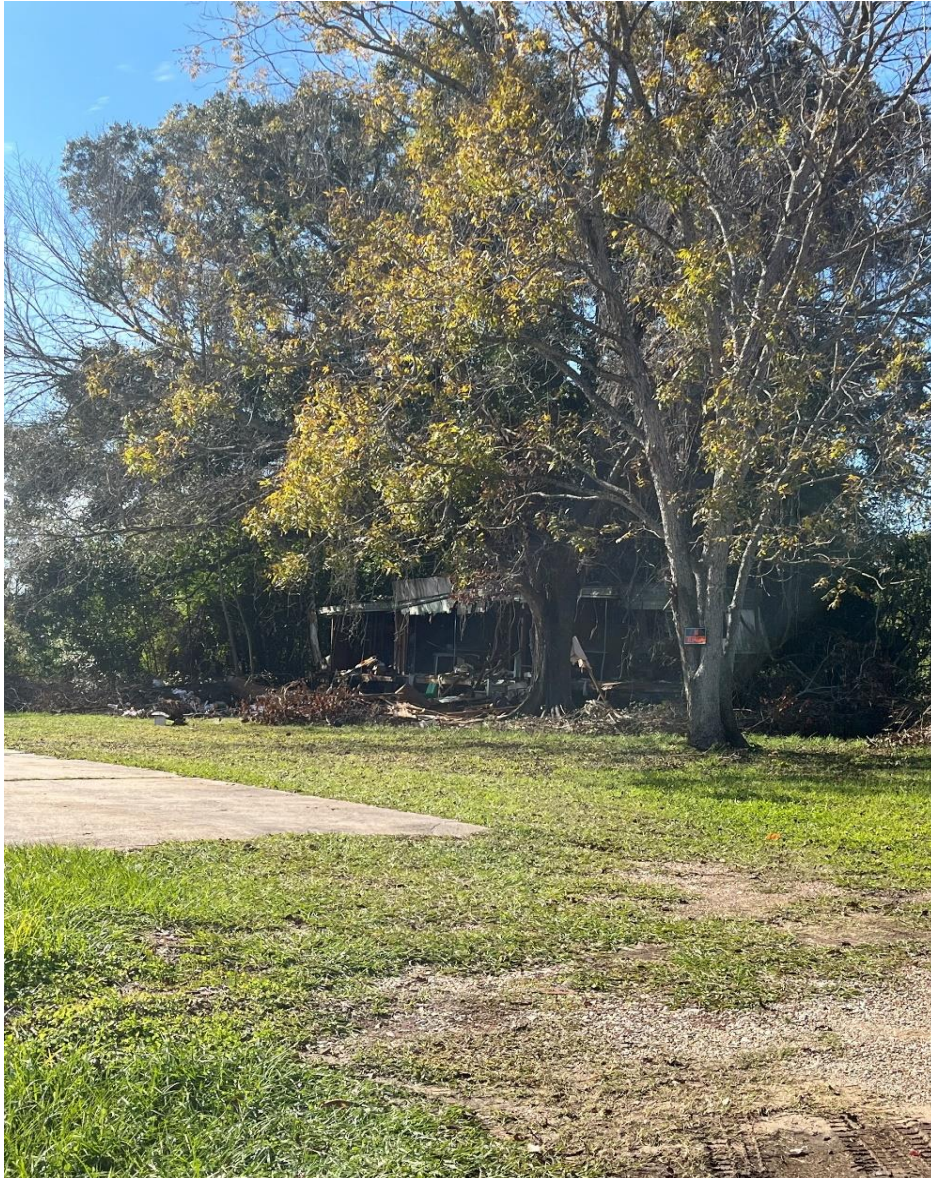
Partial demolition of 708 Lamar
