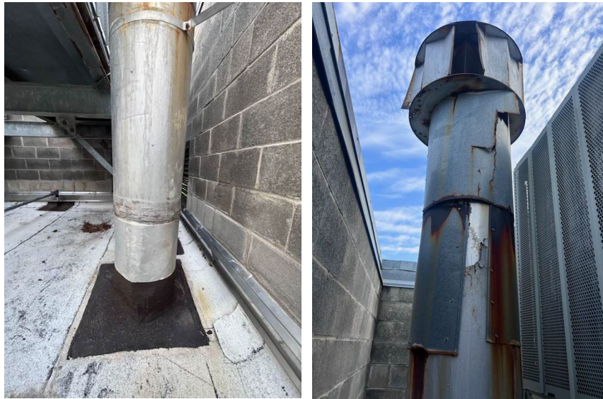
Old Boiler Pipe Flue and Cover
