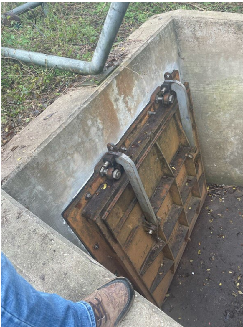
STREETS CONTRACTOR REPAIRED FLAP GATE AT CARTER ST
