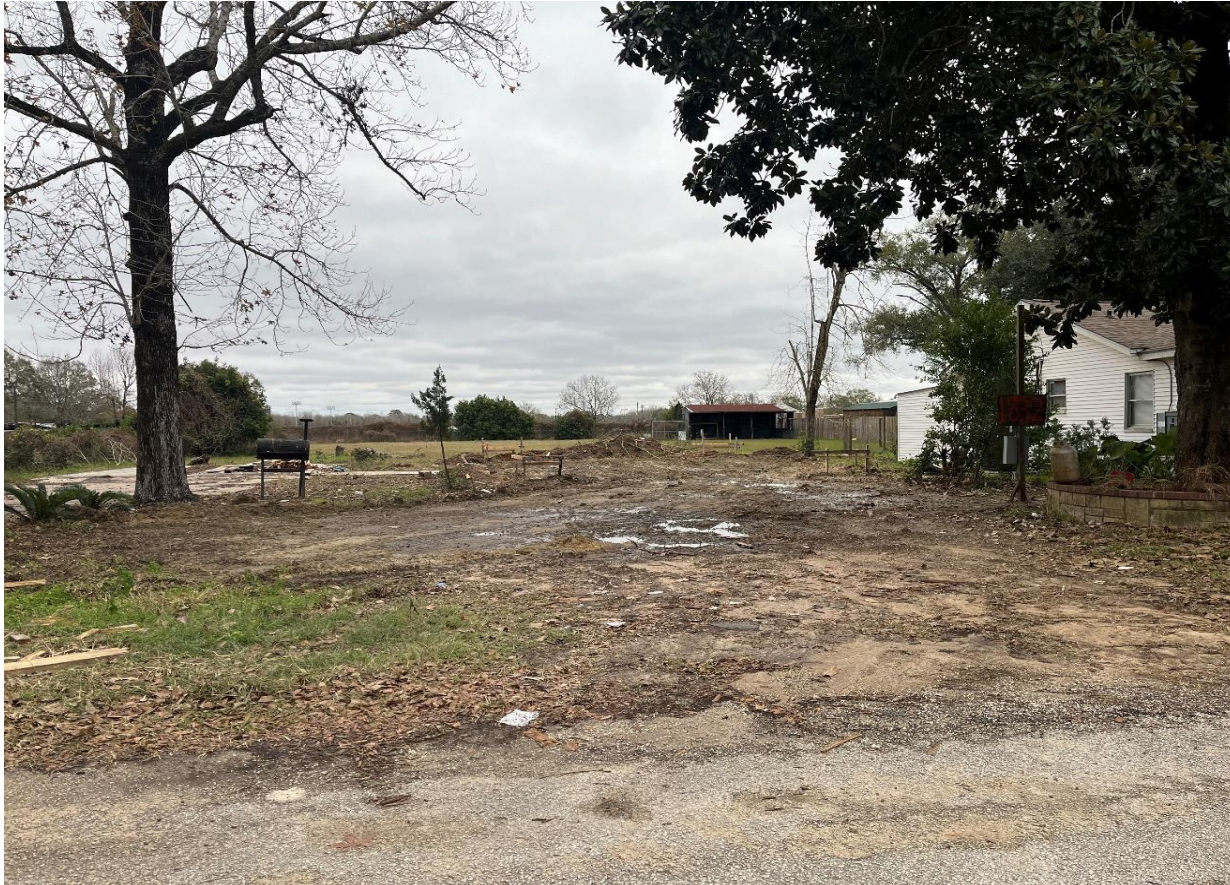
Voluntary demolition at 1832 Reese
