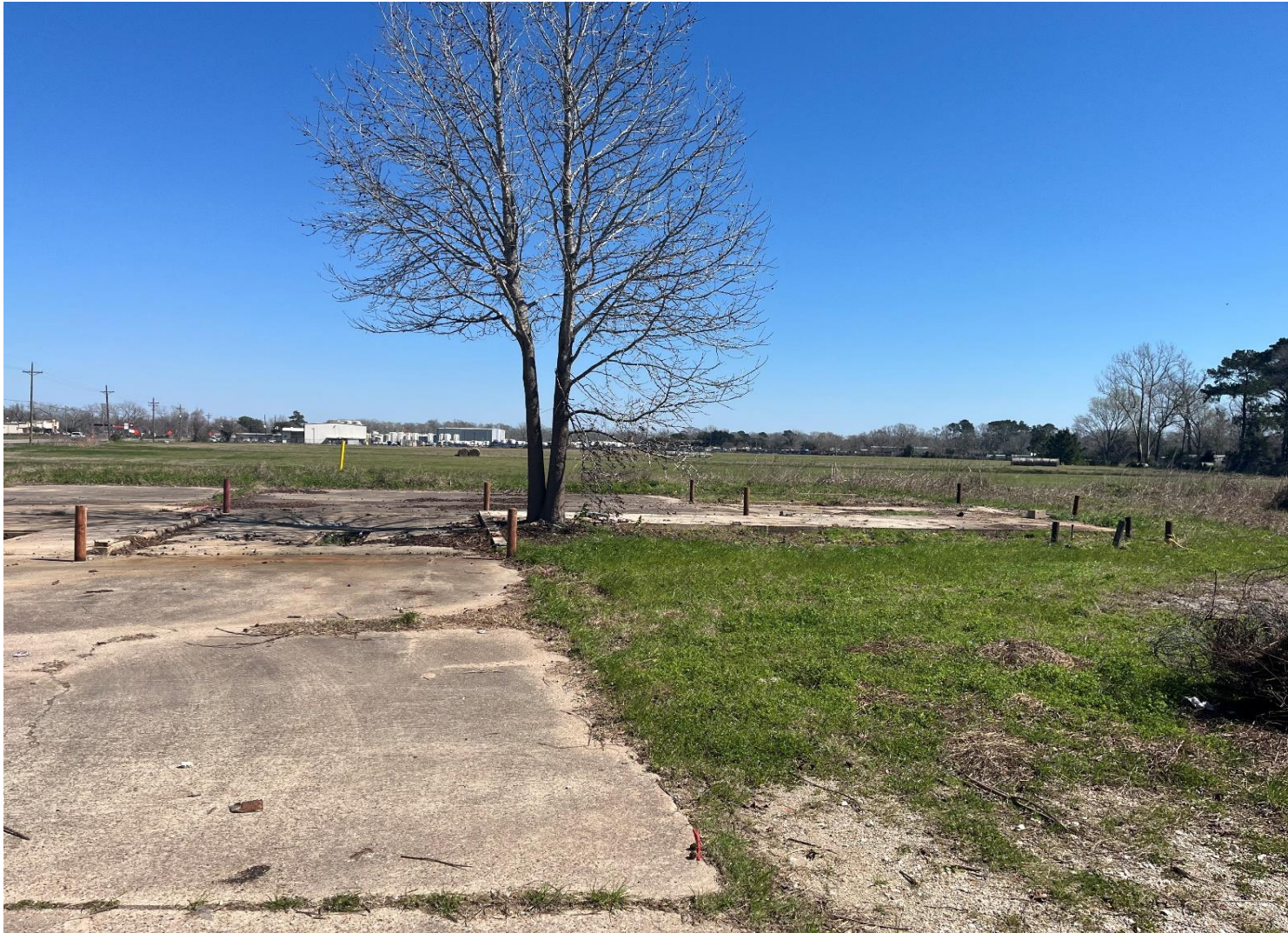
Partial demolition at 4310 N Main
