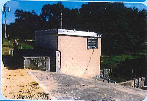
September 2015 – March 2016: Condition Assessment for Pump Stations A and B
