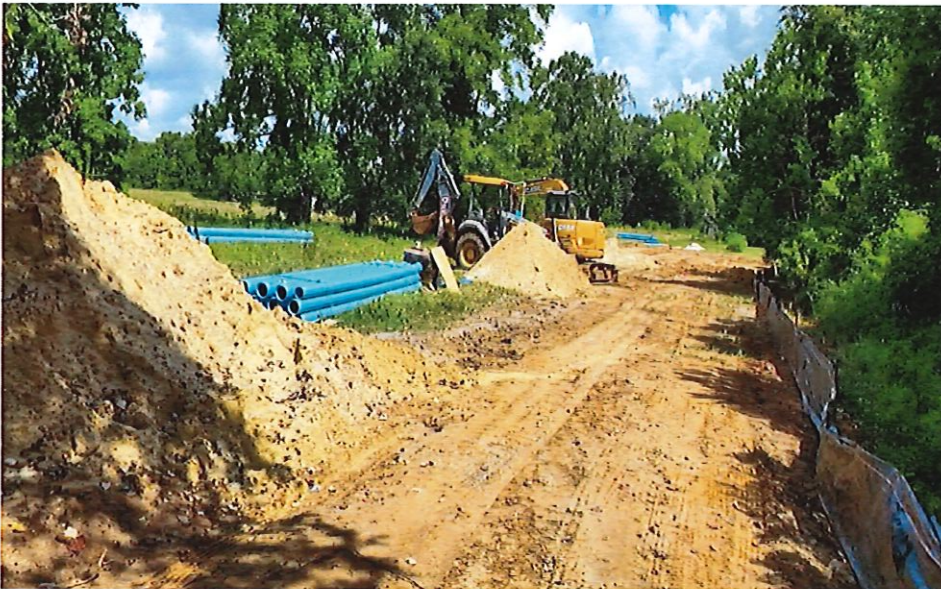
HOLLY STREET PROJECT HAS BEGUN - LOOKING DOWN BOWIE STREET ROW FROM EDGEWOOD ST.
