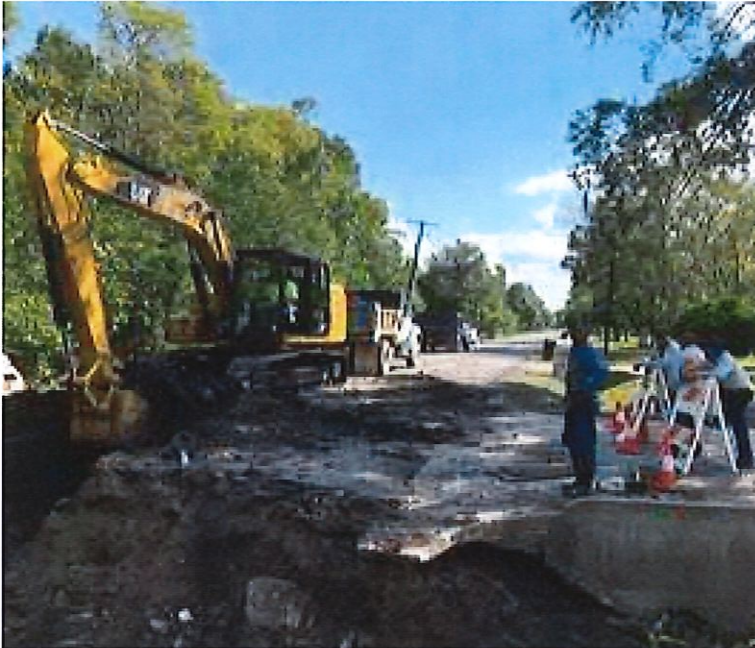
WATER / WASTEWATER DEPARTMENT EXCAVATING FOR A LARGE REPAIR
