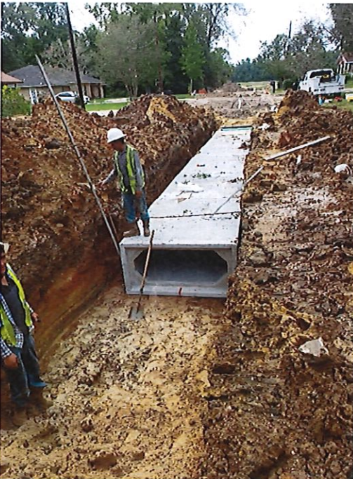
HOLLY STREET BOX CULVERT INSTALLATION
