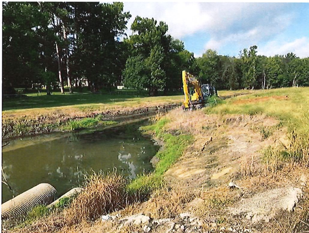
MAIN A CULVERT SEALANT WORK
