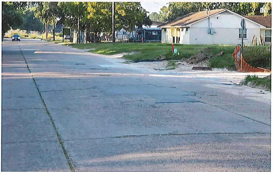
TEXAS STREET: BEAUMONT AVENUE TO NORTH OF NEWMANSTREET - SANITARY SEWER, STORM SEWER AND PAVEMENT RESTORATION
