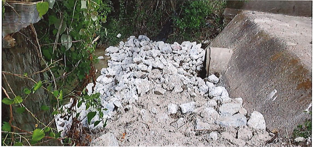
HWY 146 WATER LINE PROTECTION WORK
