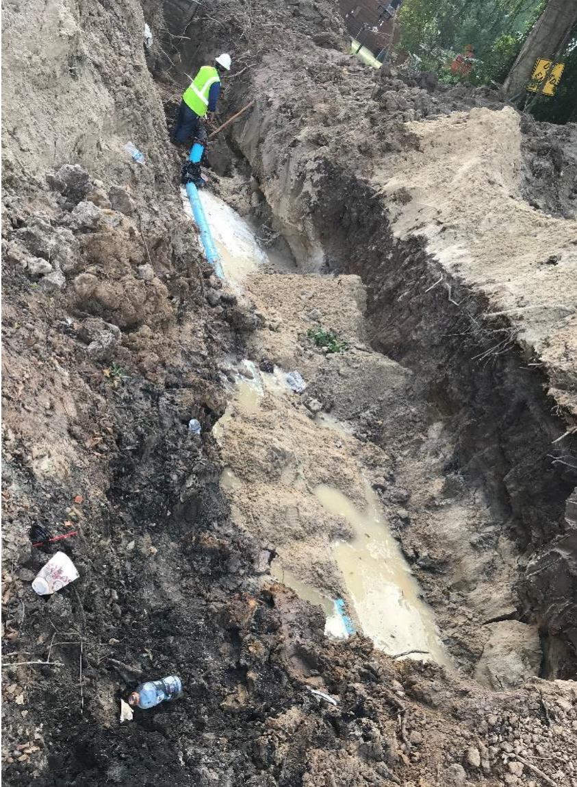
HOLLY STREET WATERLINE INSTALLATION
