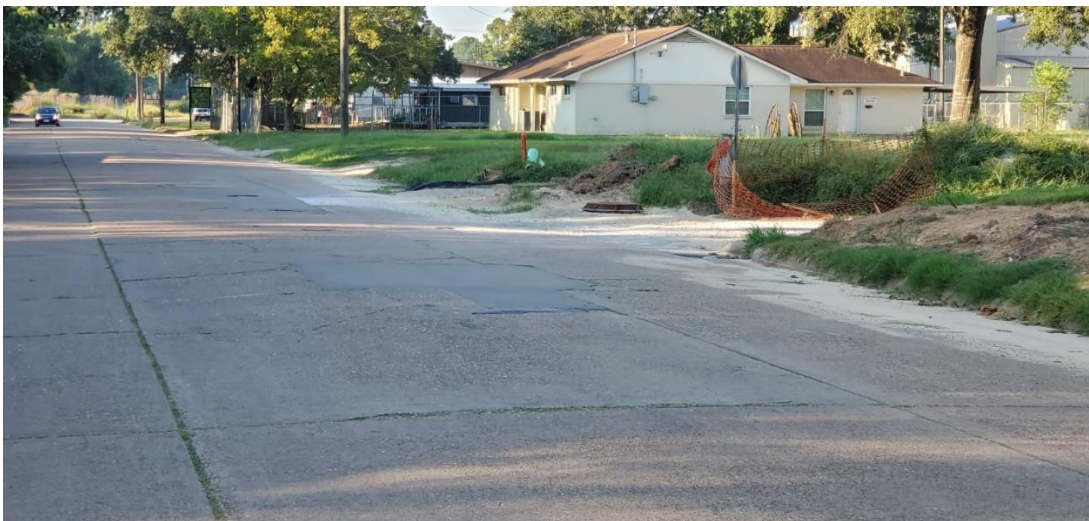
TEXAS STREET: BEAUMONT AVENUE TO NORTH OF NEWMANSTREET - SANITARY SEWER, STORM SEWER AND PAVEMENT RESTORATION
