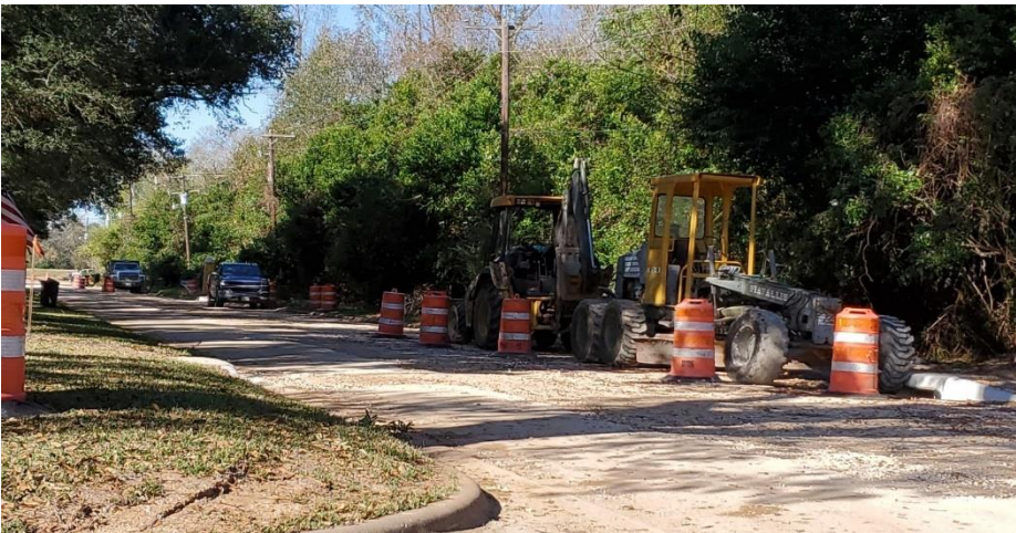
HOLLY STREET BASE PREPARATION FOR OVERLAY
