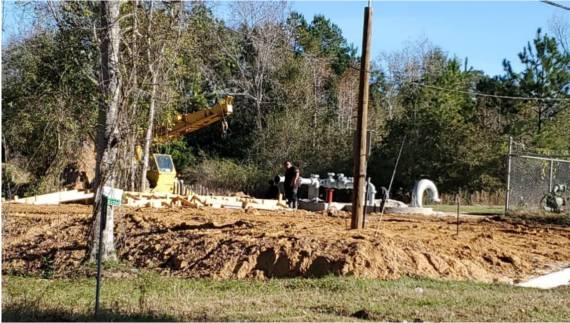
BEAUMONT STREET: BEAUMONT LIFT STATION – PROJECTED COMPLETION END OF DECEMBER
