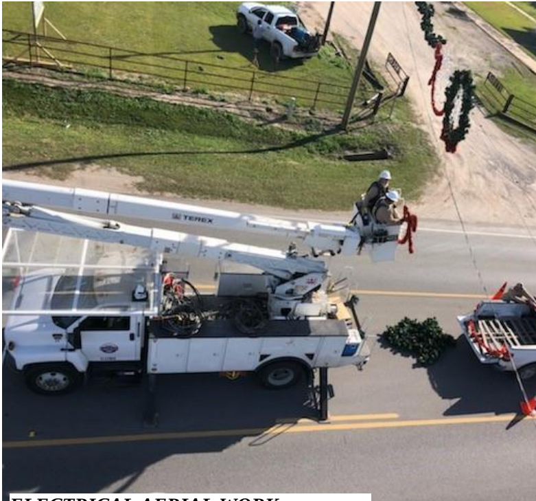
ELECTRICAL AERIAL WORK
