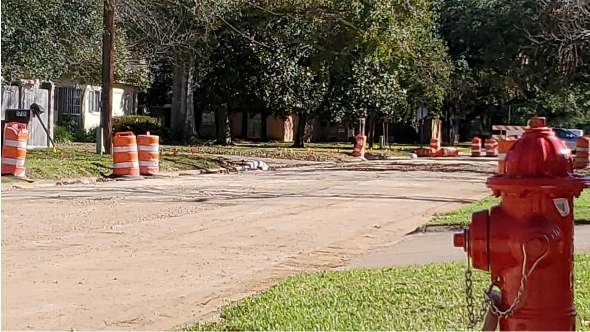
HOLLY STREET BASE PREPARATION FOR OVERLAY
