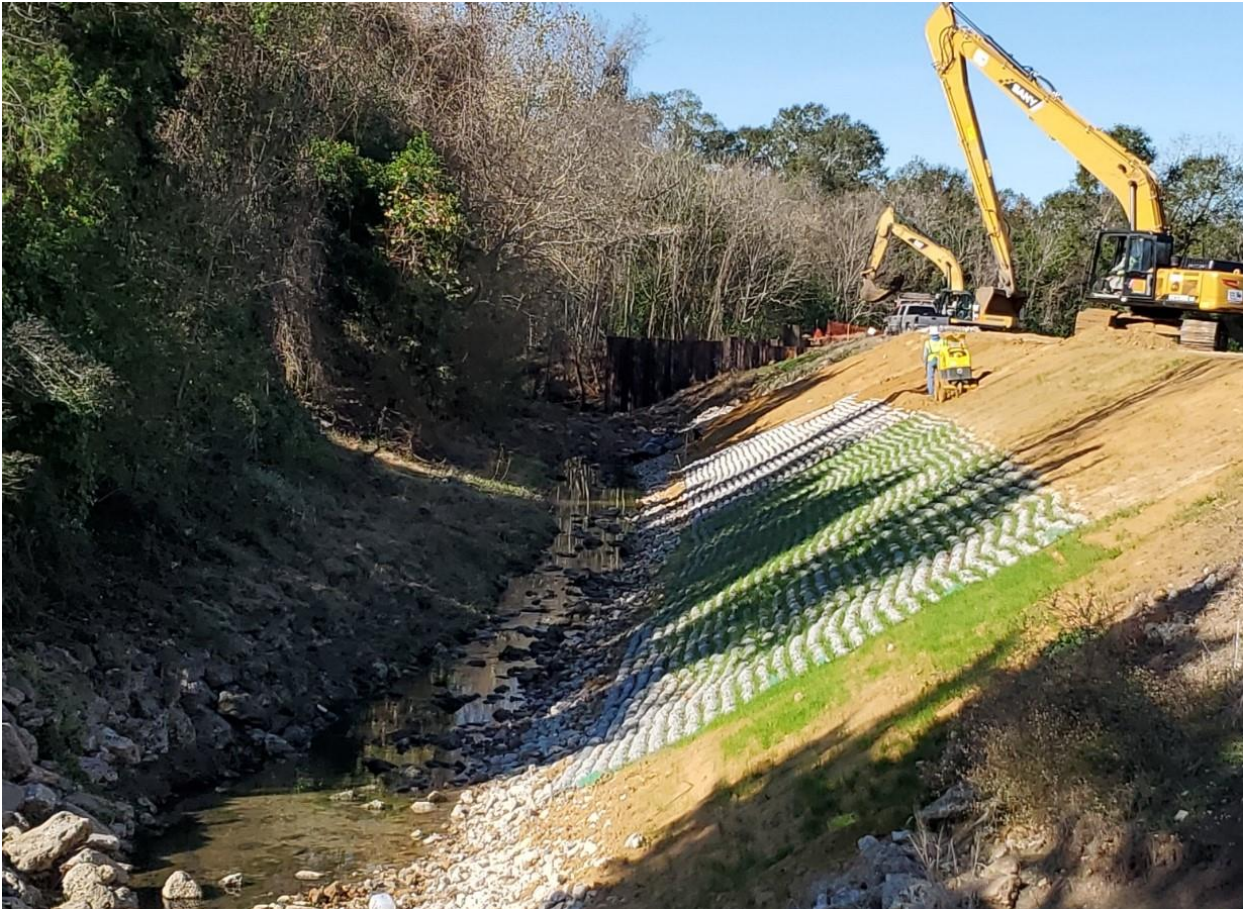
MAIN B LEVEE REPAIR
