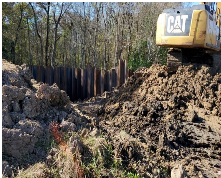
MAIN B PIPE REPAIR WORK
