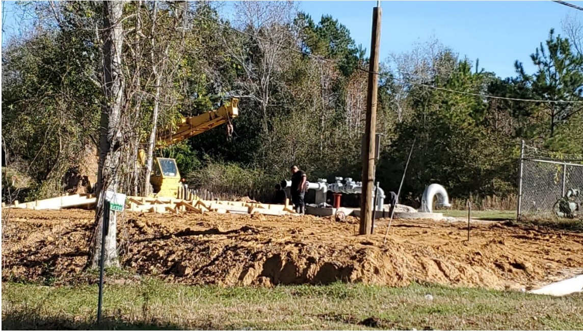
BEAUMONT STREET: BEAUMONT LIFT STATION – PROJECTED COMPLETION END OF JANUARY 2020
