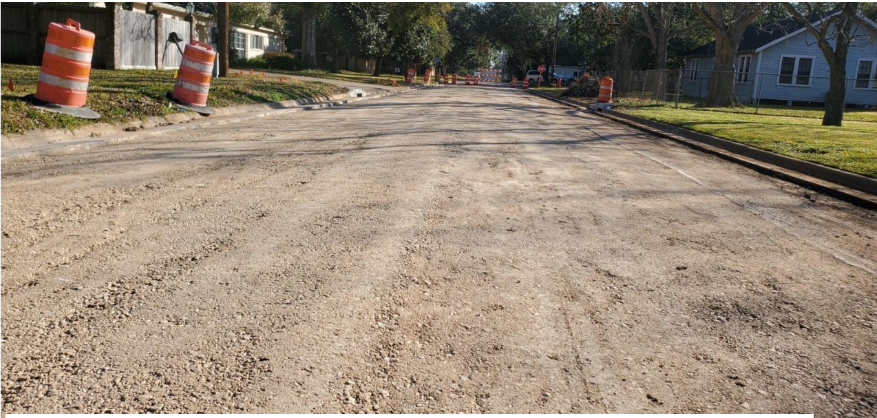
HOLLY STREET BASE PREPARATION FOR OVERLAY
