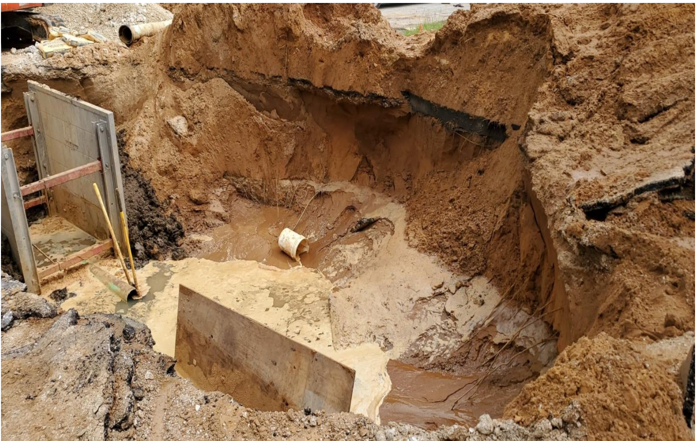
TEXAS AND HOLLY SANITARY SEWER REPAIR (Sept. 2019)
