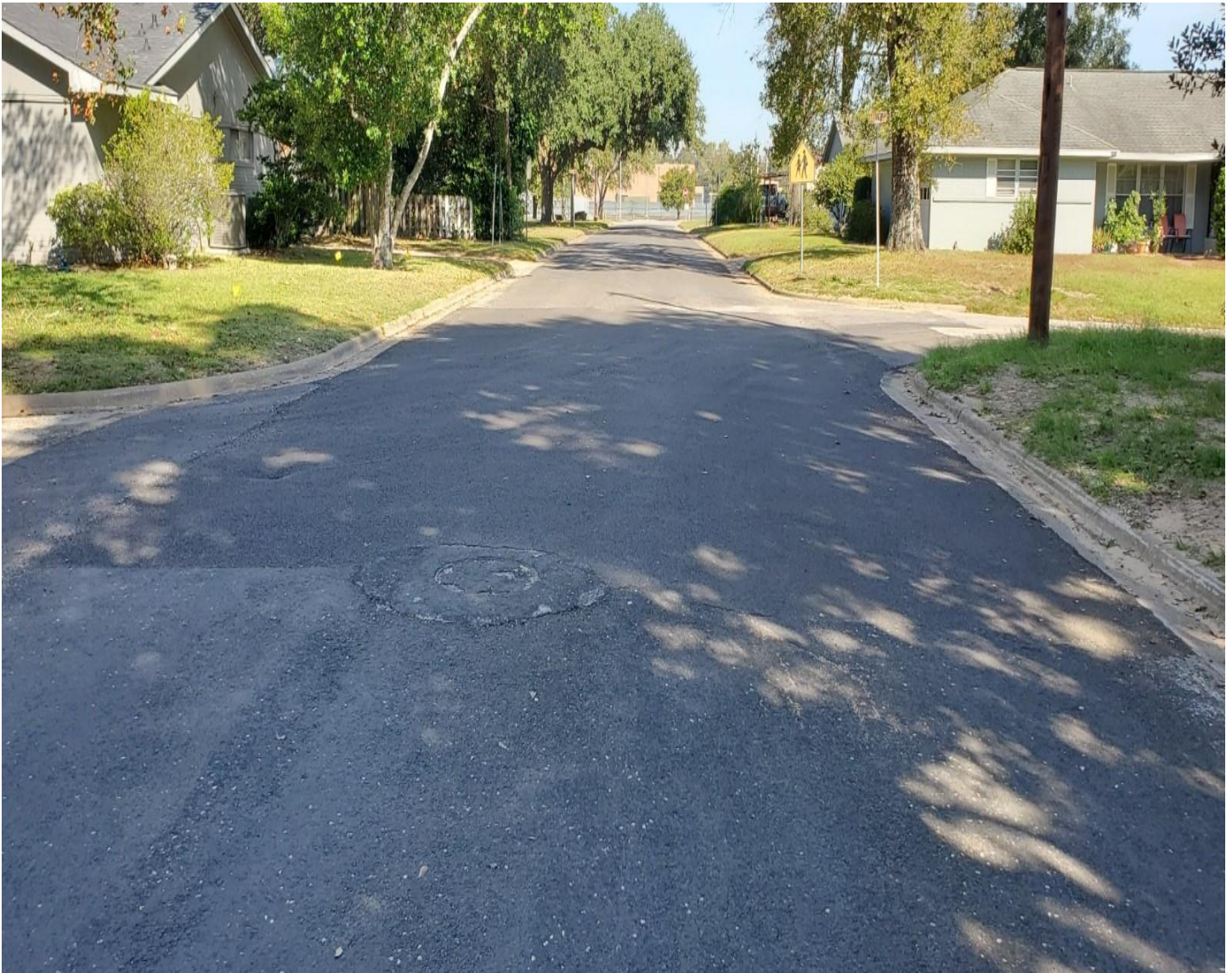
COMPLETED RESULT OF THE TEXAS AND HOLLY REPAIR PERFORMED BY THE WATER DEPARTMENT AND THE STREETS DEPARTMENT (Sept. 2019)
