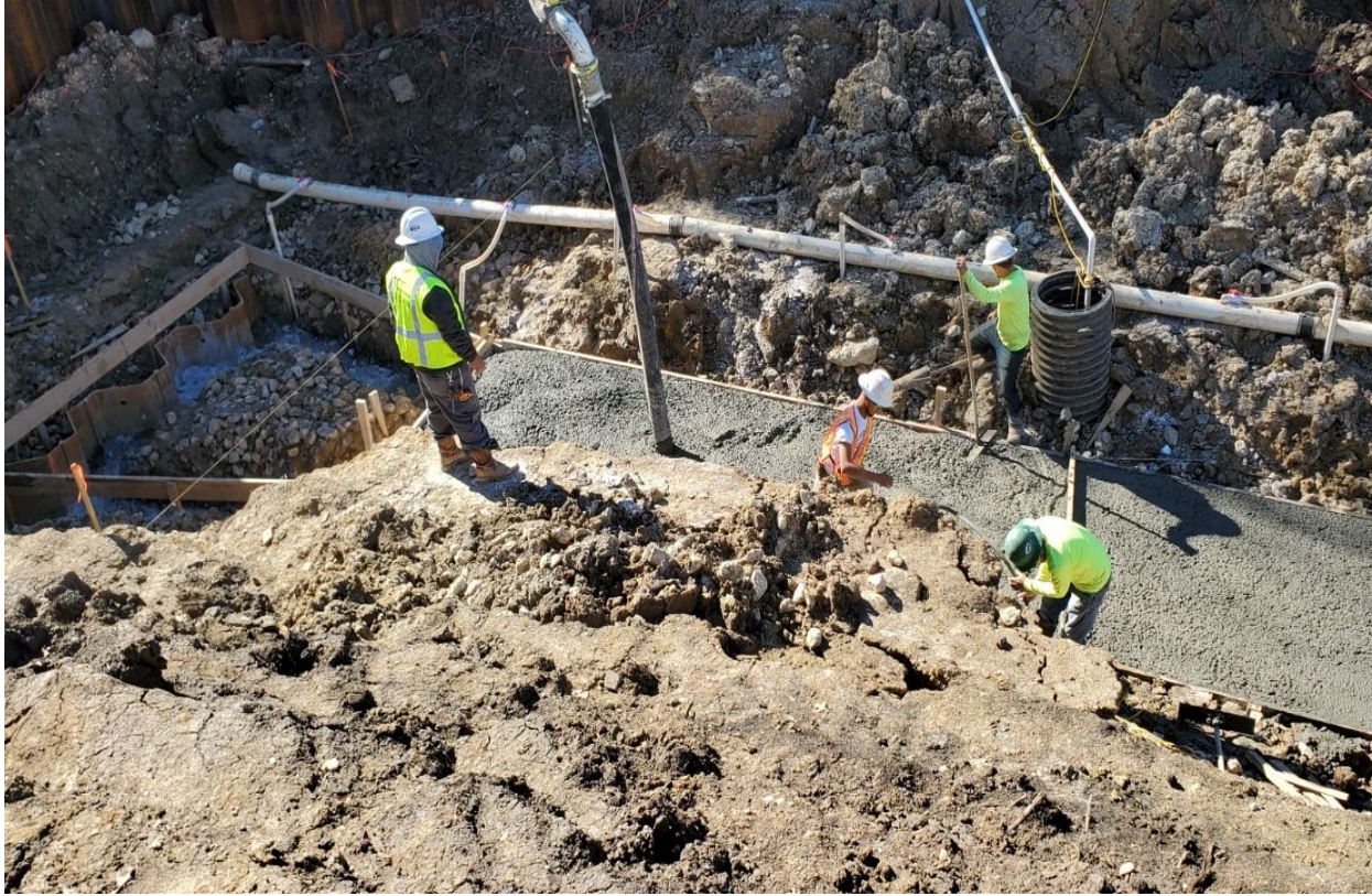
PLACING CONCRETE PIPE CRADLE FOUNDATION WITH INSTALLED WELL POINTS
