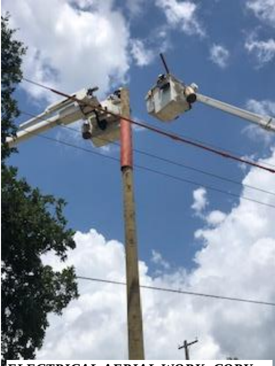
ELECTRICAL AERIAL WORK: CORY FORD AND CORY ROBINS
