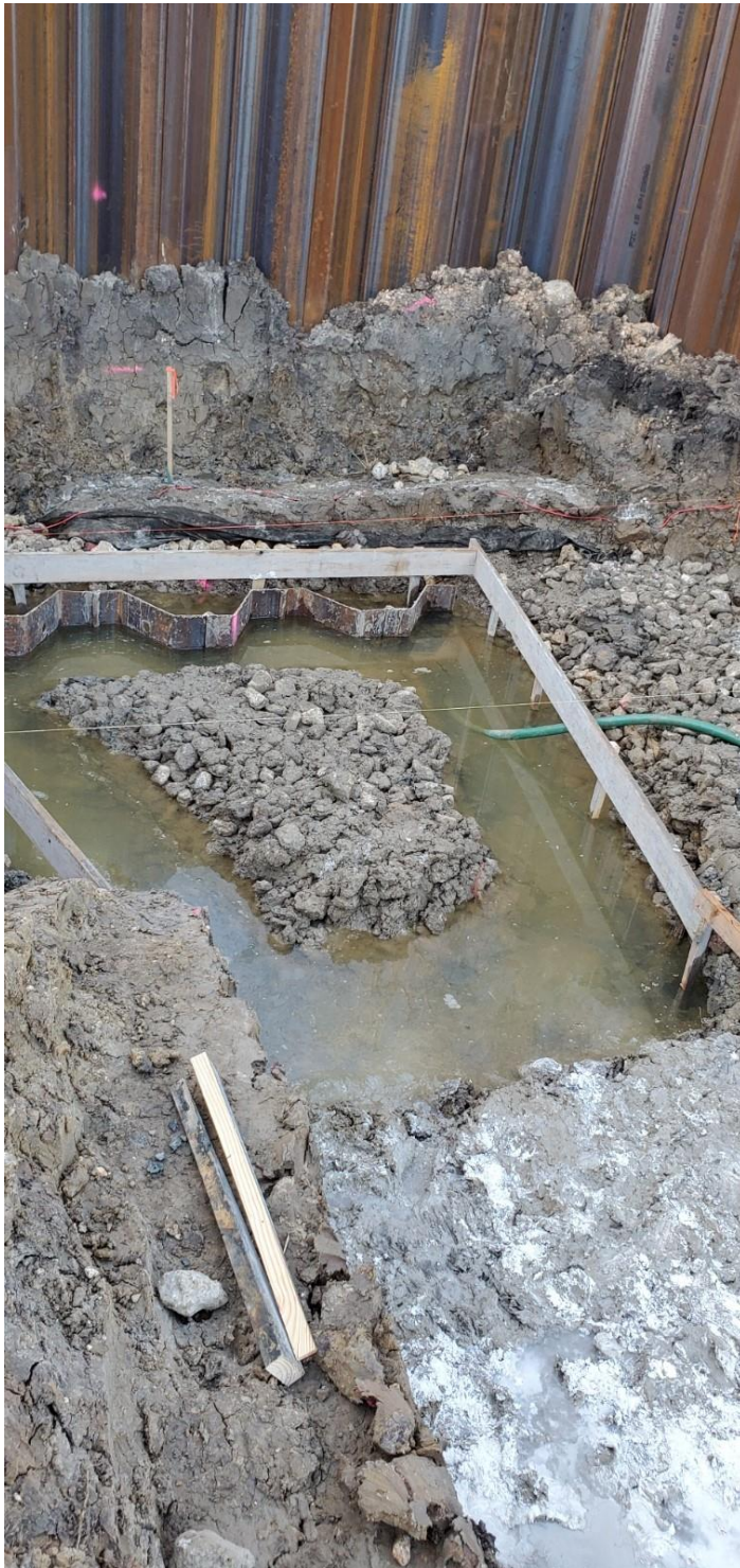
LEVEE PIPE TRENCH PRIOR TO DEWATERING
