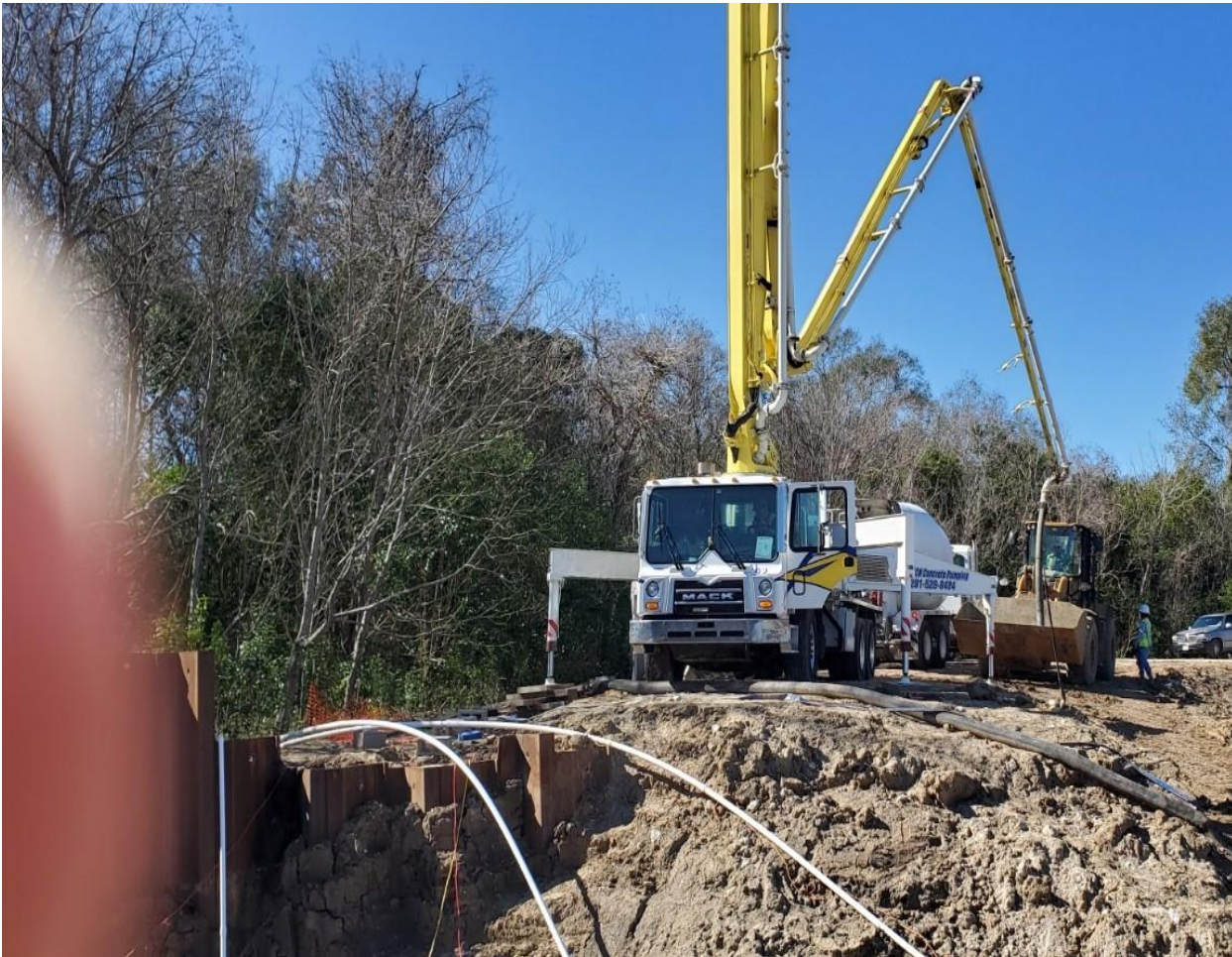
MAIN B LEVEE REPAIR
